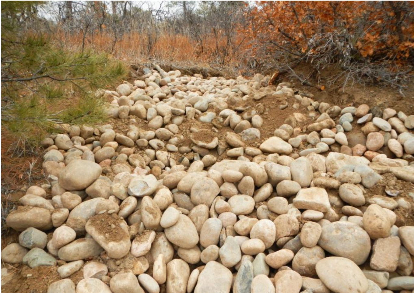
Photo 3. View of cobble placed in head-cut erosional feature.
