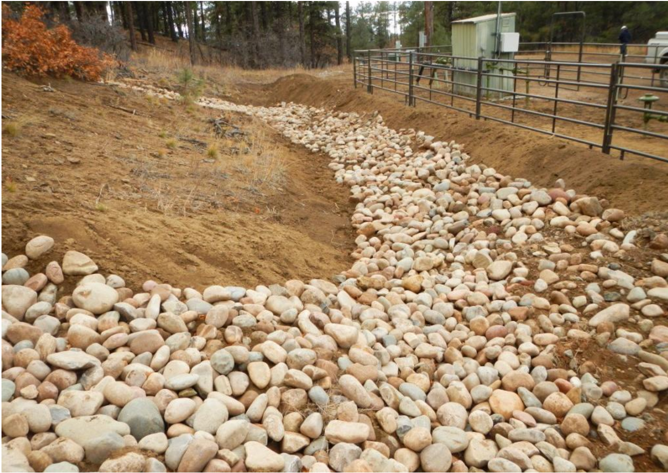
Photo 2. View of newly installed cobble and berm along eastern edge of working area.
