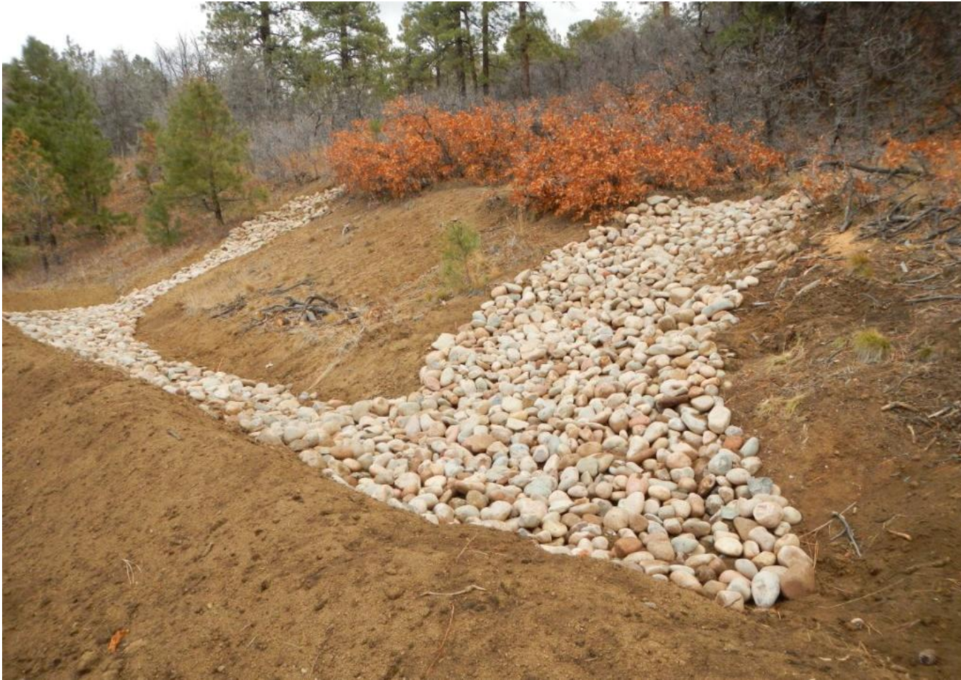
Photo 1. View of new of cobble and earthen berm placed in eastern portion of project area.
