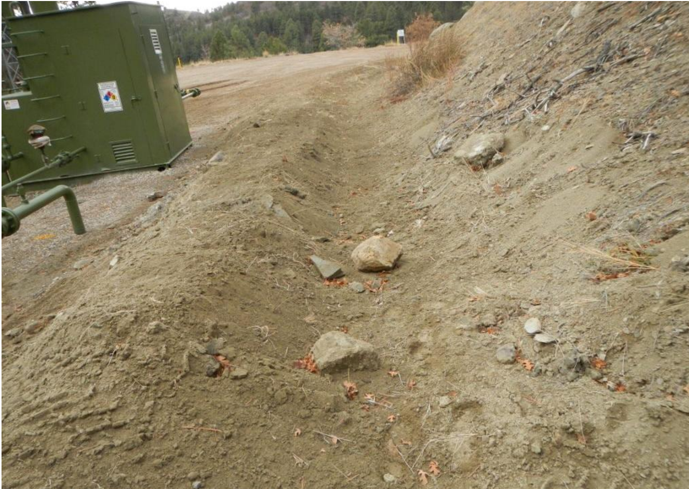
Photo 4. View of new diversion and berm in northern portion of project area facing northwestward.
