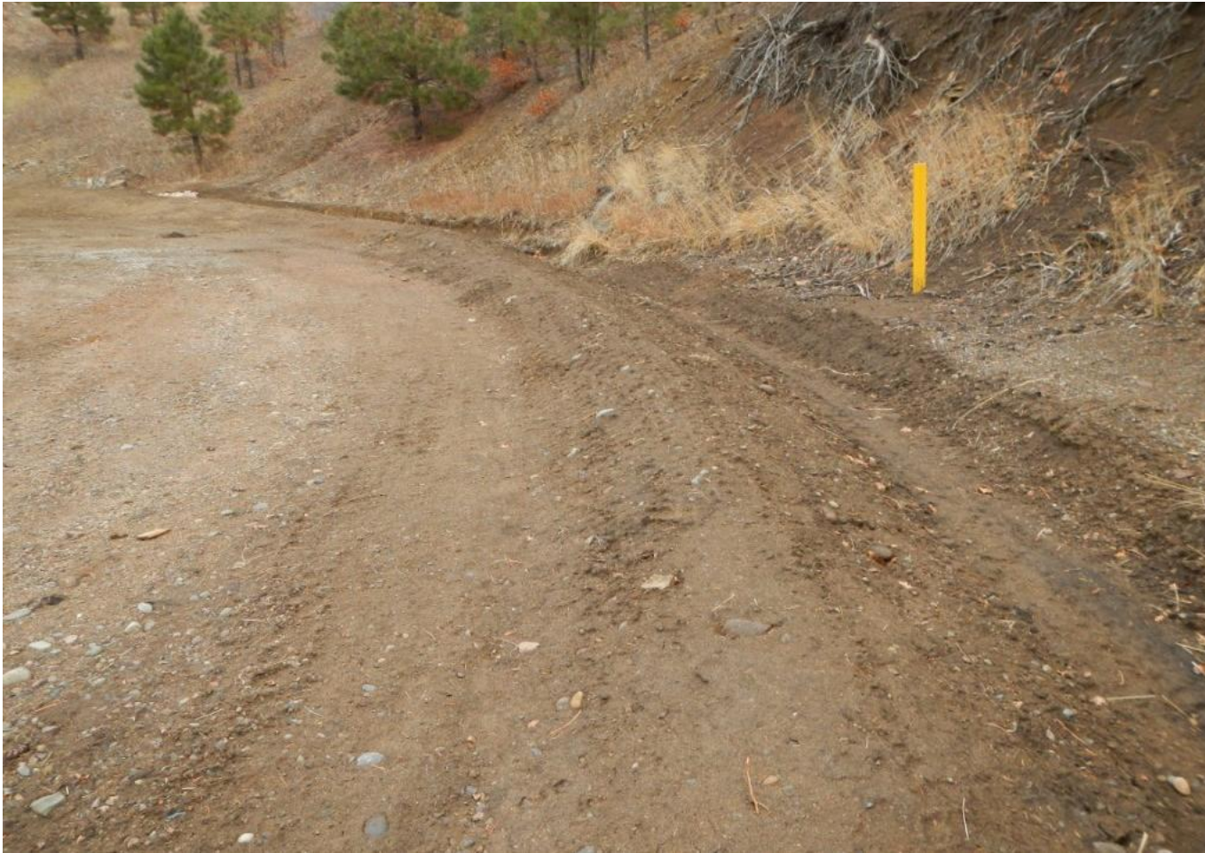
Photo 2. View of newly graded diversion on eastern edge of project area.
