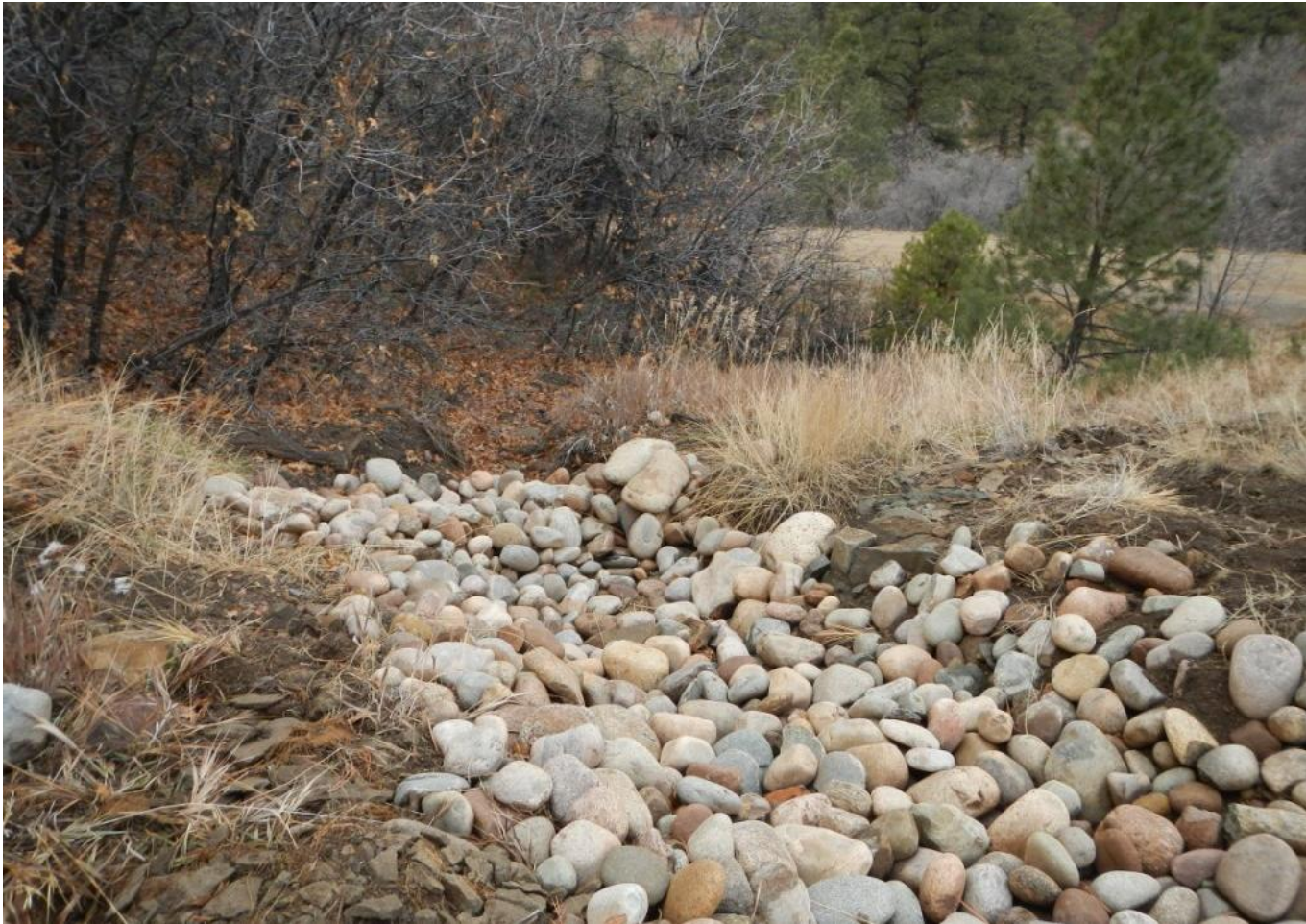
Photo 1. View of new cobble placed in gully from top of slope facing downstream.
