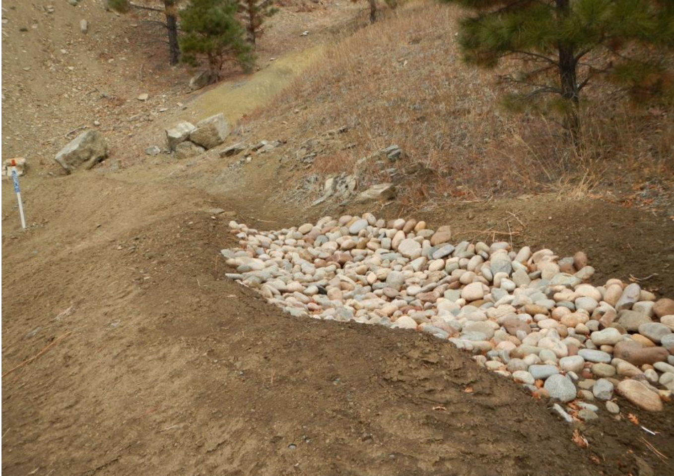
Photo 3. View of new silt trap in northeastern corner of project area.
