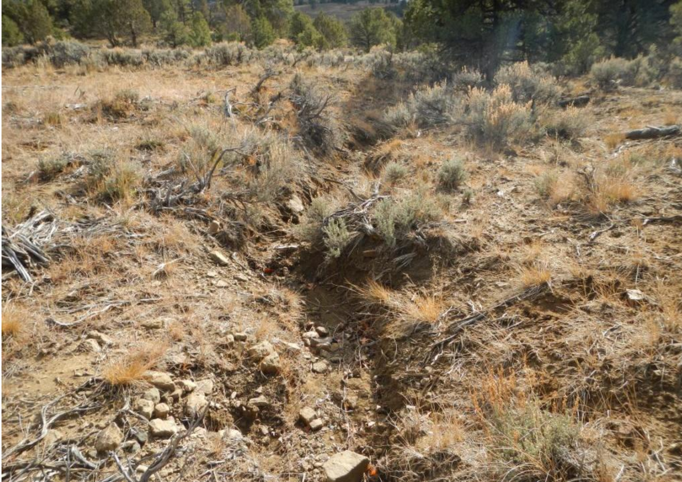
Photo 10. View of erosional channel, downstream from photos 8 and 9, facing downstream (southward). Erosion in channel appears to be accelerated by stormwater runoff from the well pad.
