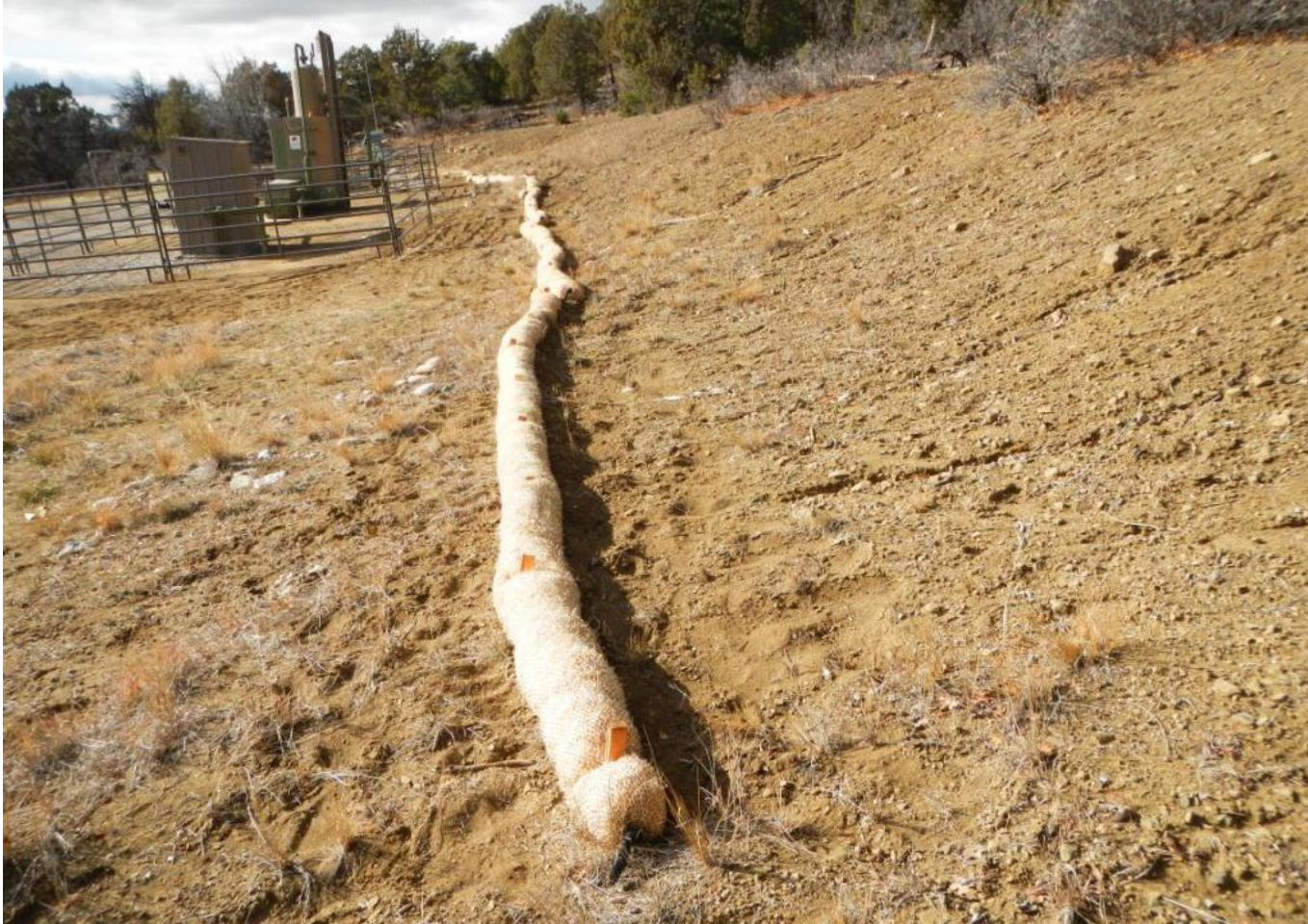
Photo 4. View of new straw wattle placed at the toe of the length of the northern cut-slope, from eastern edge facing westward.
