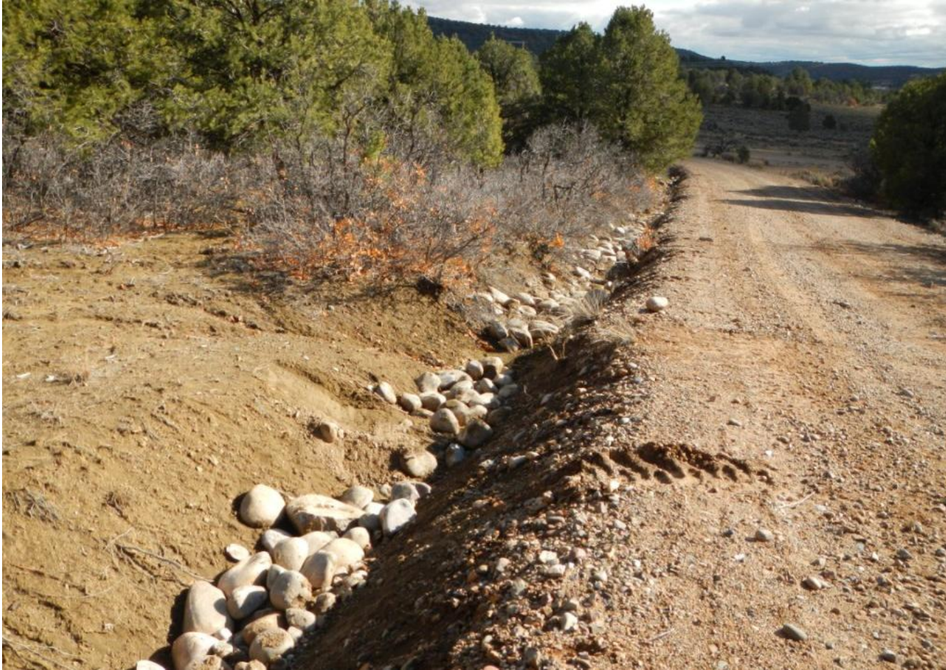
Photo 3. View downstream of diversion channel shown in photo 1 and 2, where cobble has been placed in the channel along the roadside.
