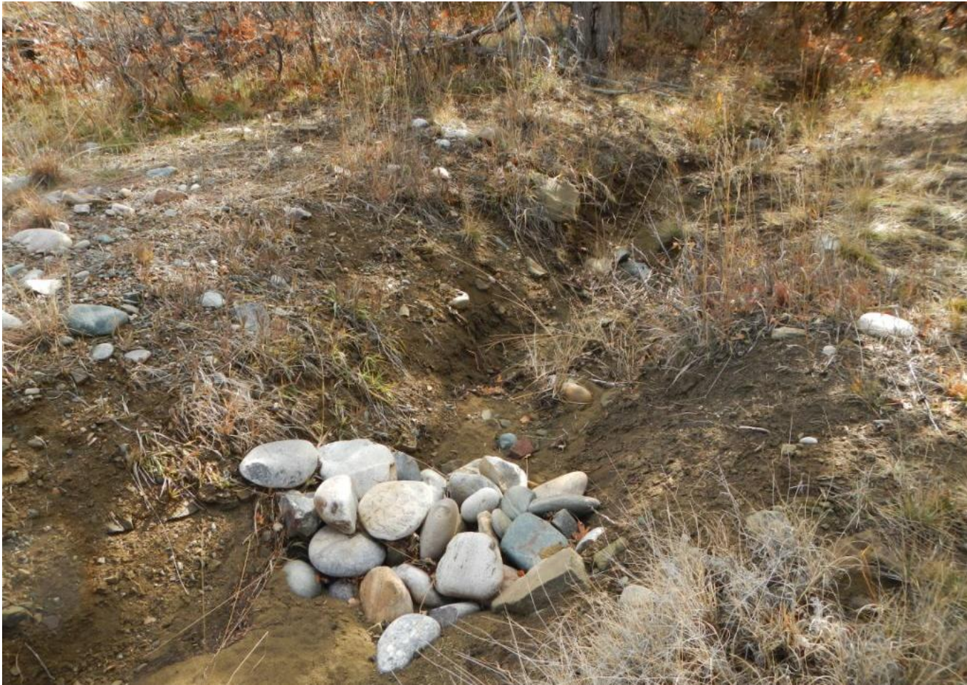
Photo 6. View of diversion channel shown in Photo 5, facing downstream (southward) where the channel exits the project area. The filter dam in the foreground was recently installed.
