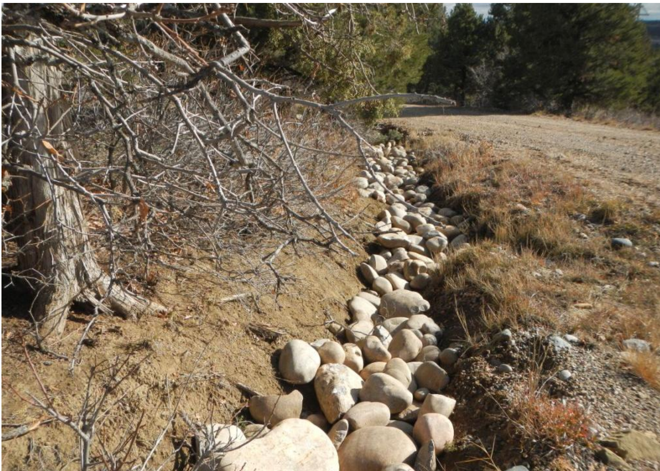
Photo 2. View of diversion channel downstream from Photo 1, where channel flows along access road (facing southeastward). Large cobble has recently been placed in channel.
