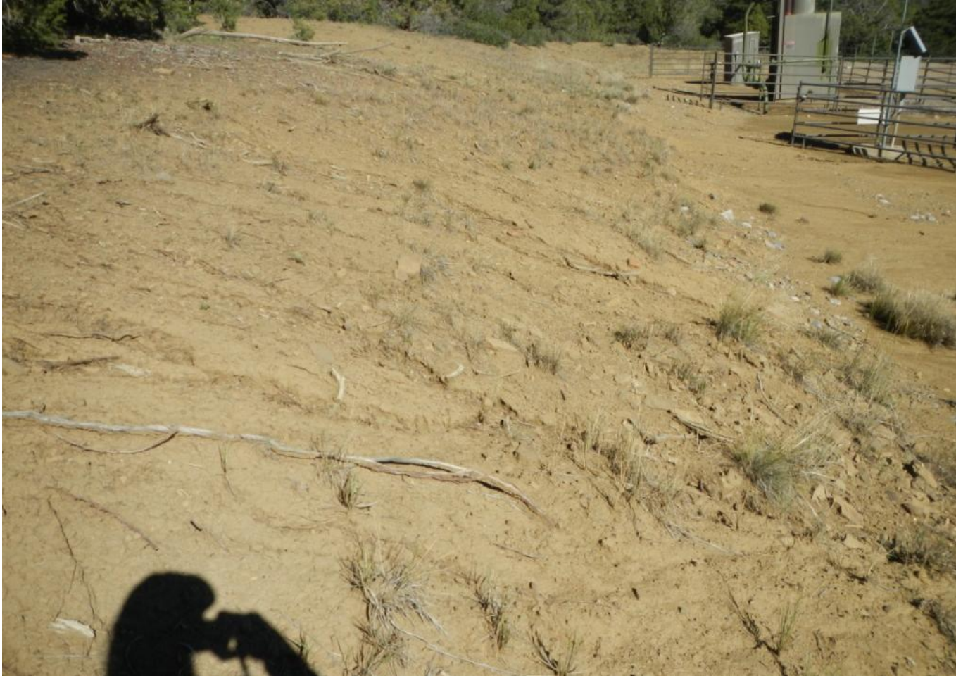
Photo 11. View of rill erosion on northern cut slope from northwestern edge facing eastward. Photo from October 2, 2014 inspection.
