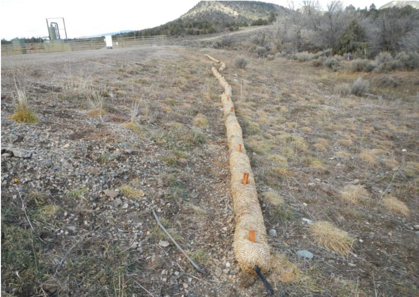
Photo 2. View of newly installed straw wattle in northern portion of the project area from northeastern corner facing westward.
