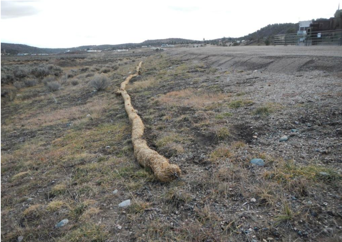
Photo 1. View of newly installed straw wattle in northern portion of the project area from northwestern corner facing eastward.
