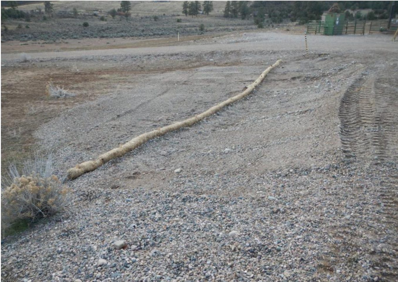
Photo 3. View of repaired gullies, new gravel, and straw wattle in eastern portion of project area.
