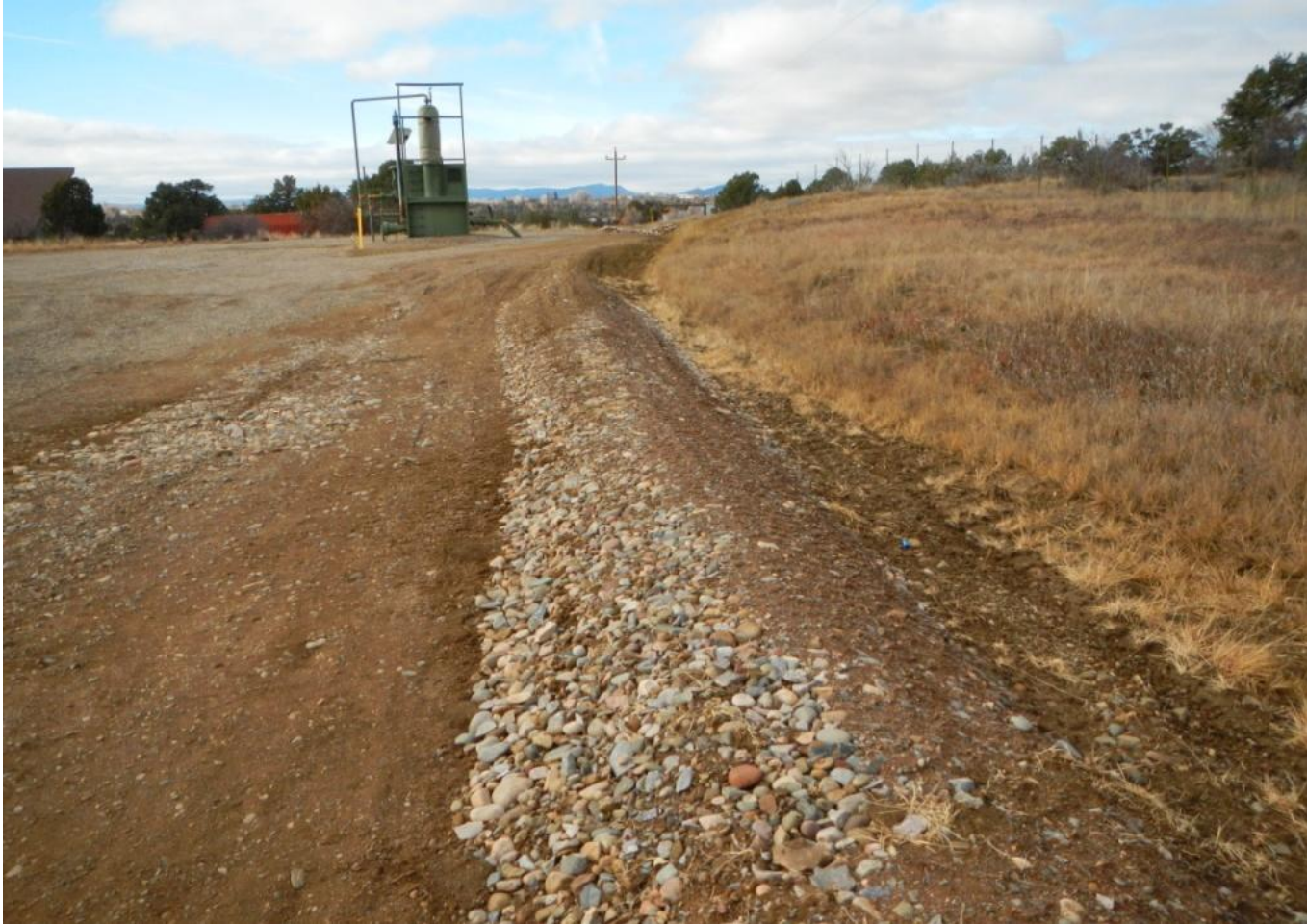
Photo 5. Newly installed berm to divert stormwater flows on the western edge of the well pad.
