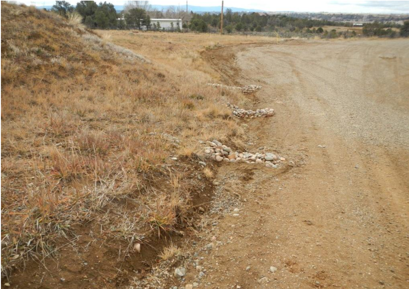
Photo 1. View of newly installed rock check dams on eastern side of access road.
