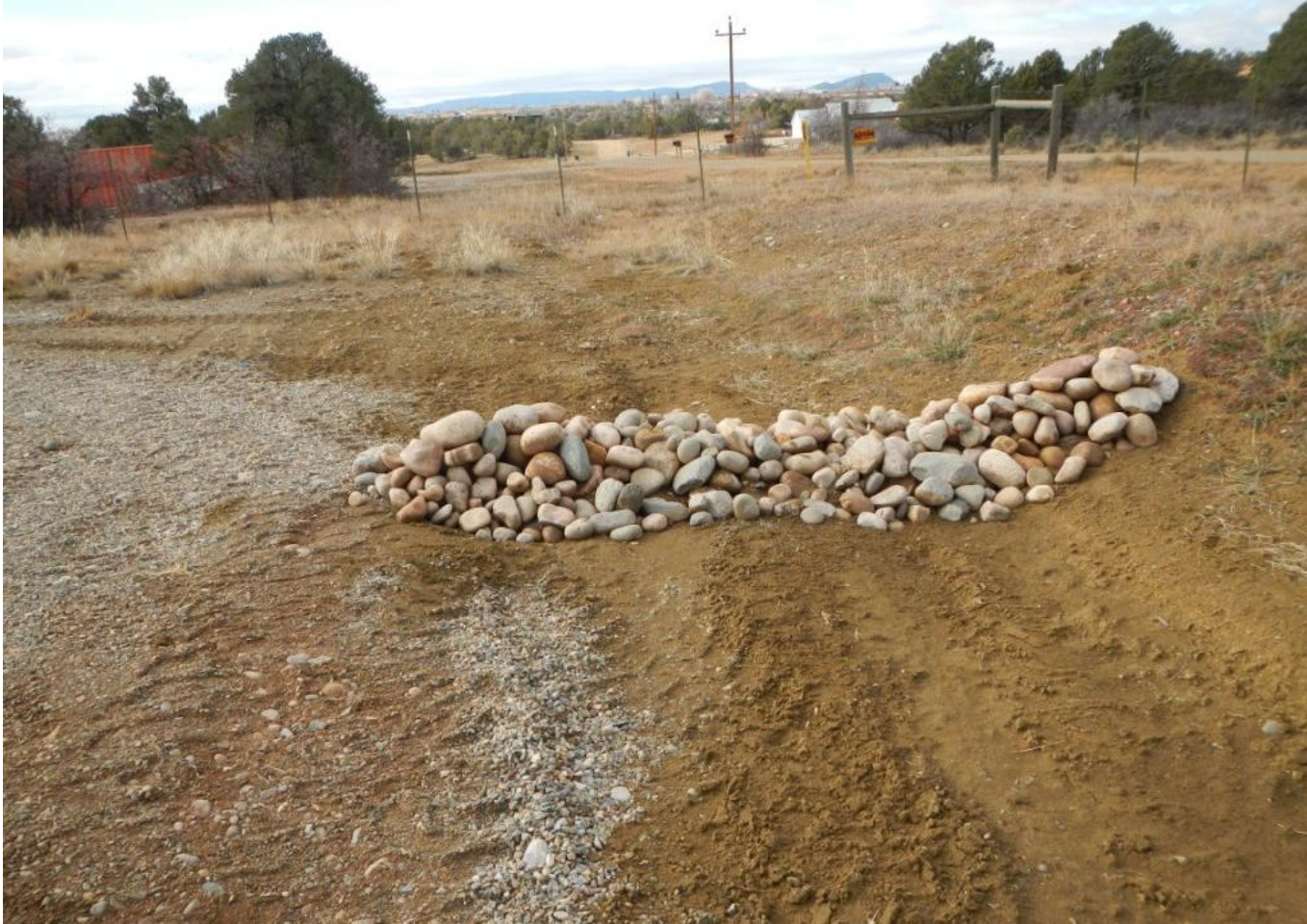
Photo 5. View of cobble check dam in southwestern corner of working area where diverted stormwater flows exit the project area.
