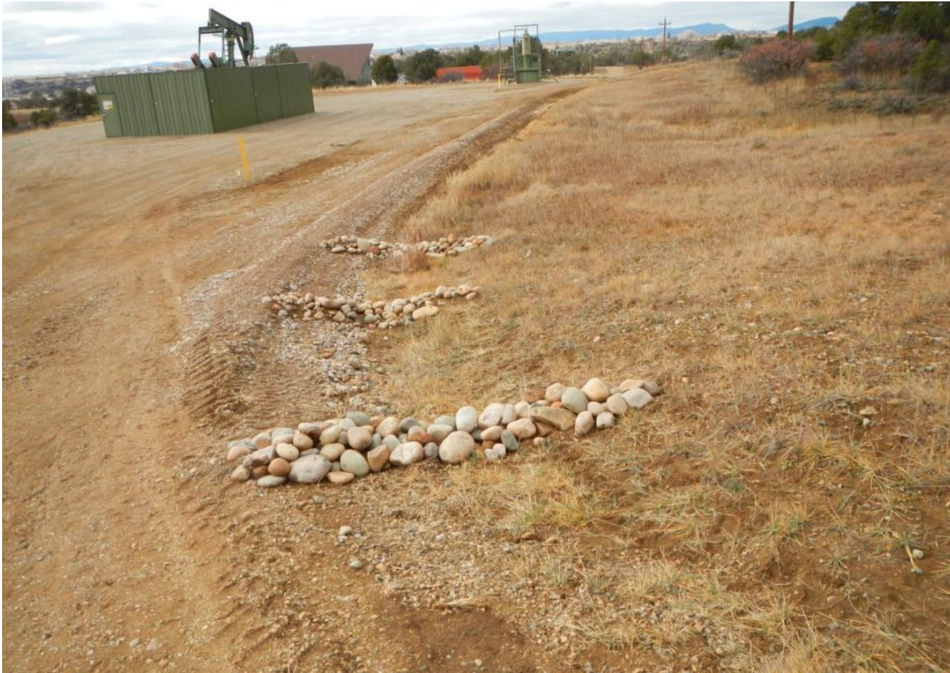
Photo 3. Newly installed rock check dams along the western edge of the access road.
