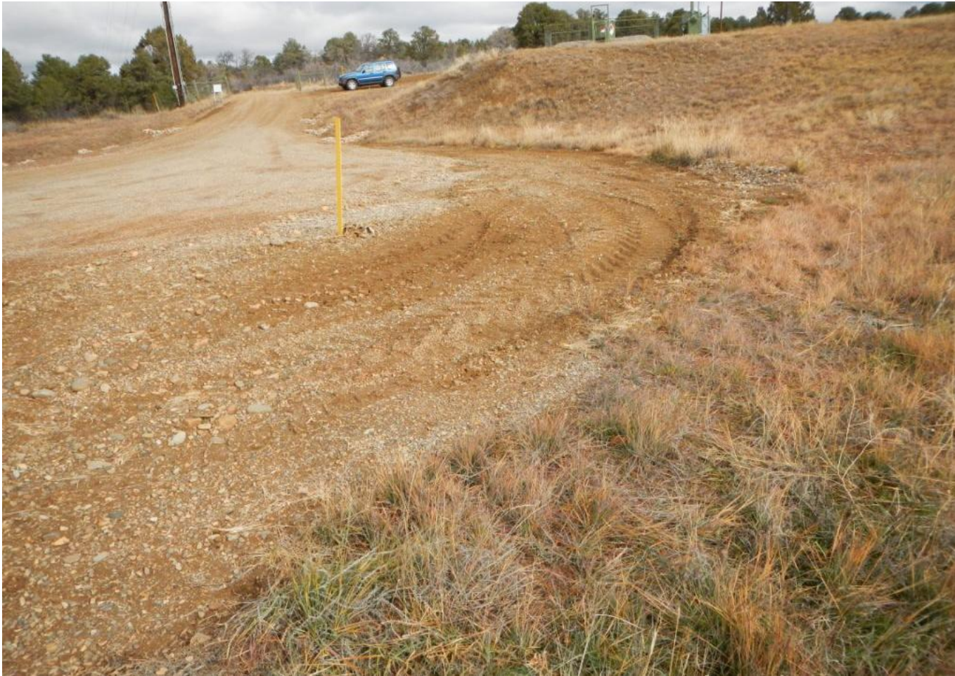
Photo 2. View of northeastern edge of working area downstream from access road that appears to have been recently bladed to divert stormwater flows to the eastern interim reclamation area.
