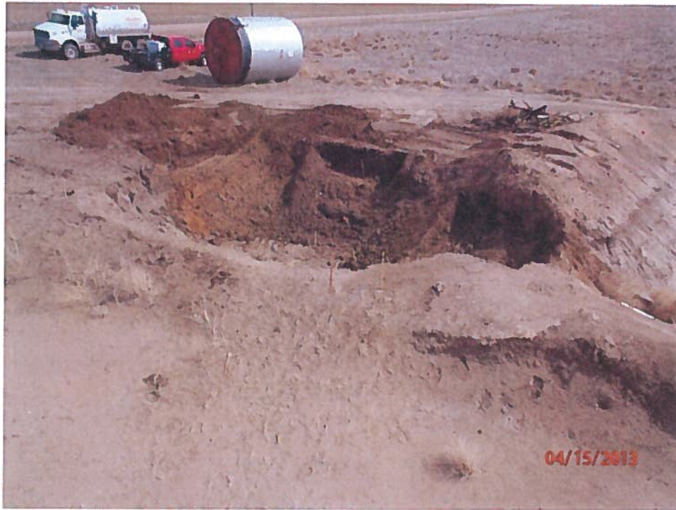
Figure 7; Former skim pit at end of second round of excavation.
