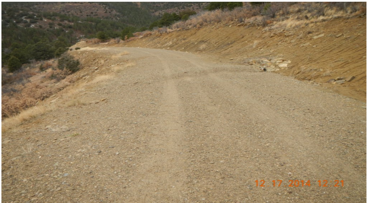
photo 4: Gravel remains along the access road and the road has not been recontoured.
