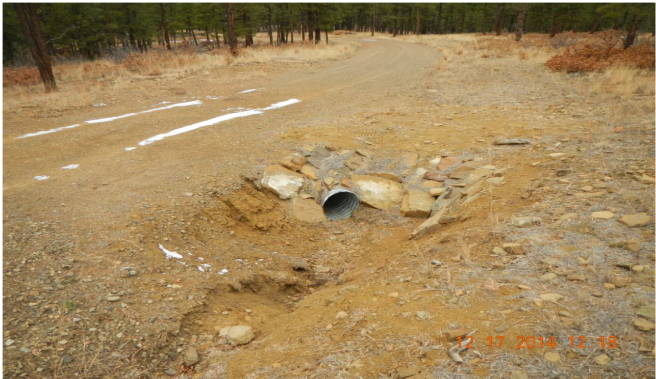
photo 2: Gravel and culverts have not been removed and the road has not been reclaimed.
