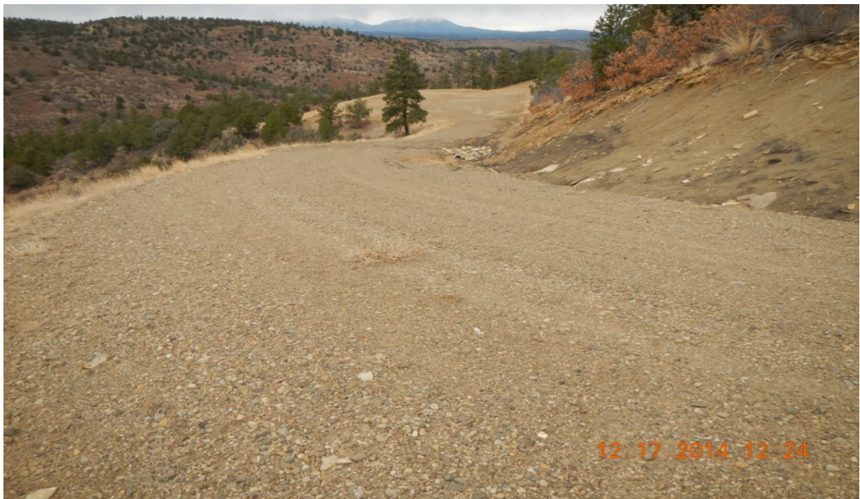
photo 6: Facing north from the access road towards the location.
