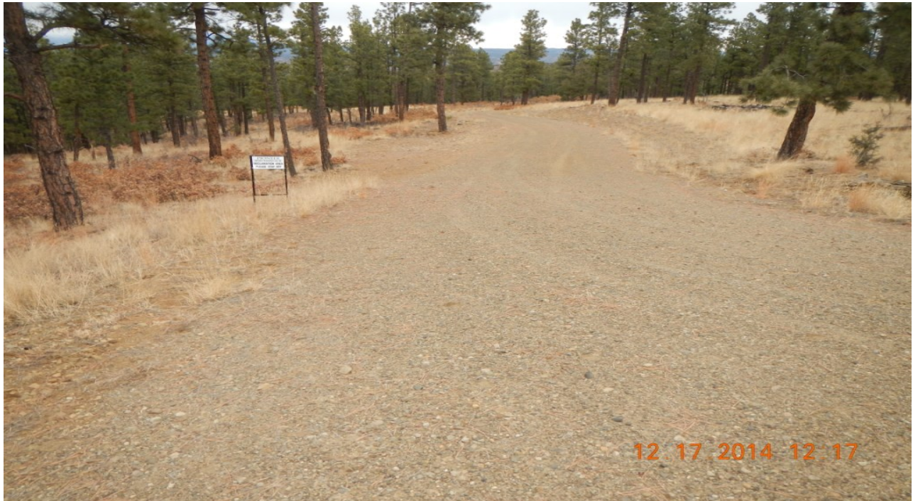
photo 1: Access road north to the location off of the main road.
