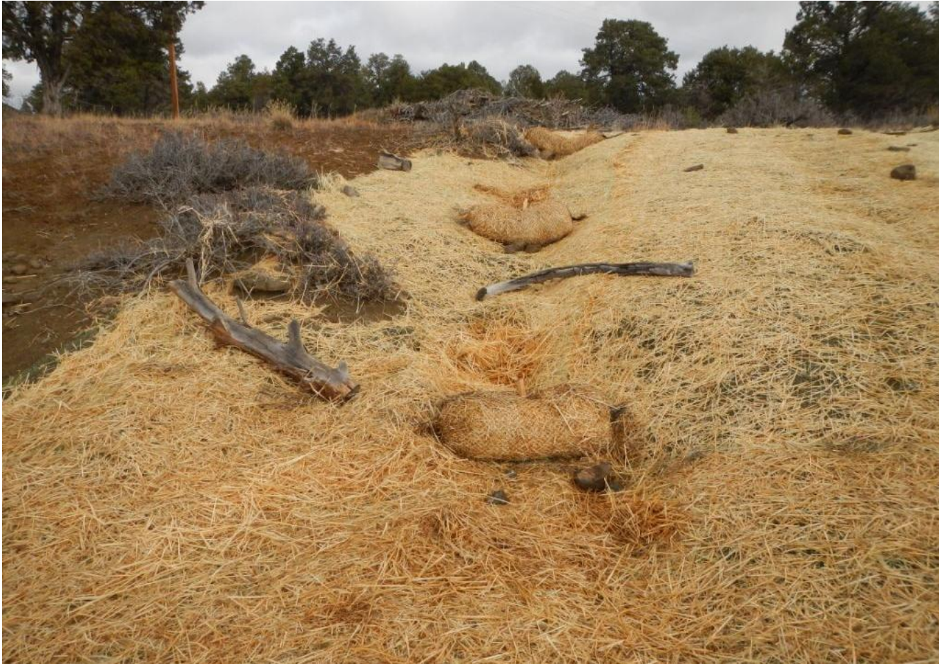
Photo 4. View of straw logs place in erosional channel.
