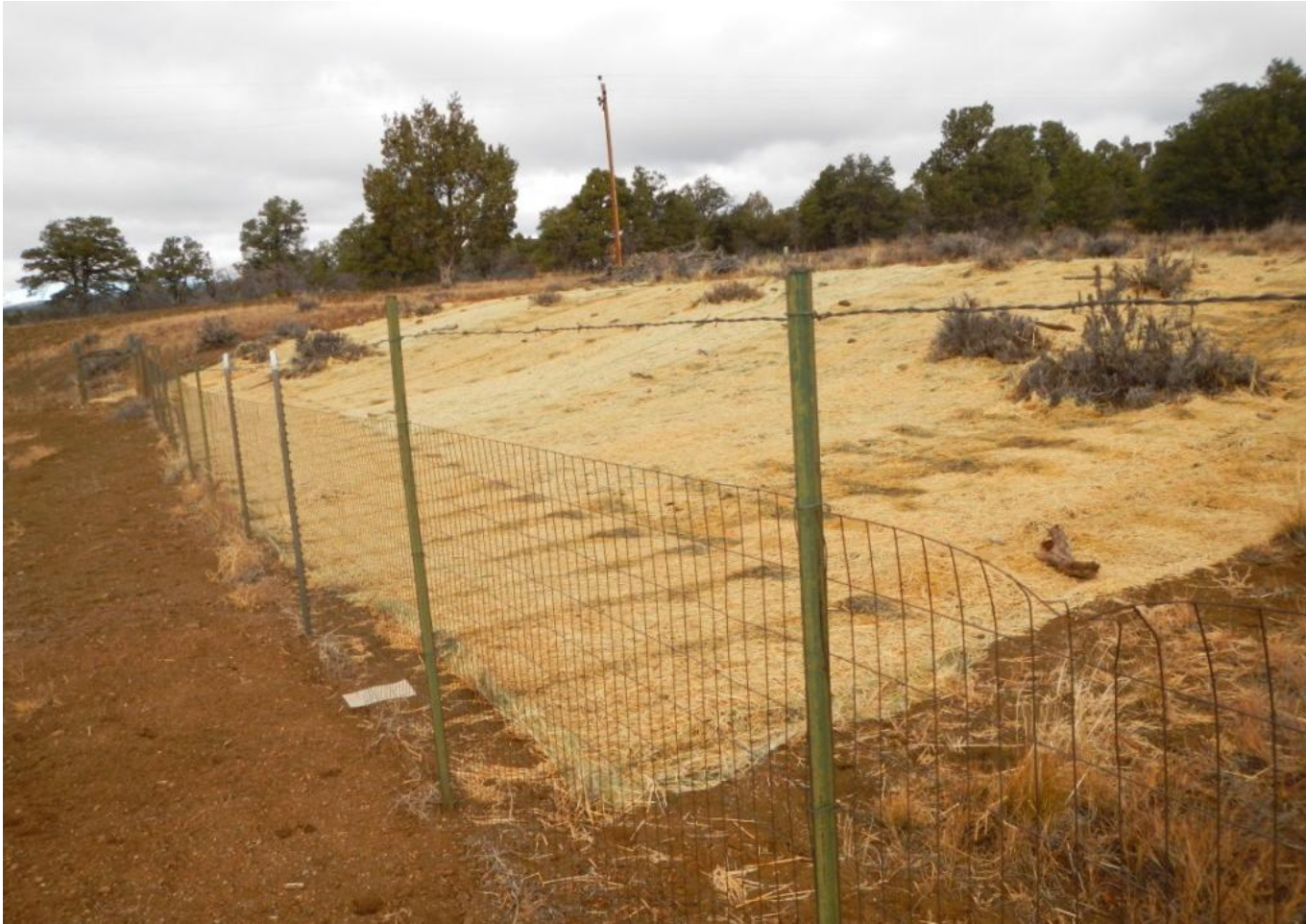
Photo 3. View of straw blanket placed on cut slope for stormwater control.
