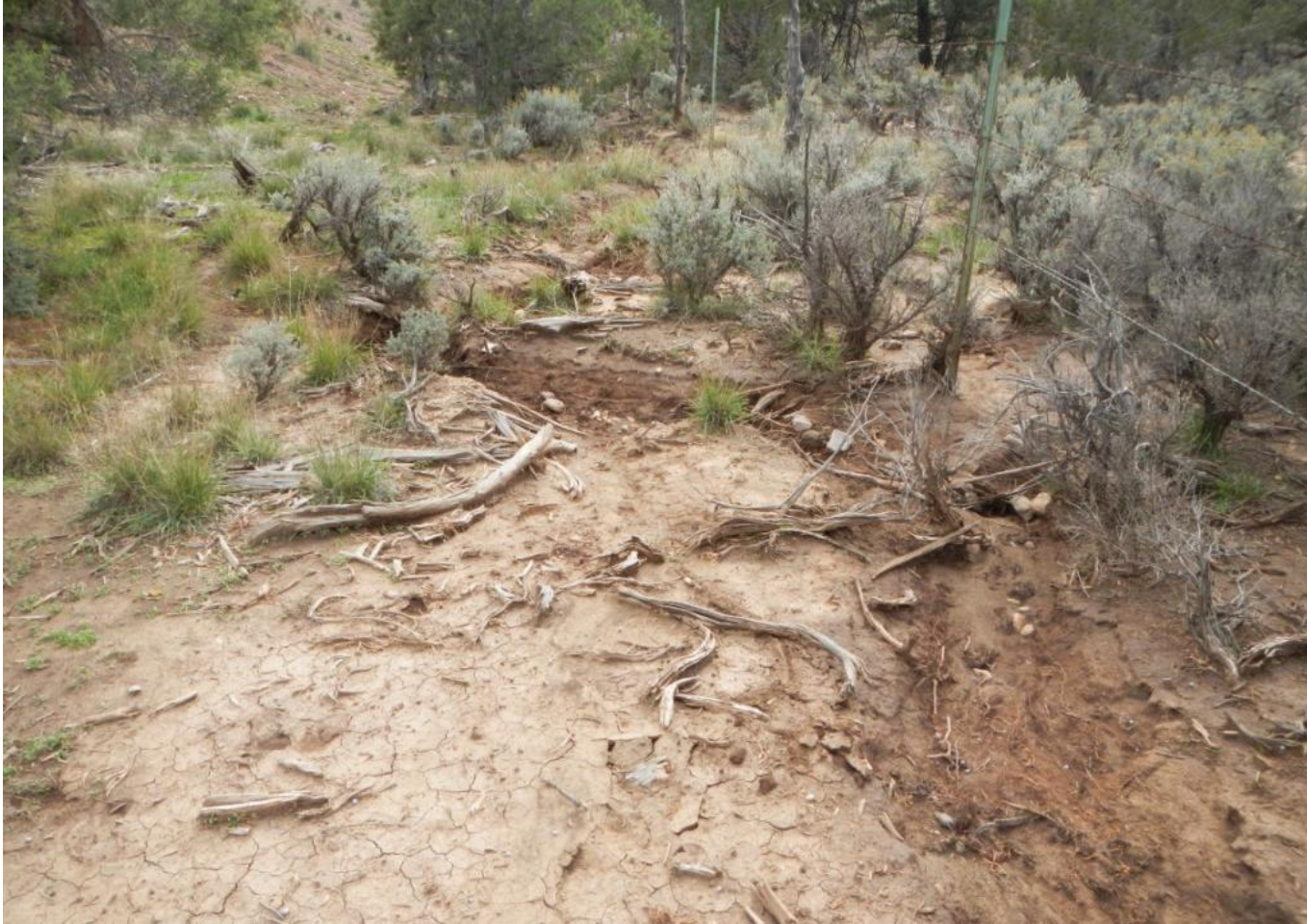
Photo 6. View of stormwater erosion outside of project area from concentrated flows not properly de-energized exiting the culvert at the well pad entrance.
