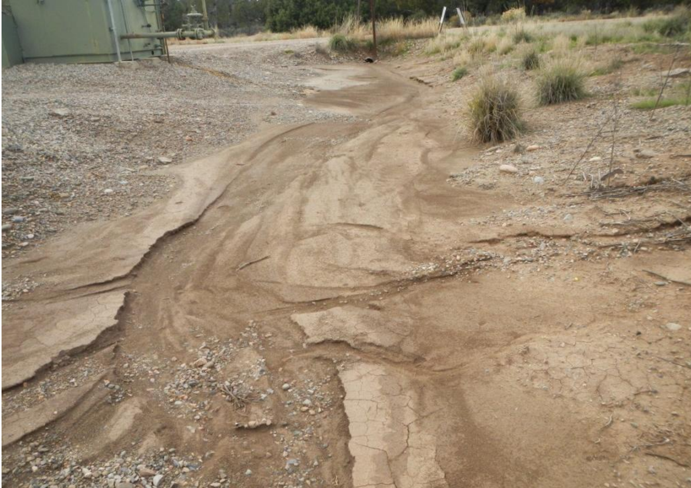
Photo 5. View of large amounts of sediment in stormwater diversion channel in northern portion of project area. Culvert in background is filling with sediment.
