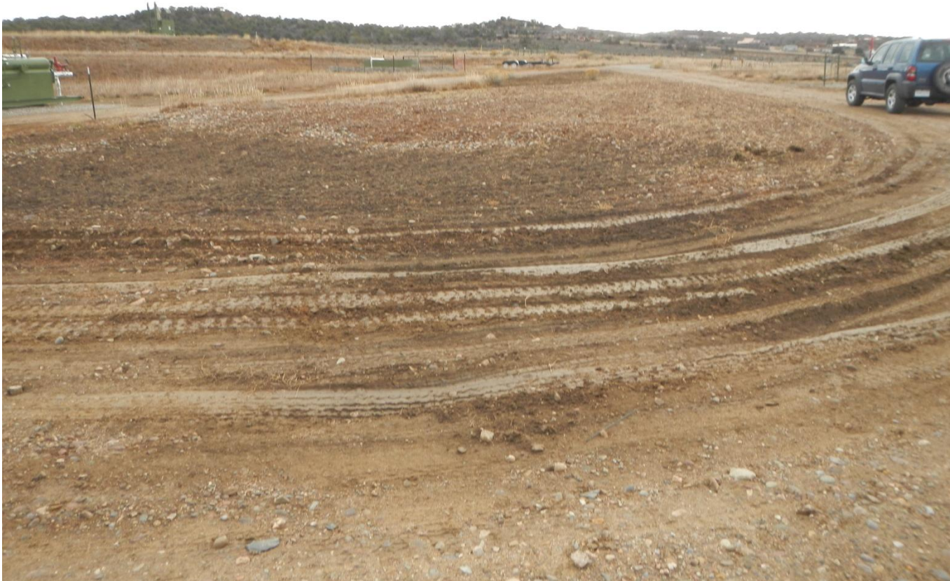
Photo 1. View of newly reclaimed area in center of well pad “teardrop” from northern portion of well pad facing southward.
