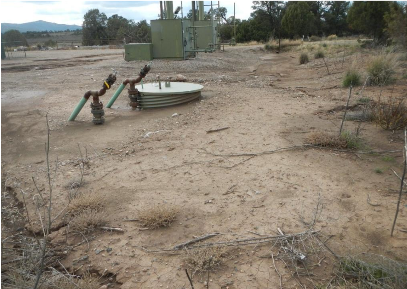
Photo 8. View of sediment run-on and erosion onto well pad in northern portion of project area.
