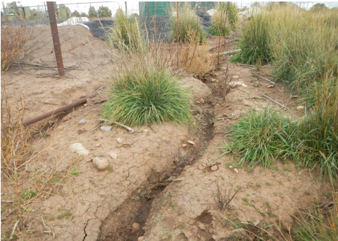
Photo 6. View of erosion at edge of old pit and exposed pipe in western portion of project area.
