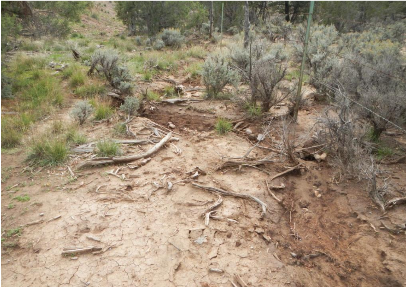
Photo 10. View of stormwater erosion outside of project area from concentrated flows not properly de-energized exiting the culvert at the well pad entrance.
