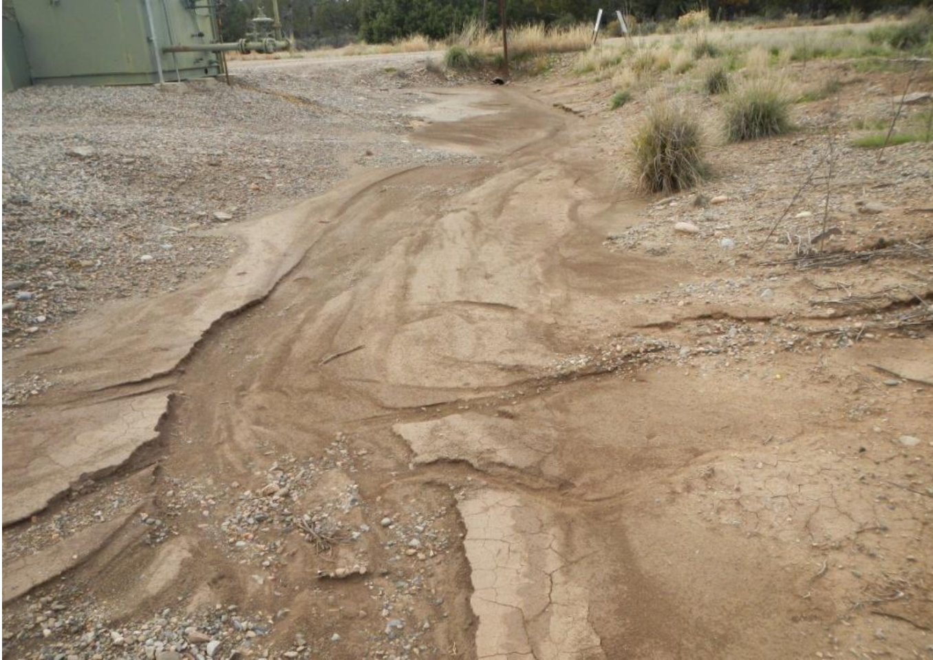
Photo 9. View of large amounts of sediment in stormwater diversion channel in northern portion of project area. Culvert in background is filling with sediment.
