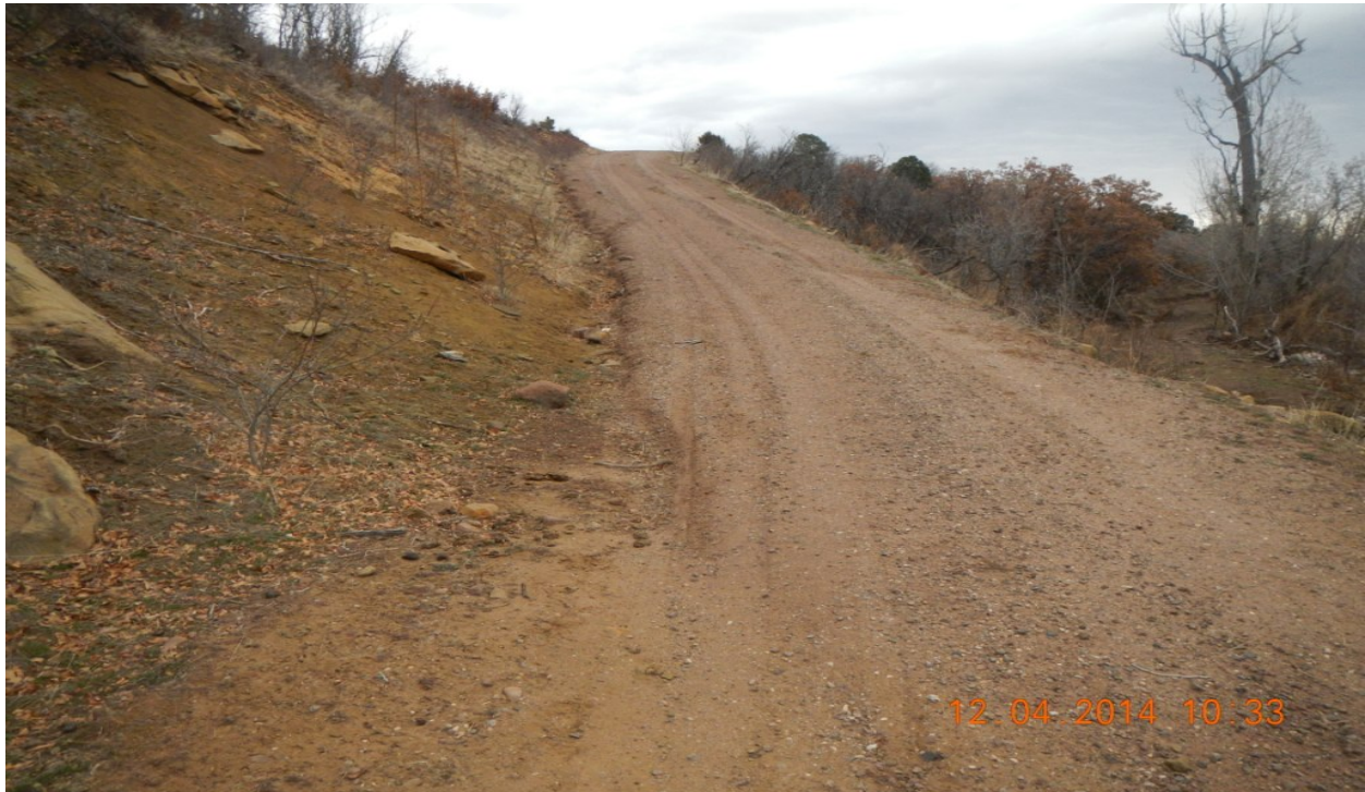
photo 6: Erosion is occurring off the slope and down the access road.
