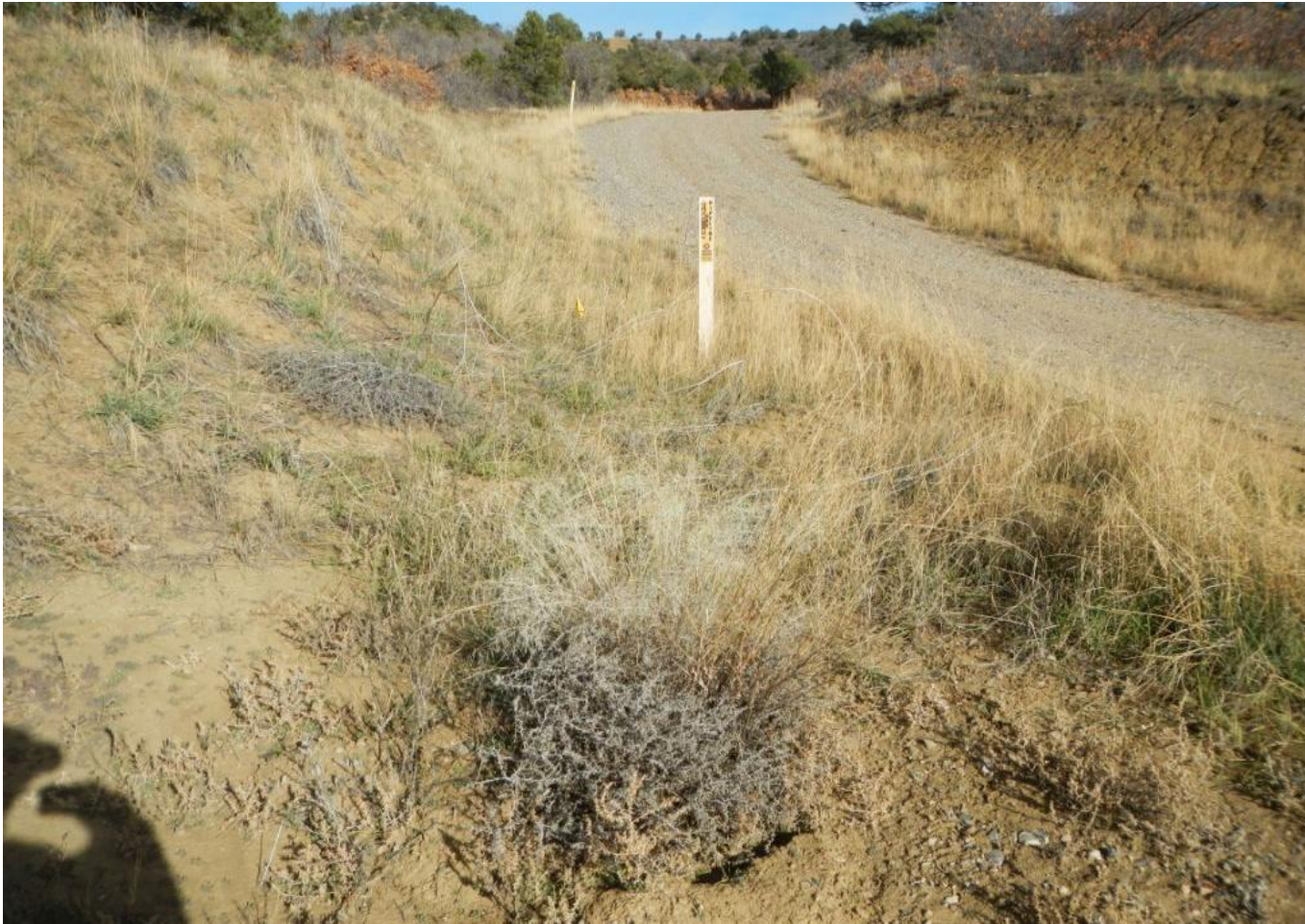
Photo 6. View of rill erosion in cut-slopes along access road near well pad entrance facing northward.
