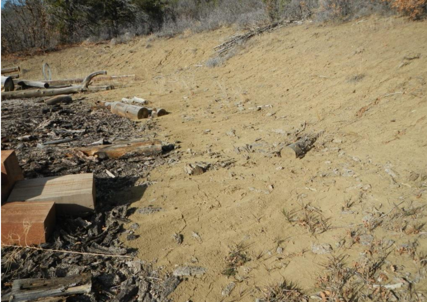
Photo 7. View of stormwater erosion in northeastern corner of project area from unstabilized cut-slope onto well pad.
