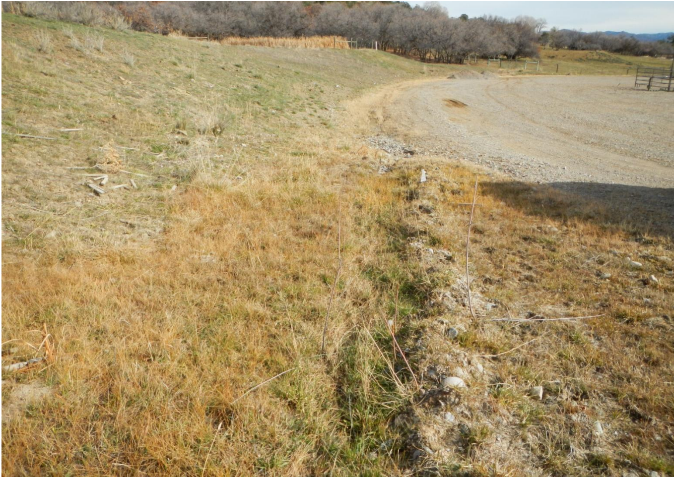
Photo 2. View of vegetated stormwater diversion ditch adjacent to northern edge of working area.
