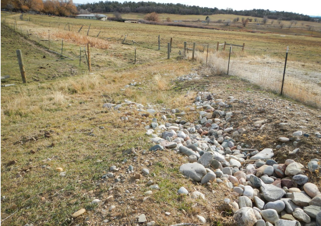
Photo 5. View of cobble revetment along stormwater channel exiting the southeastern corner of the project area.
