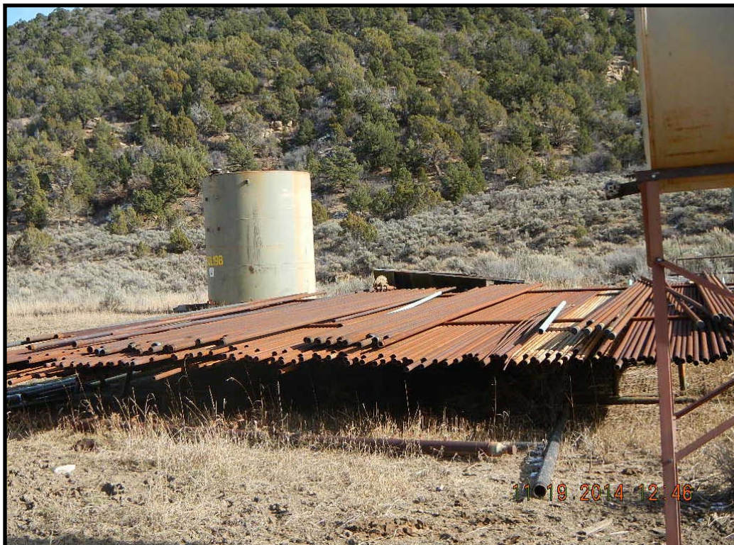
Pipe rack, unused tanks .
