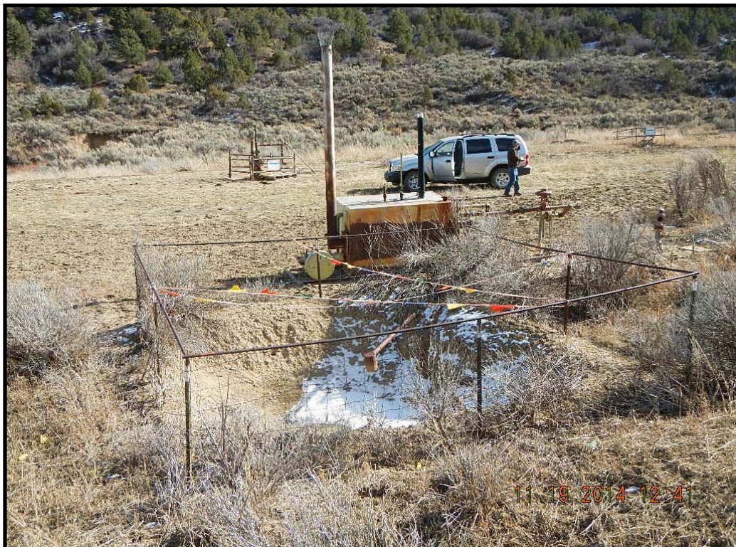
Inactive pit. Vegetation growing on the perimeter of the pit.
