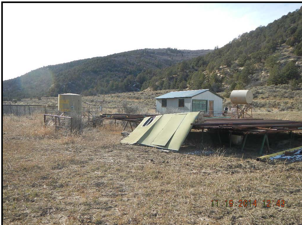
Wooden pipe rack, junk, unused tanks.
