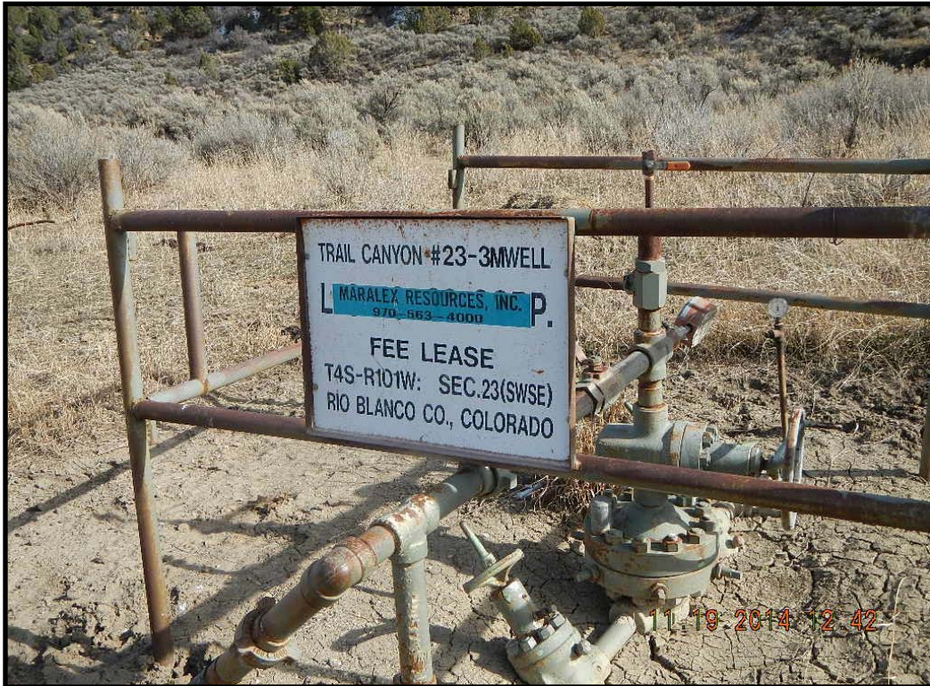
Shut-in well (since April 2011).
