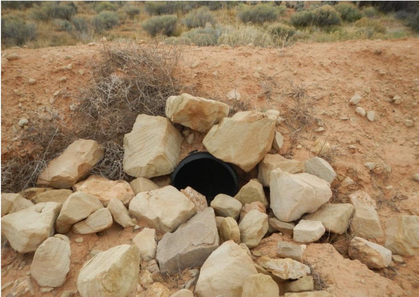
Photo 4. View of armored culvert in southwestern corner of project area.
