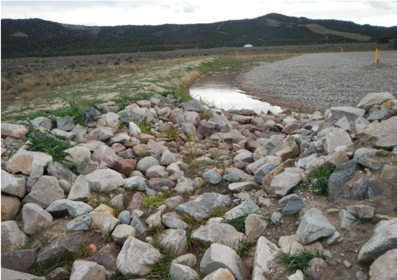
Photo 4. View of rock filter dam functioning to contain stormwater within the project area.
