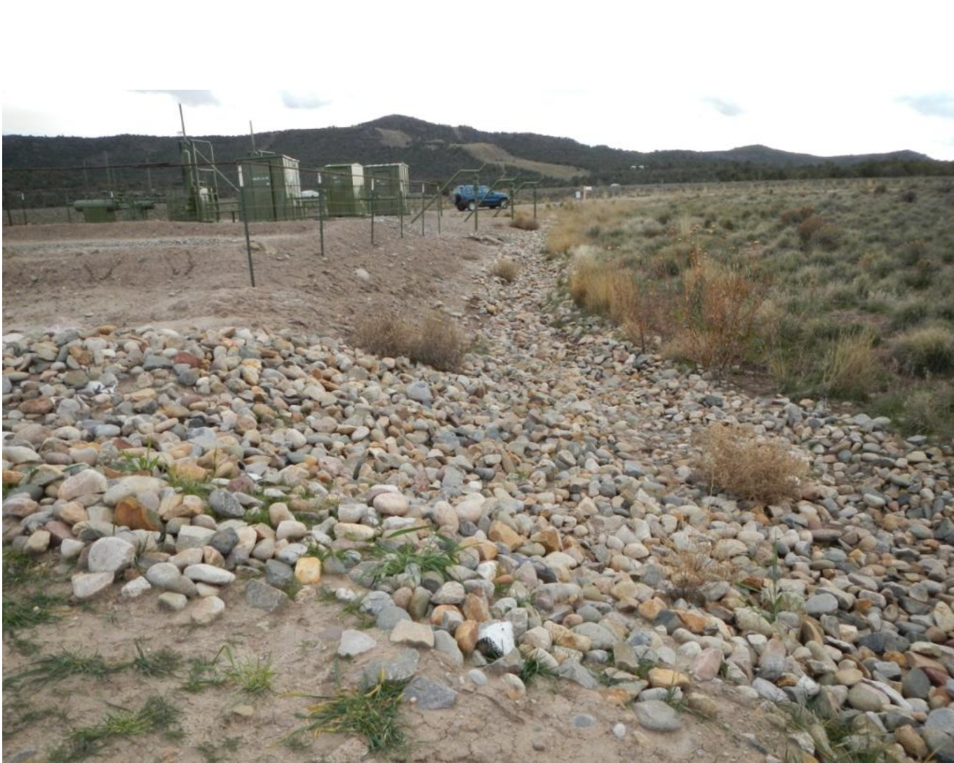
Photo 5. View of armored stormwater diversion channel in good condition.
