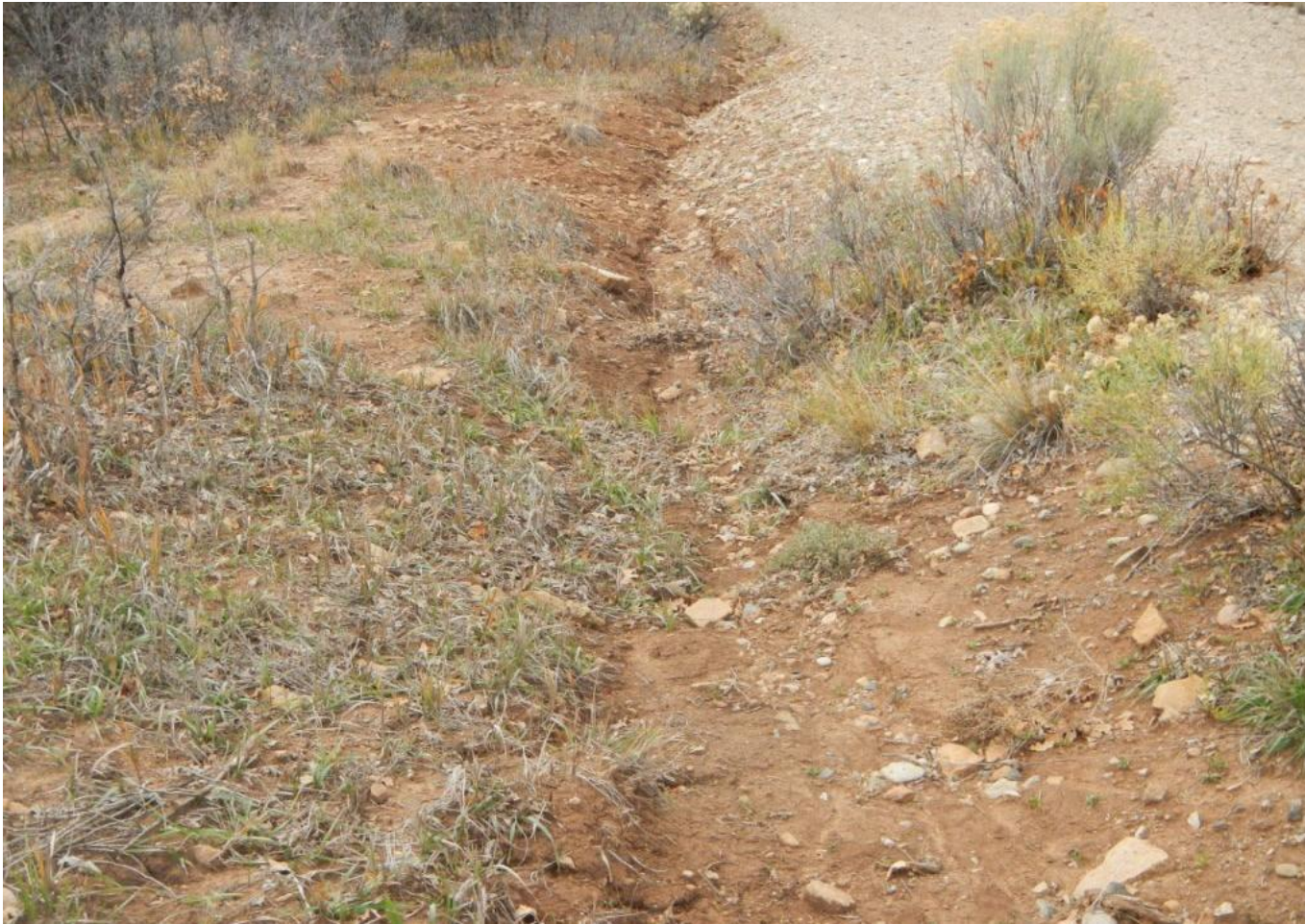
Photo 2. View of stormwater erosion and downcutting in roadside ditch along graveled portion of access road.
