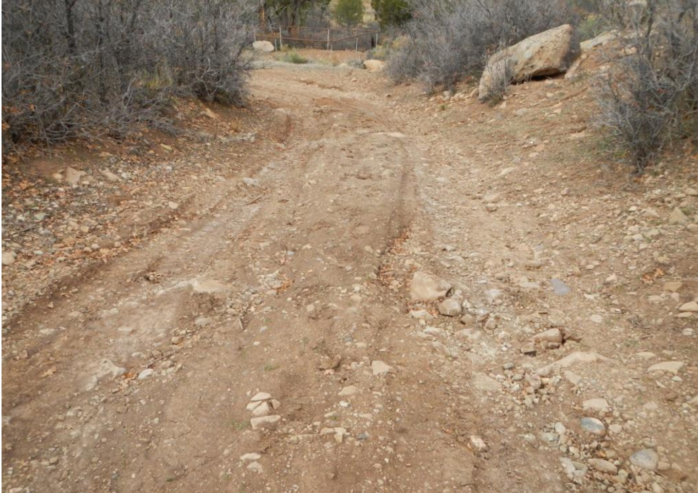
Photo 3. View of stormwater erosion on road surface of un-graveled portion of access road within project area upslope from project facilities.
