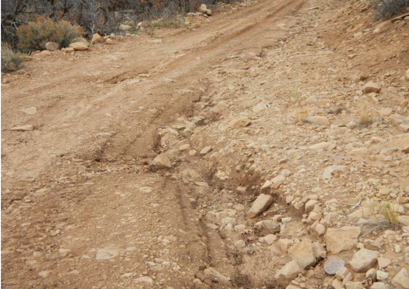
Photo 4. Another view of stormwater erosion and exposed rocks on surface of un-graveled access road near project facilities.
