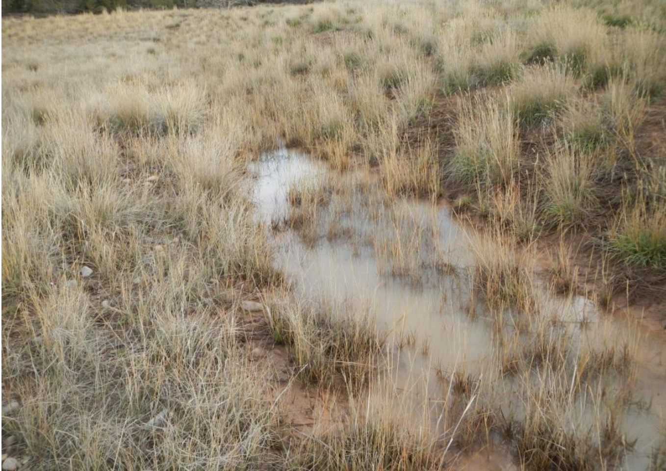
Photo 3. View of vegetated silt trap and vegetated swale functioning properly as a stormwater diversion.
