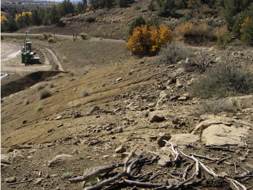
Northwest slope above well pad—Looking south-southwest
