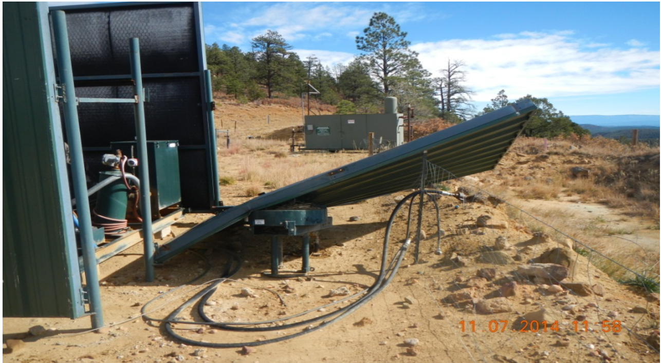
photo 3: Shed panel has fallen over.
