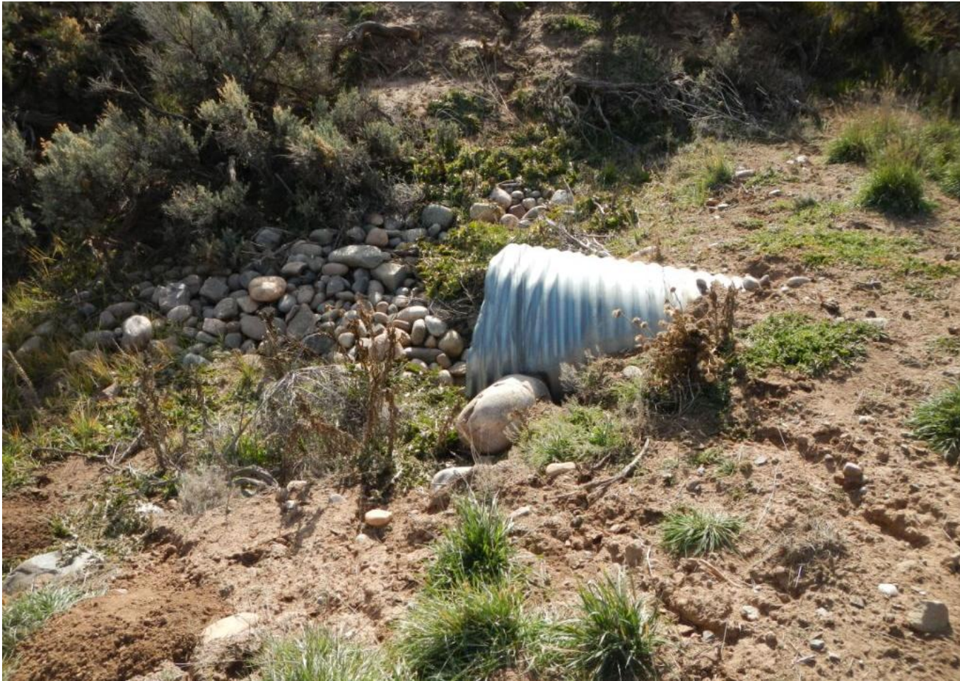
Photo 6. View of rill erosion and thistles around culvert inlet.
