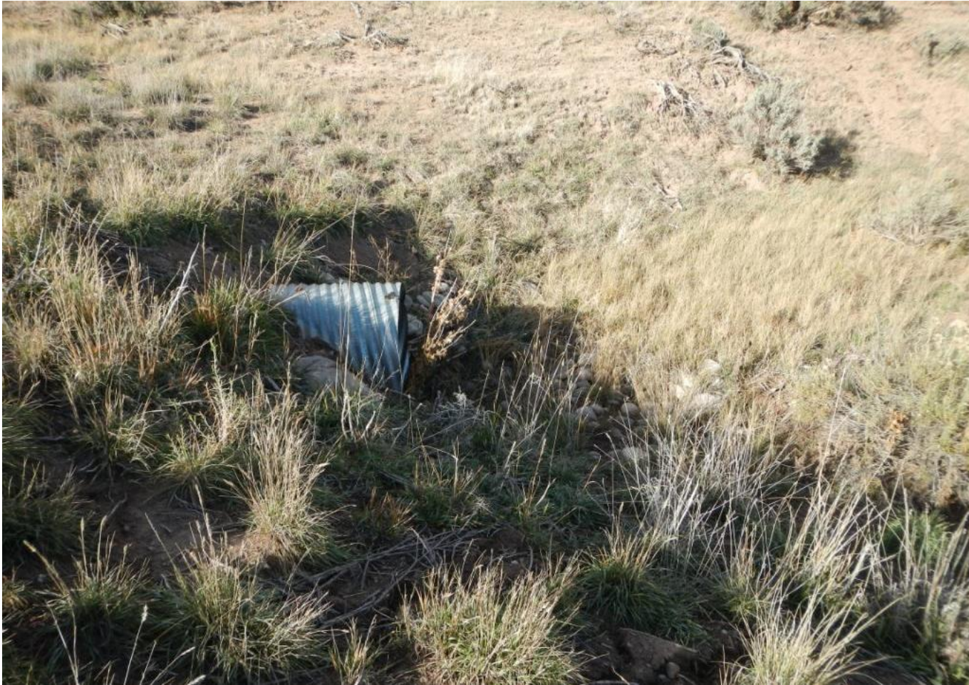
Photo 3. View of good revegetation and stabilization around culvert inlet.
