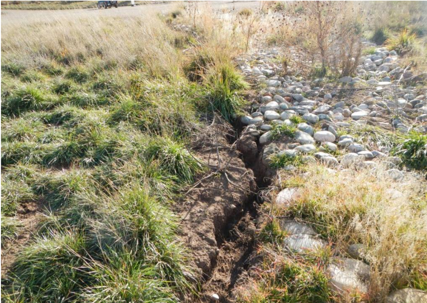
Photo 2. View of rill erosion adjacent to cobble BMP in northeastern portion of project area.
