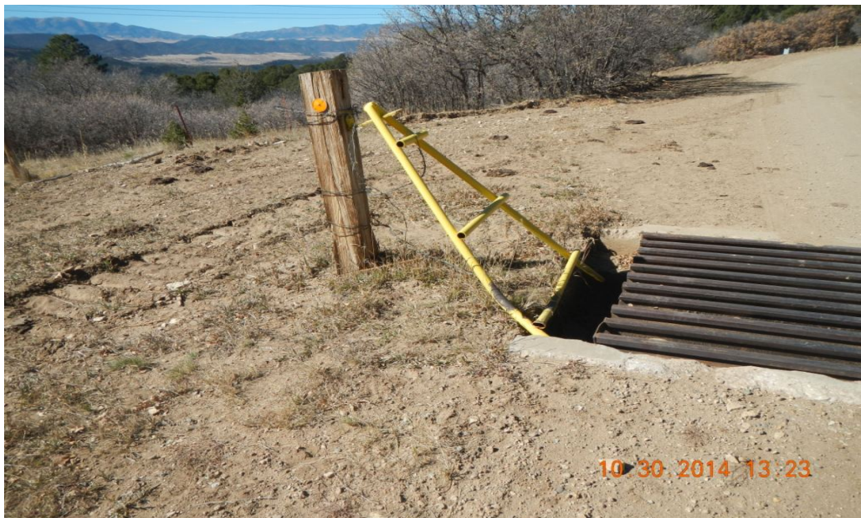
Cattle guard to this location is damaged
