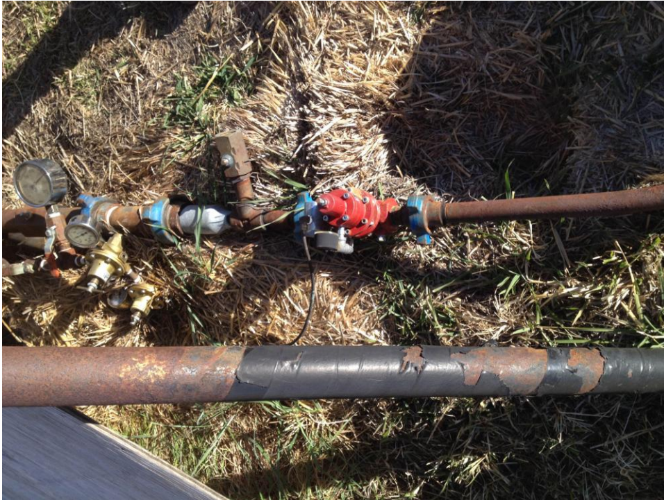
Bradenhead vent pipe and regulator system. Insulation on location at time of inspection is a little bit of straw and a piece of plywood. The \frac{1}{4} " pipe is plumbed from the casing at 2200psi.
