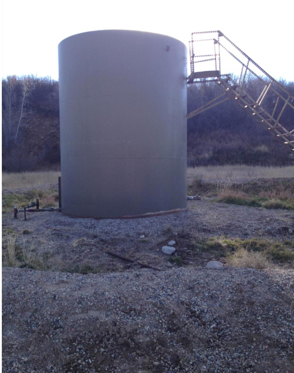
Produced water tank at time of inspection. Required labeling and placard not provided.
