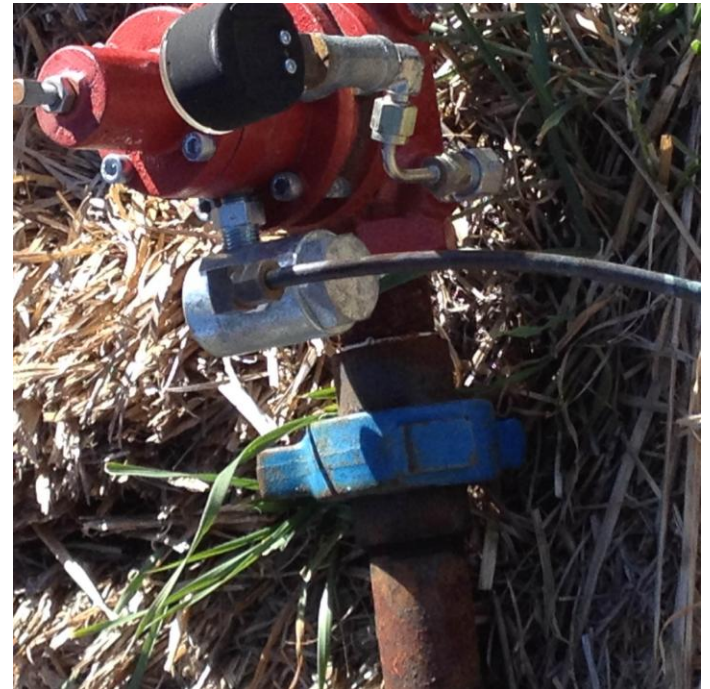
Bradenhead vent pipe and regulator system. Insulation on location at time of inspection is a little bit of straw and a piece of plywood. The \frac{1}{4} " pipe is plumbed from the casing at 2200psi.
