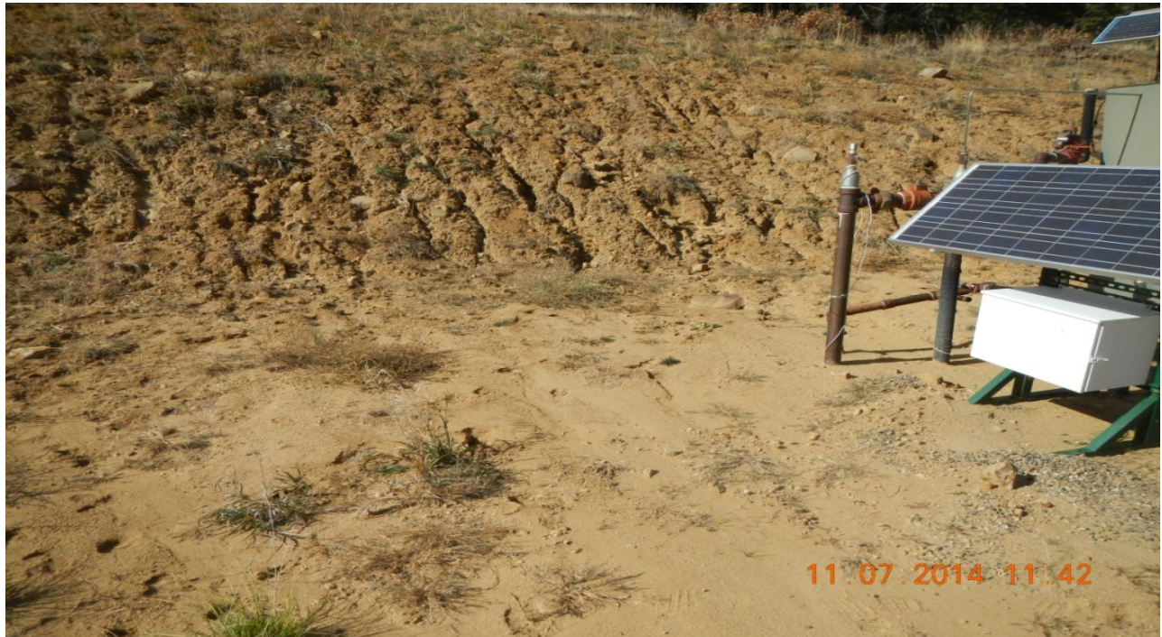
Erosion rills off the slope at the West side of location
