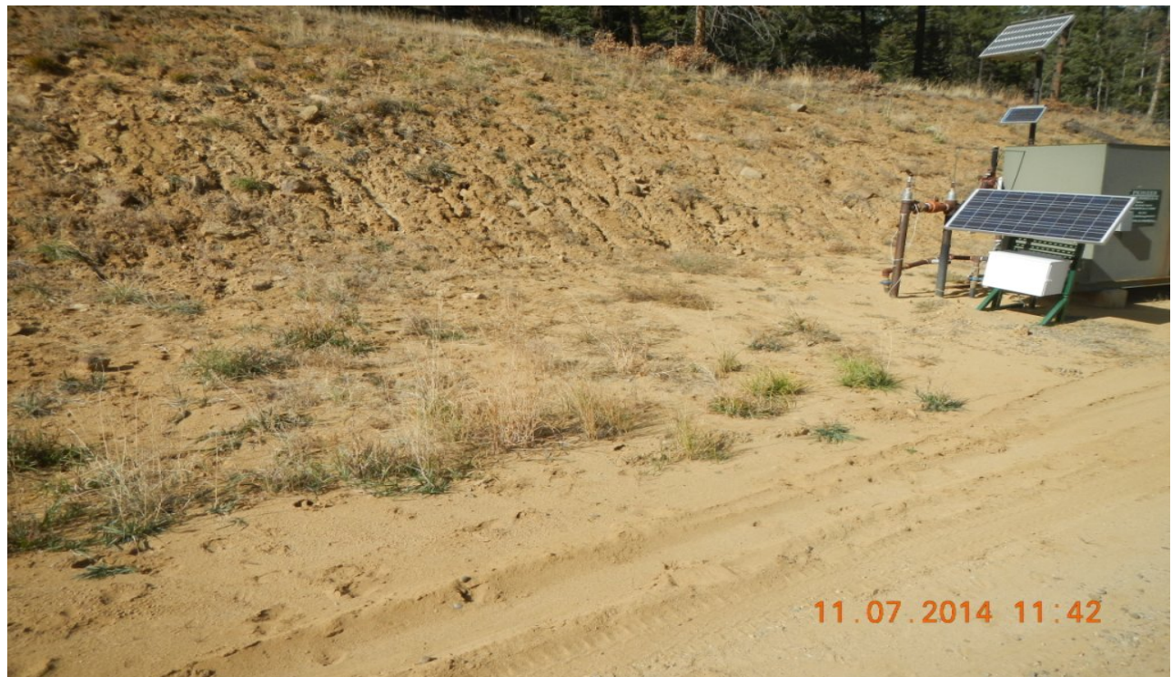
Erosion rills off the slope at the West side of location
