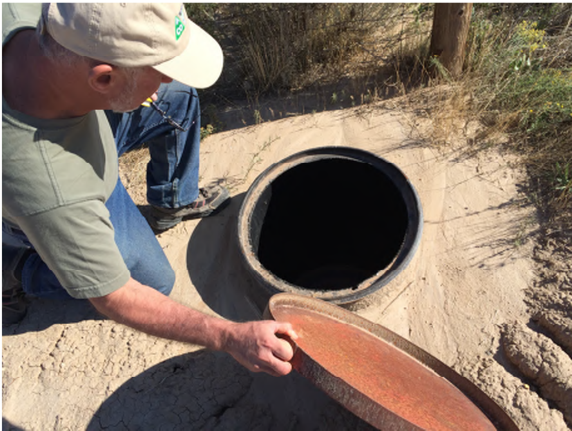
Photograph 2: Leak Detection Manhole
