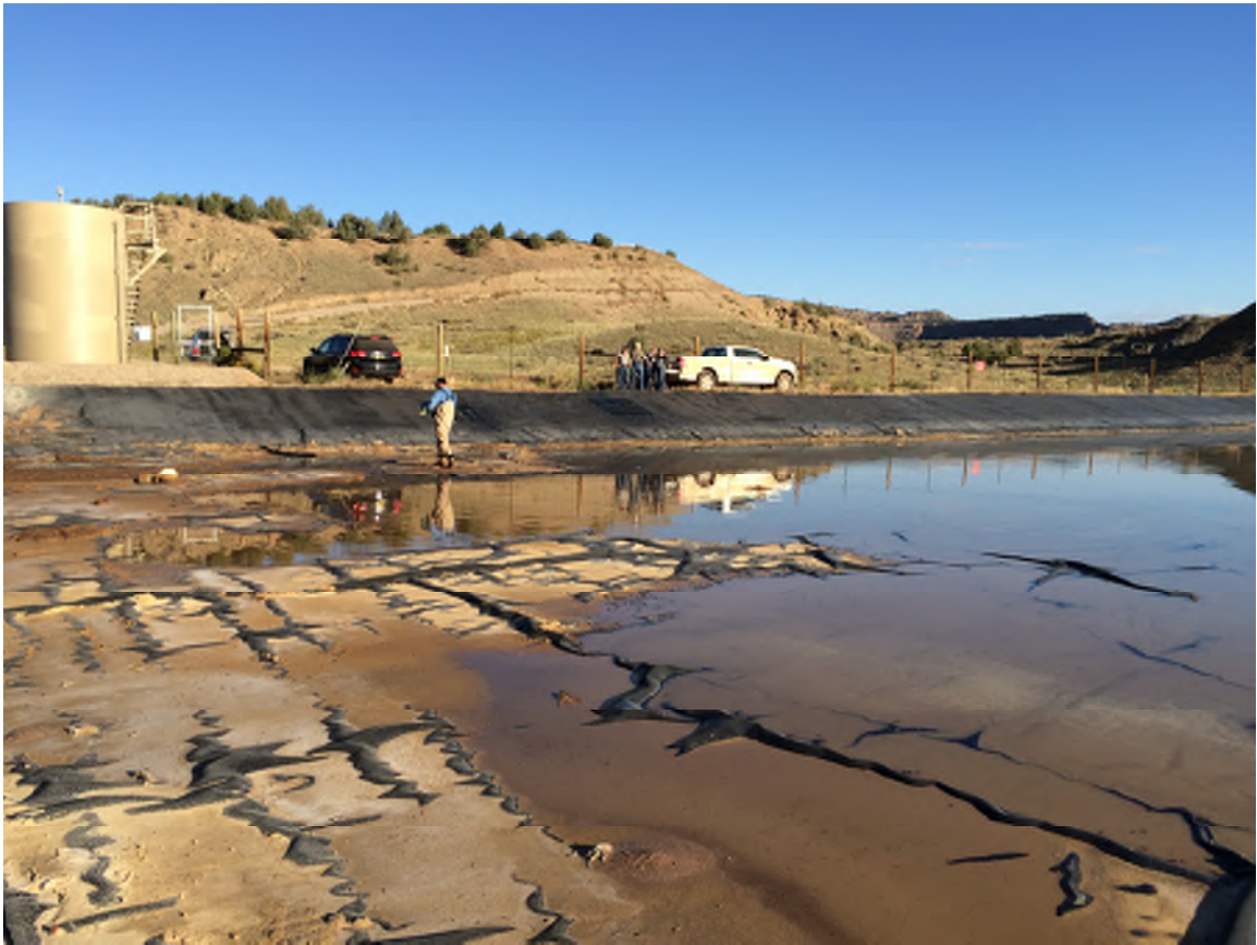
Photograph 3: View looking west at exposed liner on south side of pit
