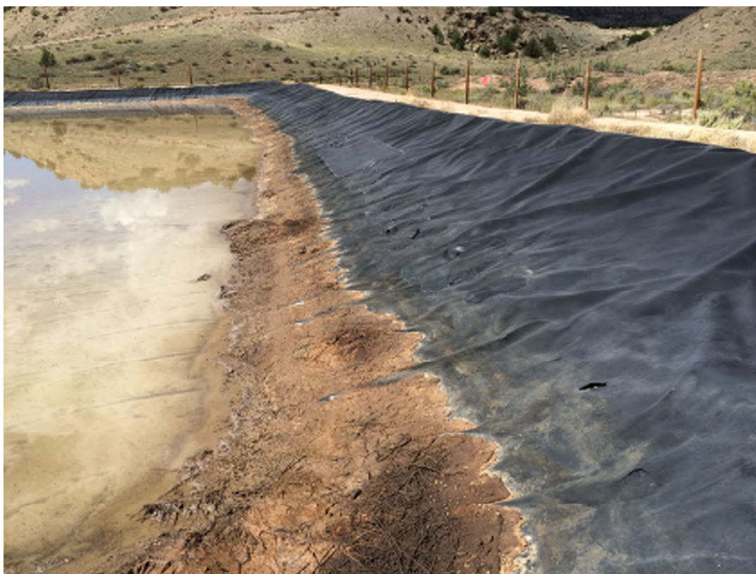
Photograph 6: View of deteriorated Panel 14 along north side of pit. Note the holes and patches are all generally located at or below the high water mark.
