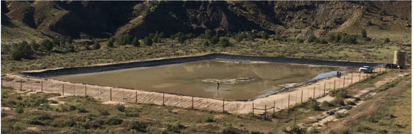
Photograph 1: View looking south of pit during leak testing. Note the LLSI testing person and exposed liner in the central portion of the pit and along the southern boundary.
