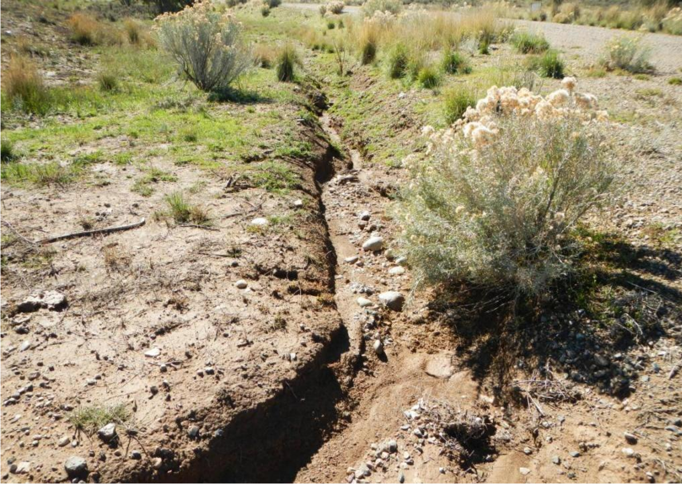
Photo 3. View of erosional drainage forming along the eastern edge of the access road near the entrance to the well pad.
