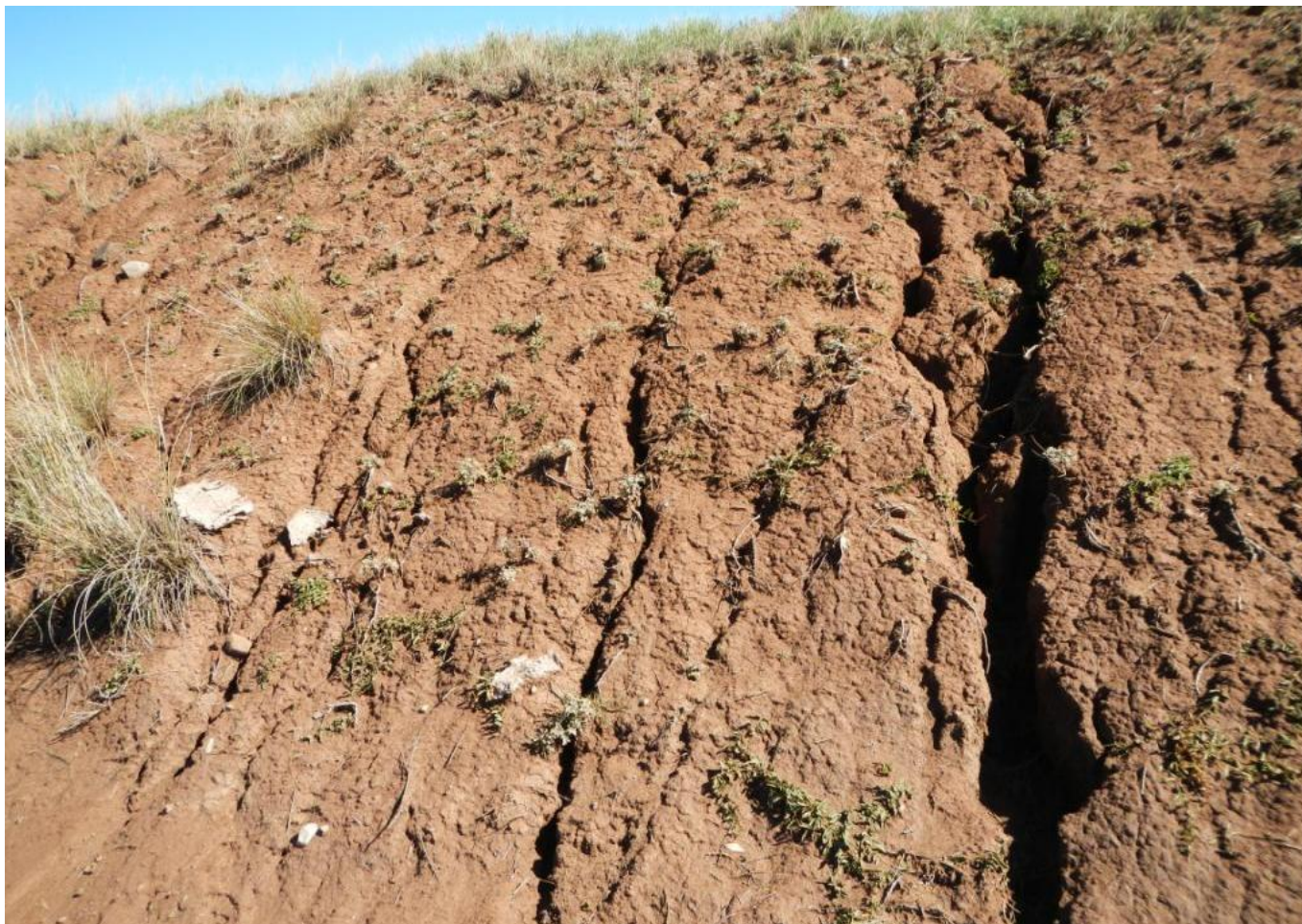
Photo 5. View of rill erosion on one of the cut slopes within the project area.
