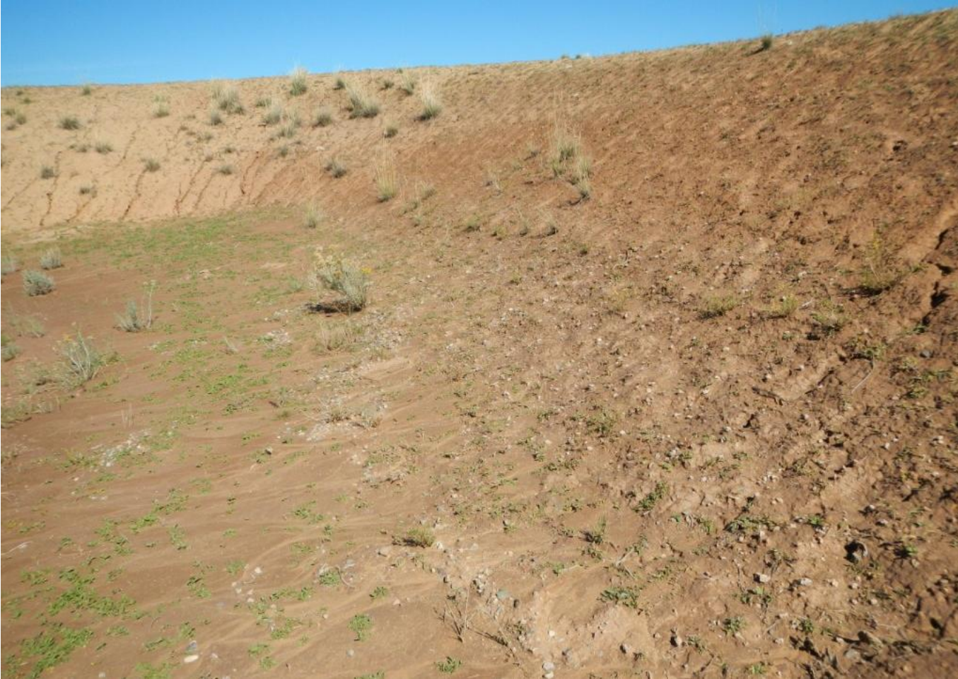
Photo 6. View of rill erosion and sediment deposition below cut slopes within the project area.
