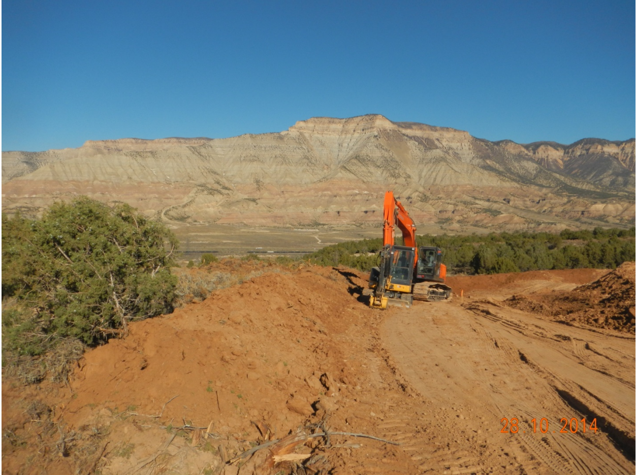
15. Pad Western perimeter, viewed North from center of Western perimeter.
