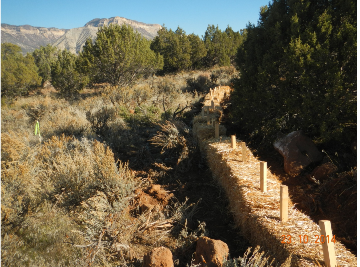
5. Pad Northern perimeter, viewed east from NW corner.
