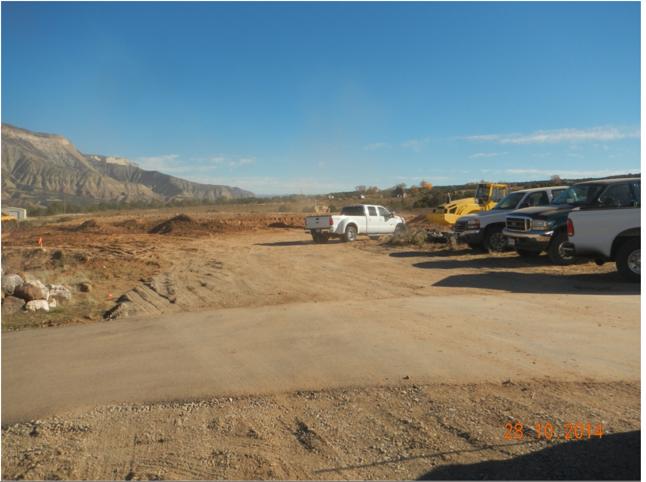
13. Location access road entrance, viewed SW from NE.
