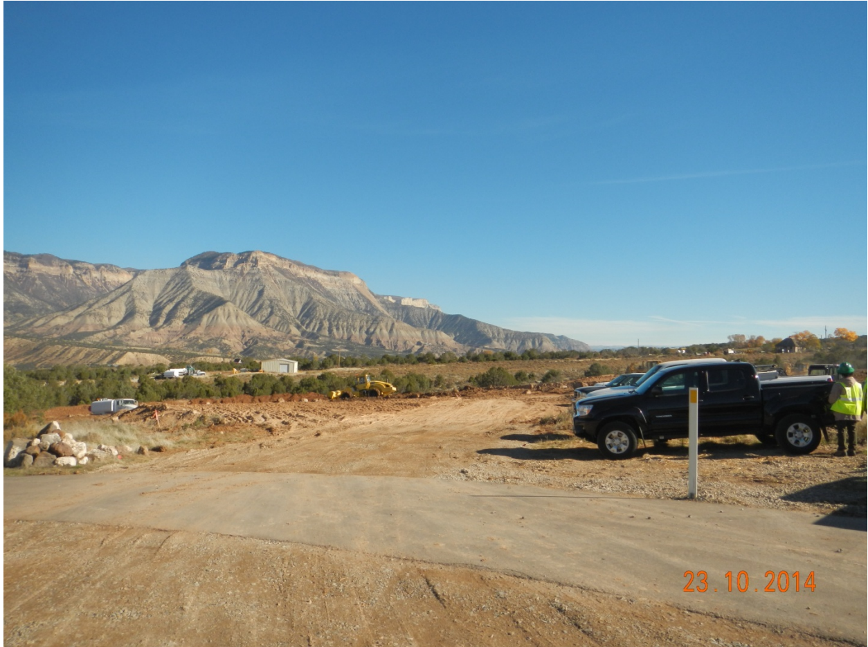
2. Location access road entrance, viewed SW from NE.
