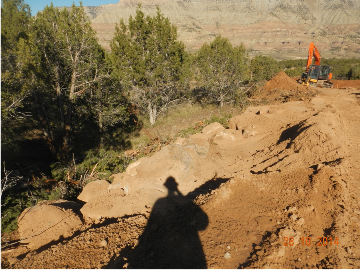
14. Pad Western perimeter, viewed North from entrance.
