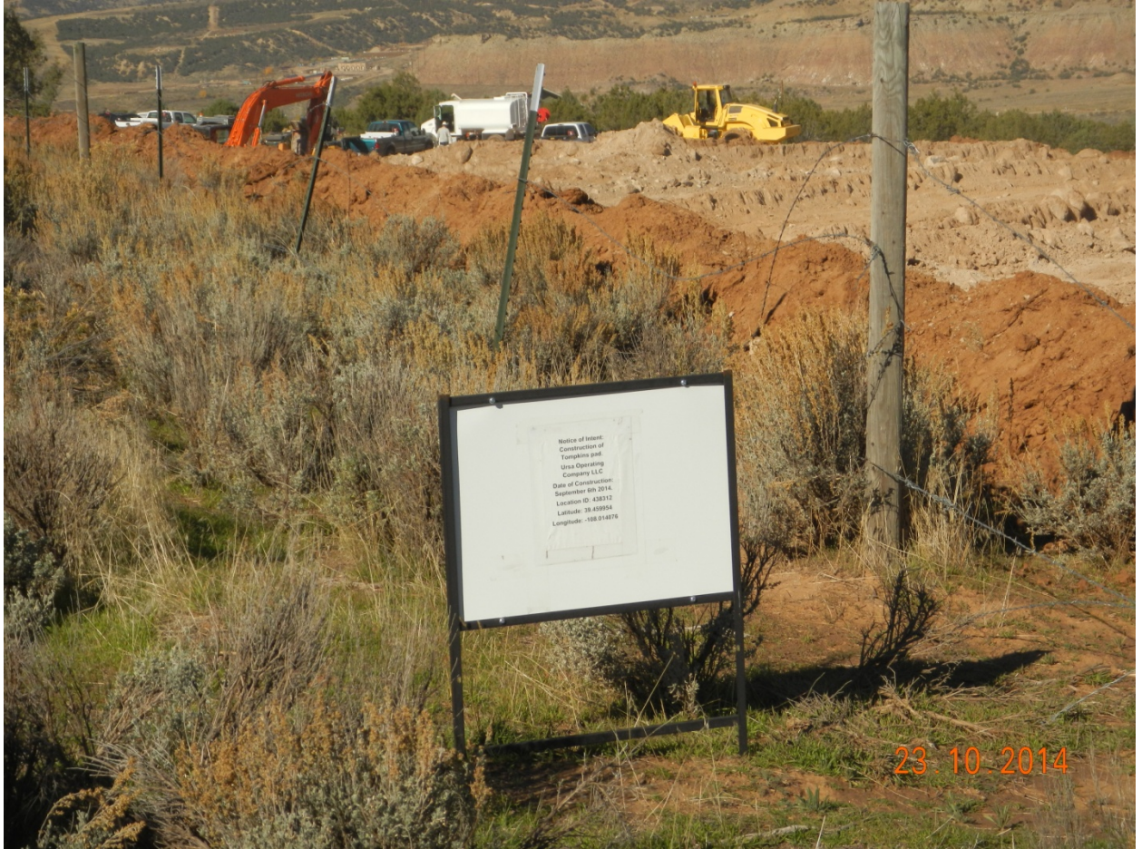
11. Pad Southern perimeter and location sign, viewed West from SE corner.
