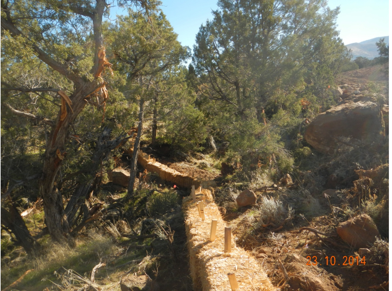
6. Pad Eastern perimeter, viewed South from center of perimeter.
