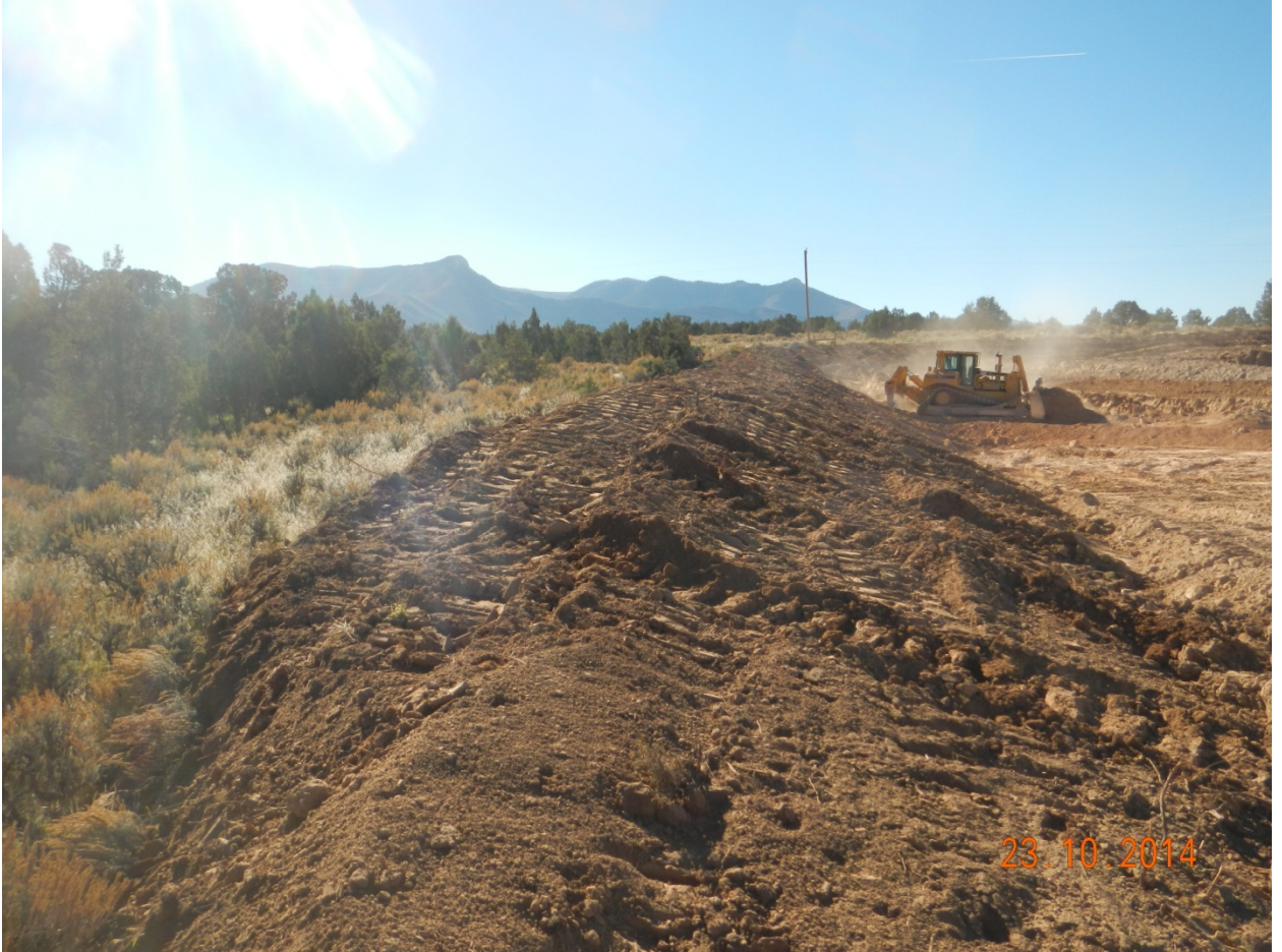
10. Pad Eastern perimeter, viewed South from SE quarter along perimeter.
