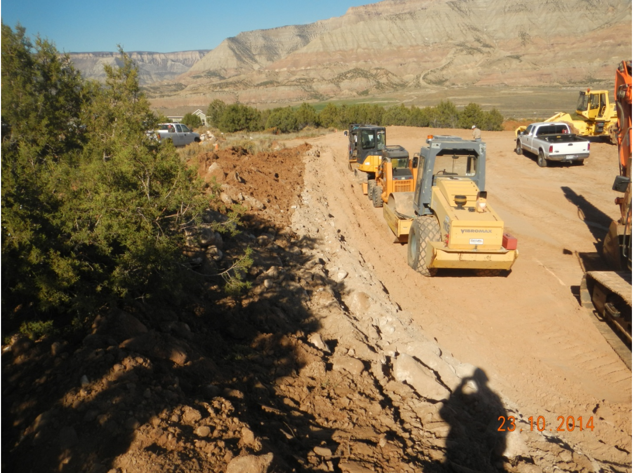
12. Pad Western perimeter, viewed North from SW corner.
