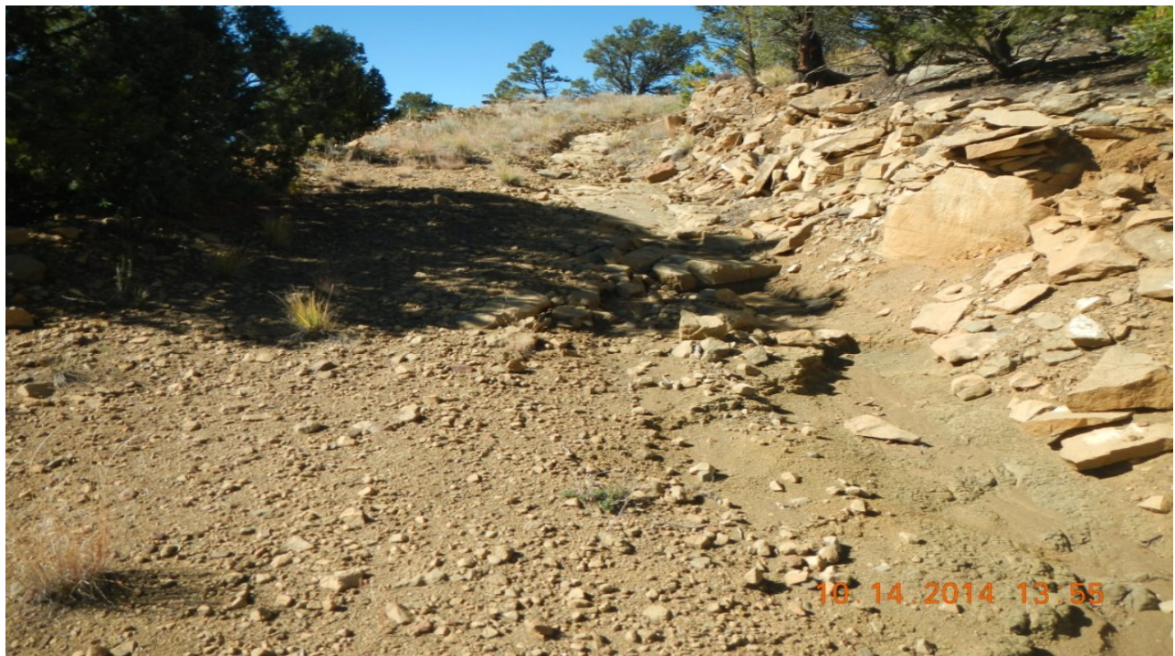
Erosion occurring at lower portion of access road
