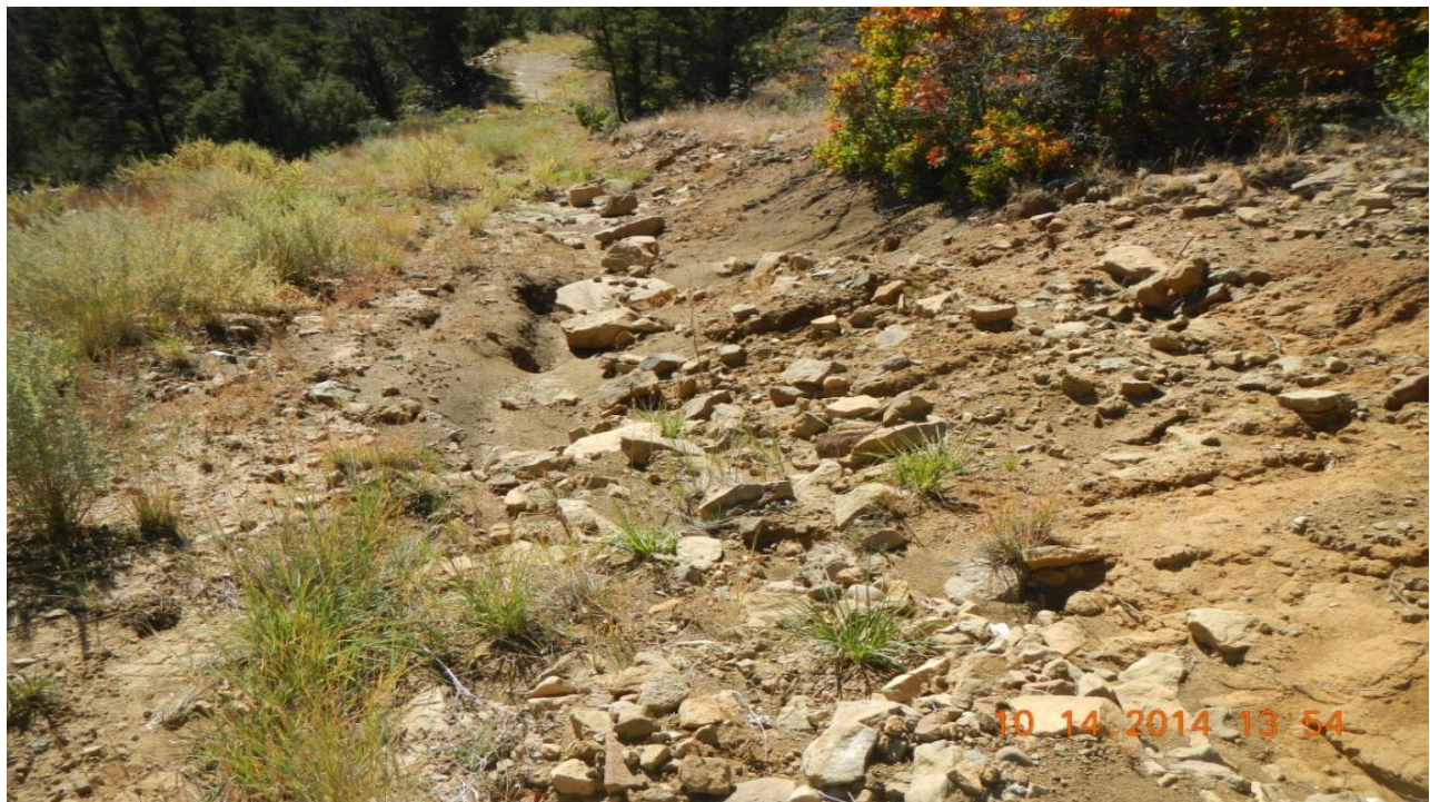
Erosion occurring at top portion of access road
