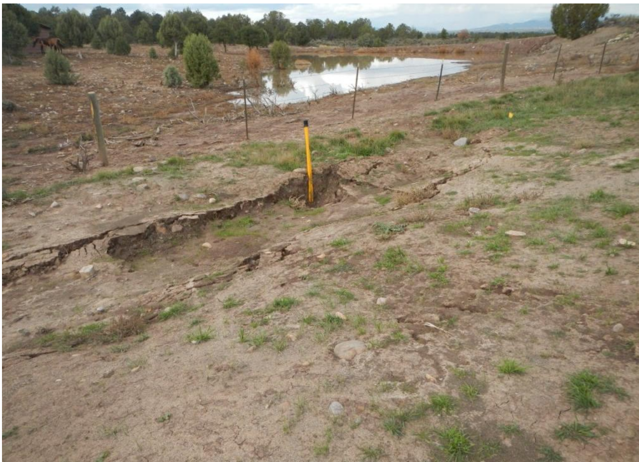
Photo 2. View of subsidence shown in Photo 1 facing westward, perpendicular to what appears to be a pipeline tie.
