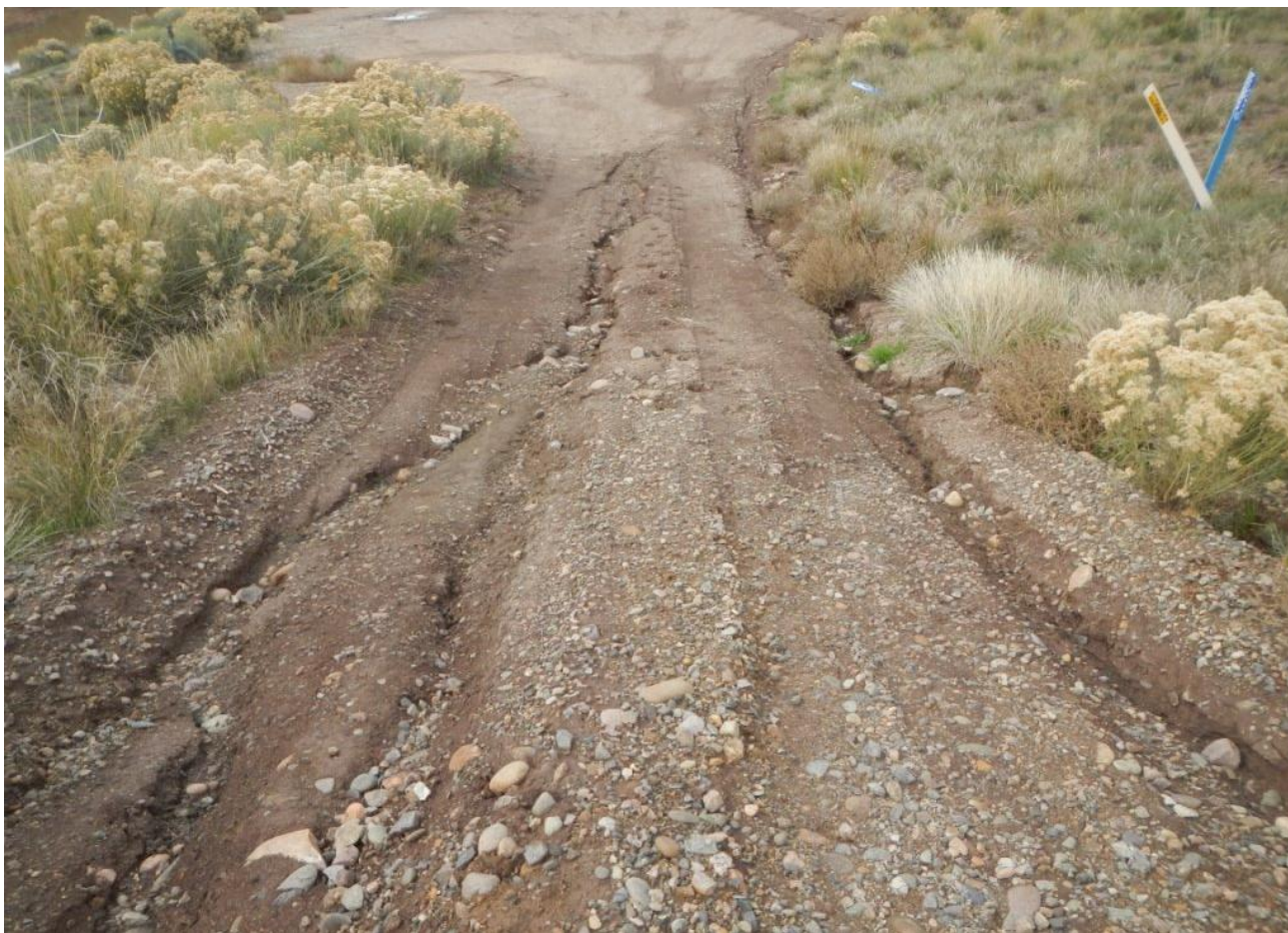
Photo 3. View of erosion on the access road from the edge of the adjacent Samson well pad facing toward the project area.
