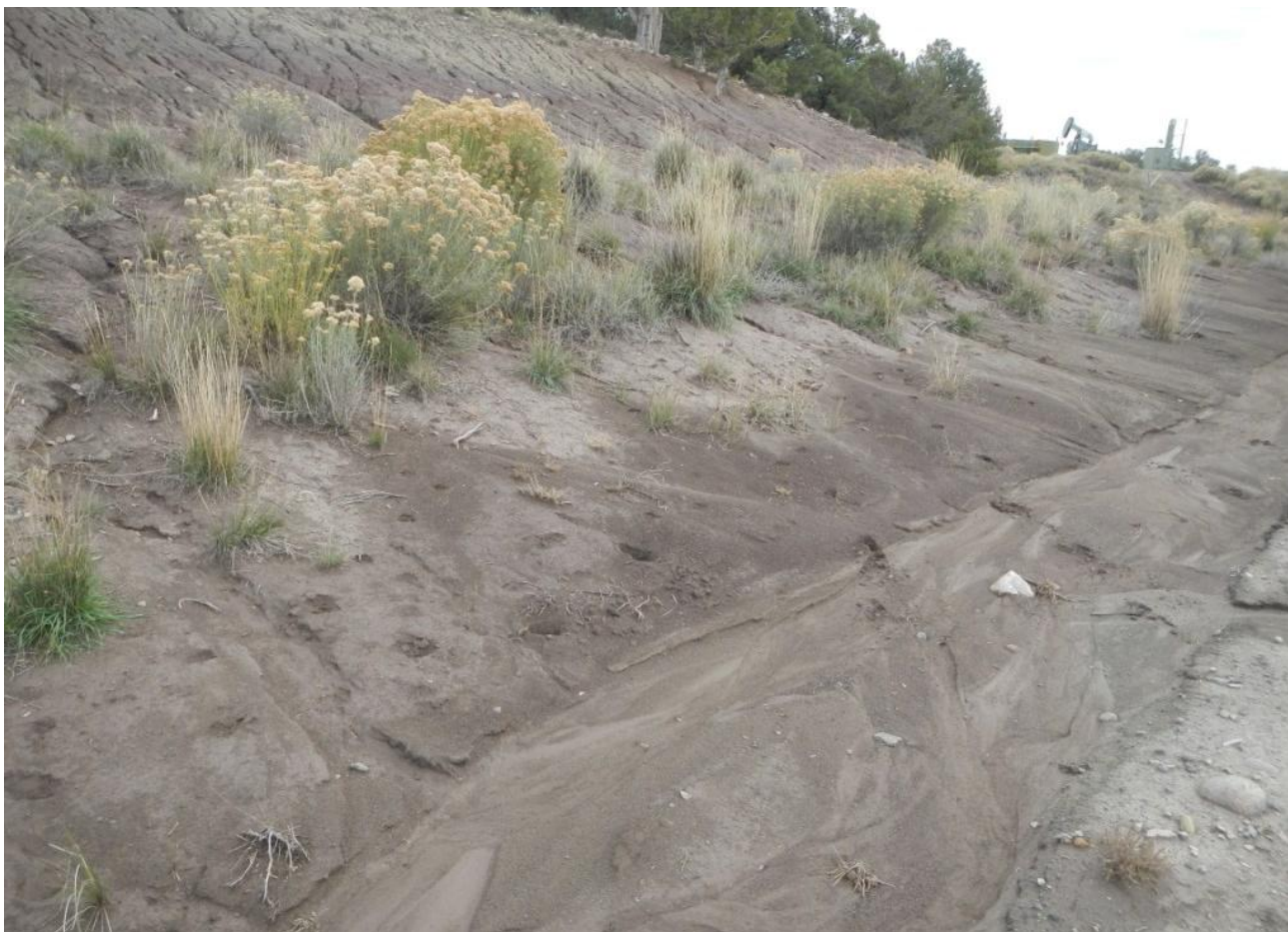
Photo 11. View of stormwater erosion channel upstream from Photo 10 and rill erosion on cut slopes of project area.
