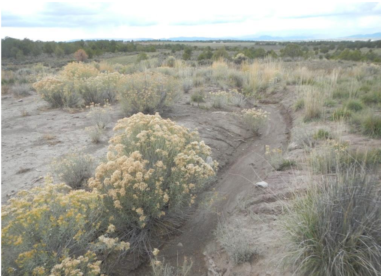
Photo 10. View of diverted stormwater flow channel from cut slopes on northeastern edge of project area flowing toward old pit (facing northward).
