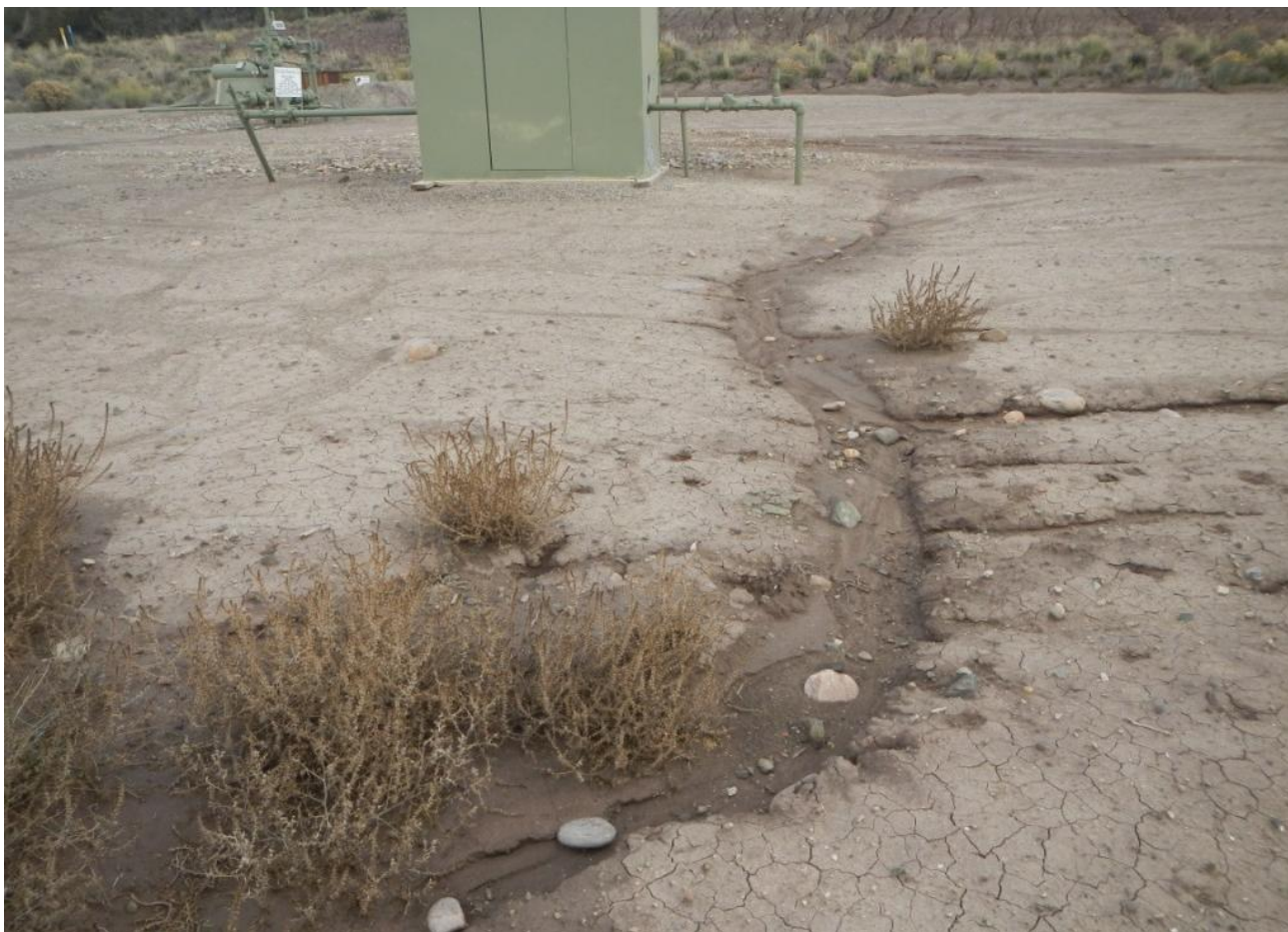
Photo 5. View of erosion on the surface of the well pad flowing toward the southwestern edge of the project area.
