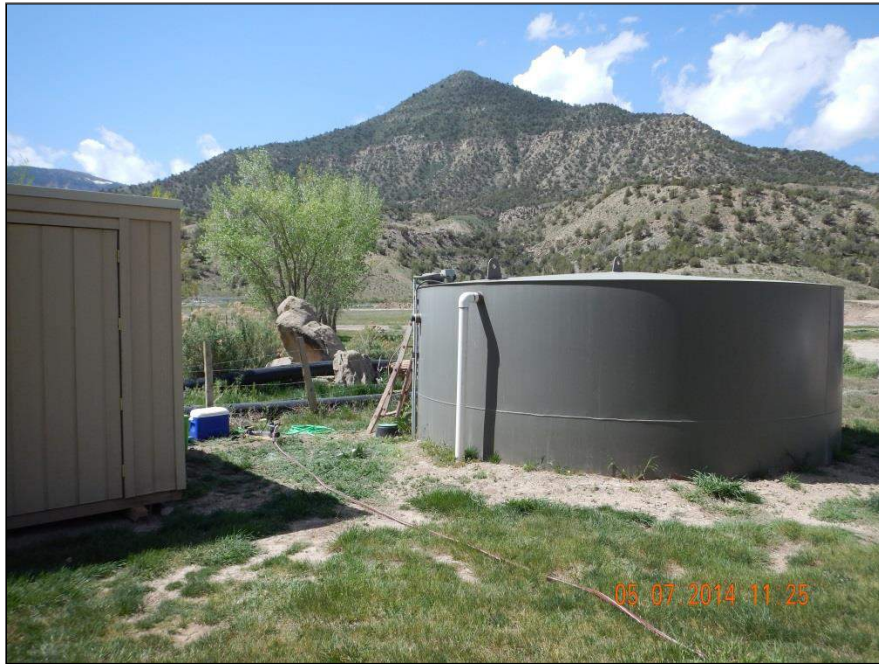
Photo 1. Union 76 Water Well No. 6 Sampling Location (Union No. 6-26068-F); cistern
