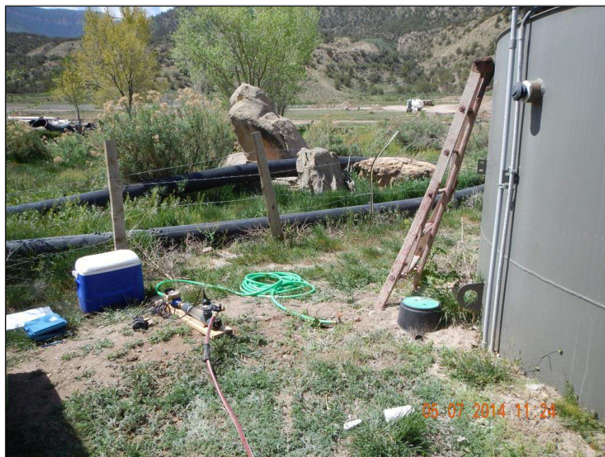
Photo 2. Union 76 Water Well No. 6 Sampling Location (Union No. 6-26068-F); cistern
