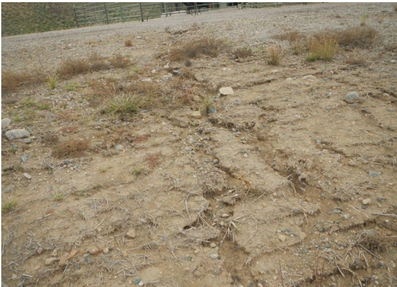
Photo 5. View of rill erosion within the western portion of the interim reclamation area.
