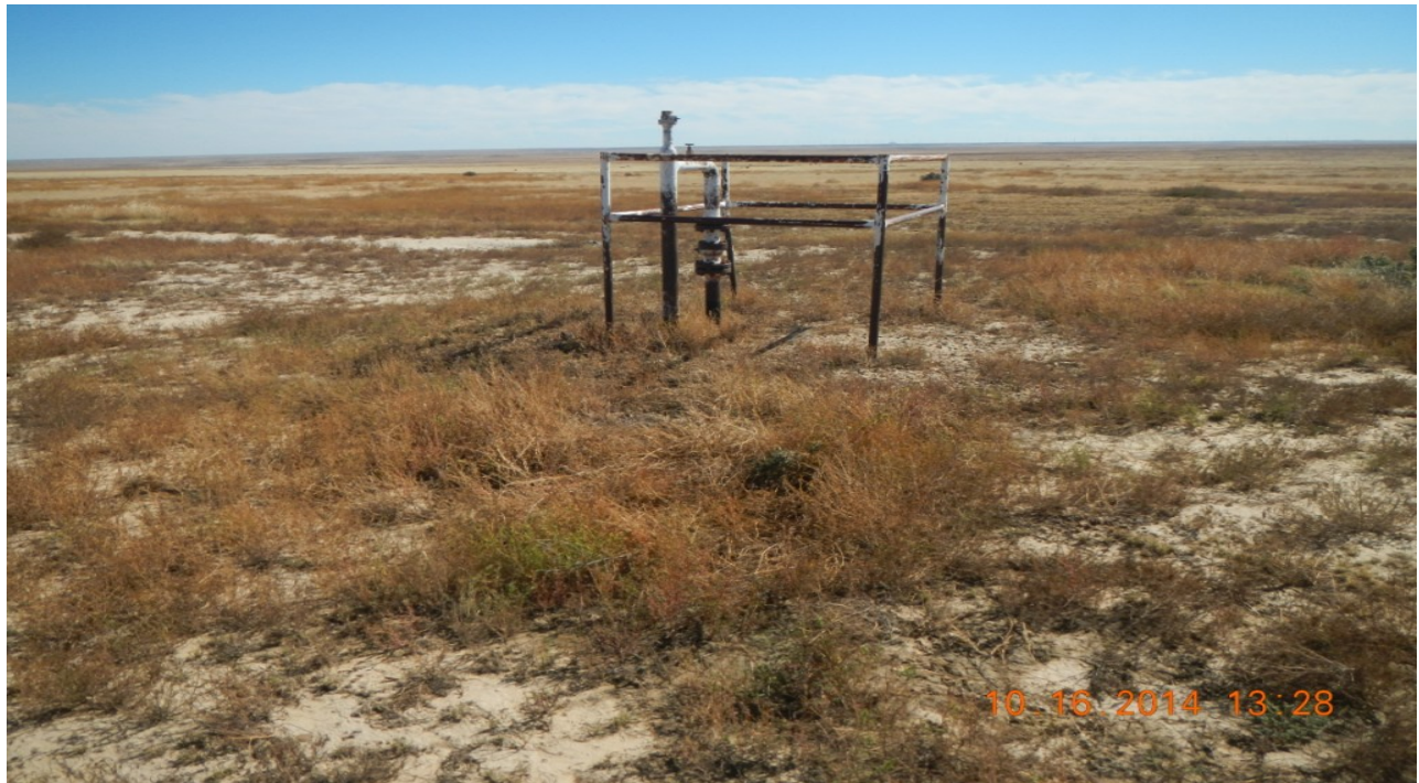
Pipeline riser on East side of location
