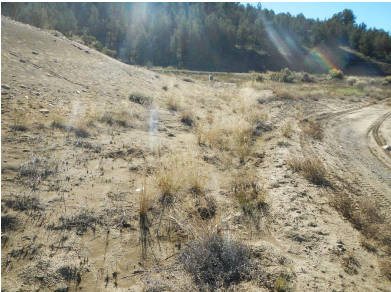
Photo 6. View of sediment deposition from cut slope on the eastern edge of the project area. Appears to be largely contained by the vegetated diversion adjacent to the access road.
