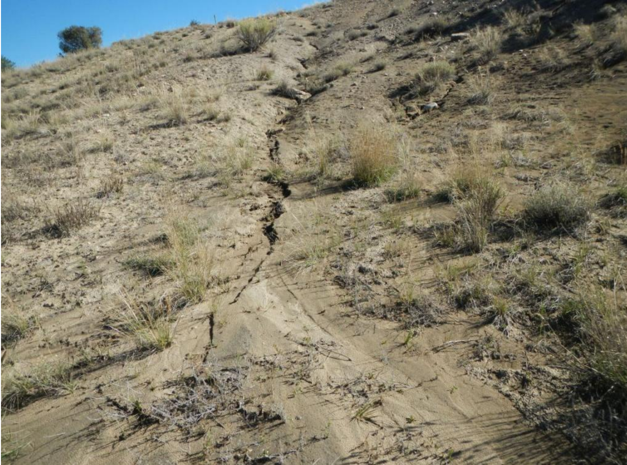
Photo 6. View of large rill within cut slope that needs to be monitored.
