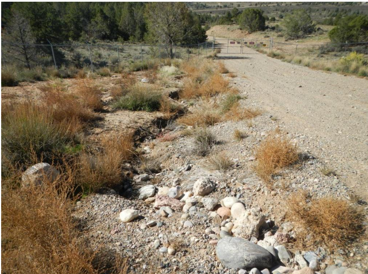
Photo 3. Erosional channel forming along the eastern side of the access road.
