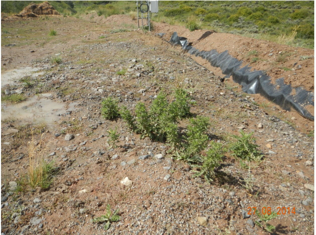
12.) Southwest corner sediment BMP will need velocity reduction/ sediment detention in near future (1).
