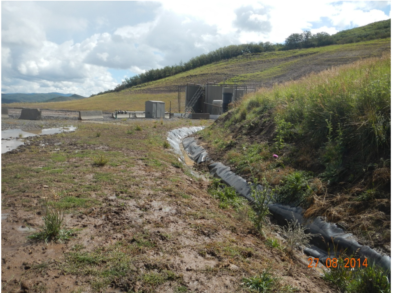
15.) Southwest corner (East side) sediment BMP will need velocity reduction/ sediment detention in near future (2).
