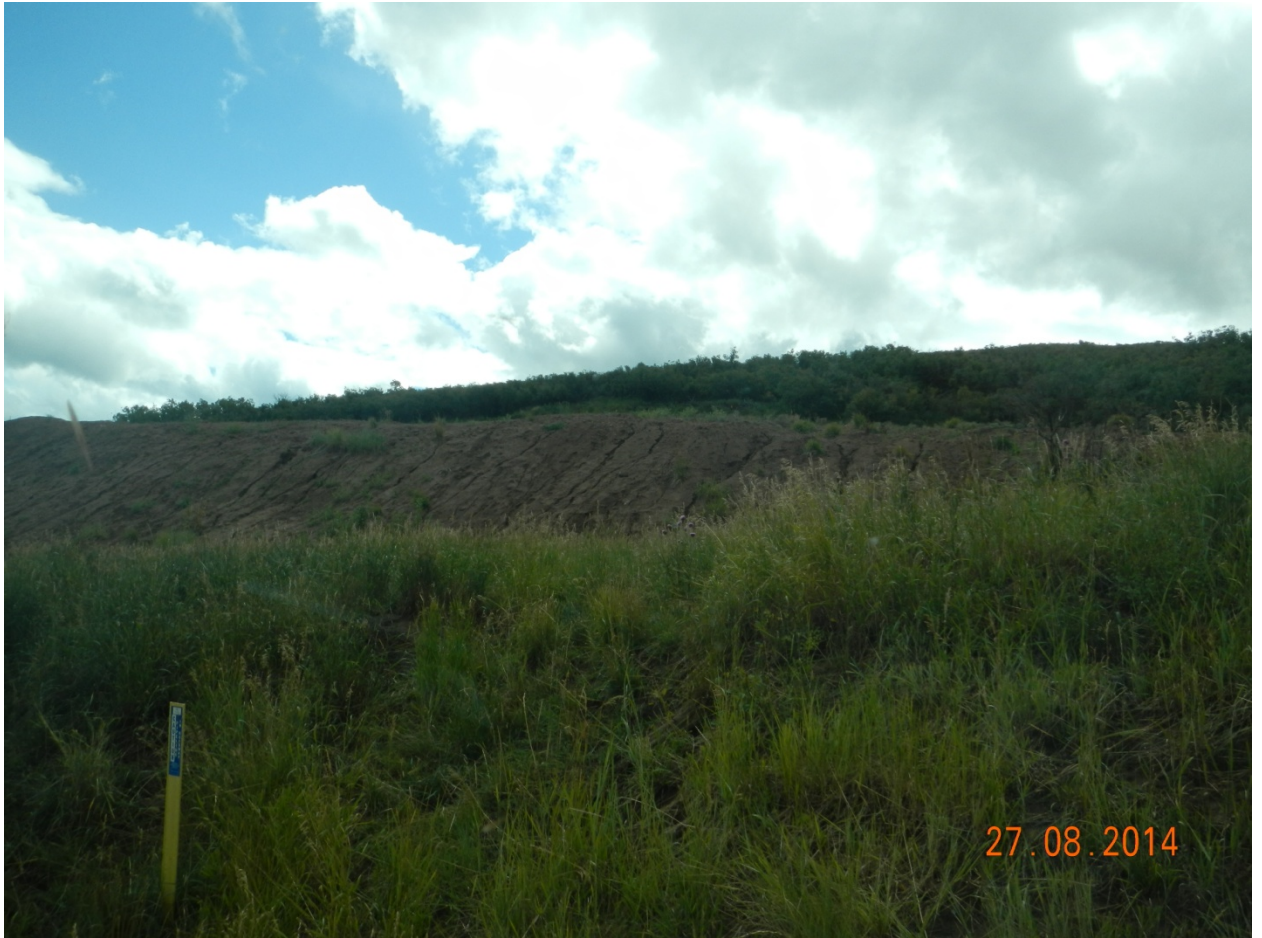
2.) Rilling on Fill below access sign, uphill from access road on South Side.
