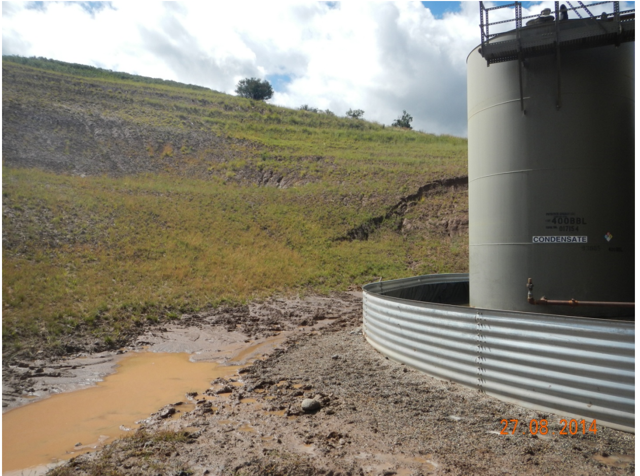
17.) Eastern perimeter cut sloughing, rilling and sediment.
