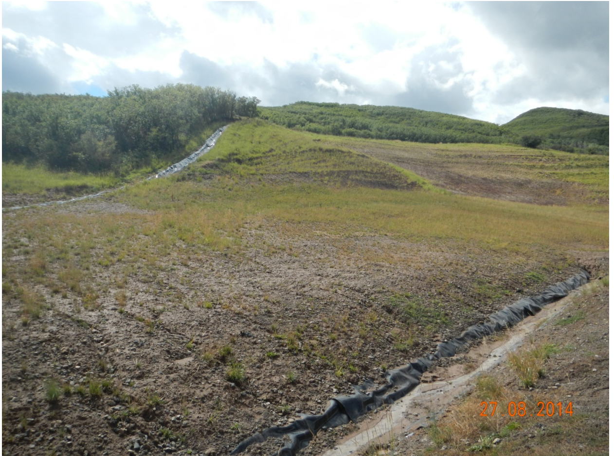
19.) Pad from Northern disturbed appendage looking Southwest. Stormwater BMPs need velocity reduction/ sediment detention.
