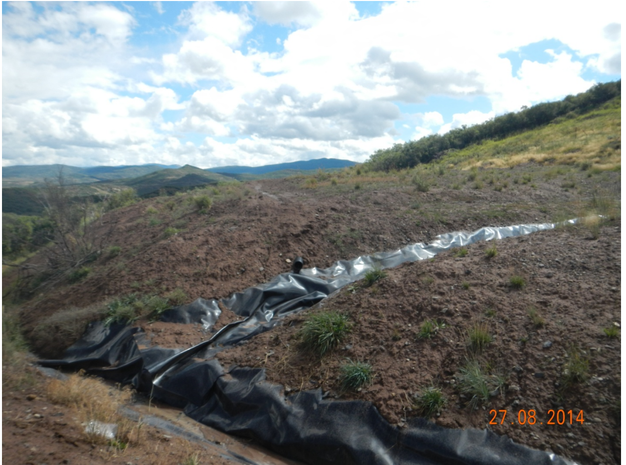
18.) Northeastern BMP needs velocity reduction/ sediment detention.
