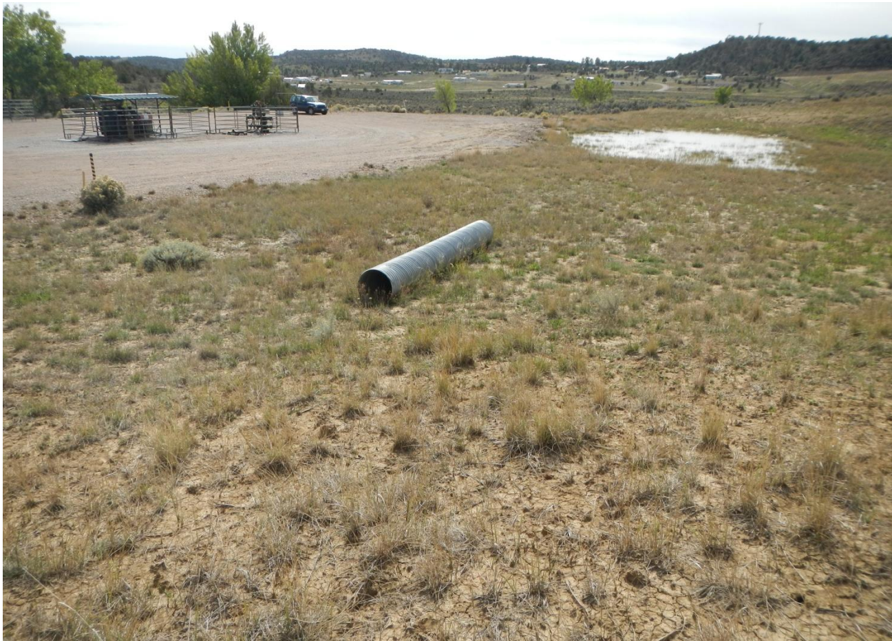
Photo 6. View of unused culvert in project area.
