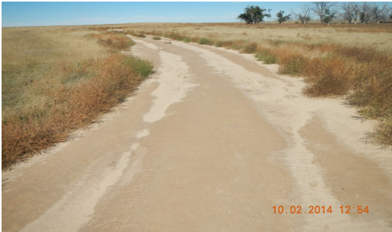
Access road has very little vegetation growth
