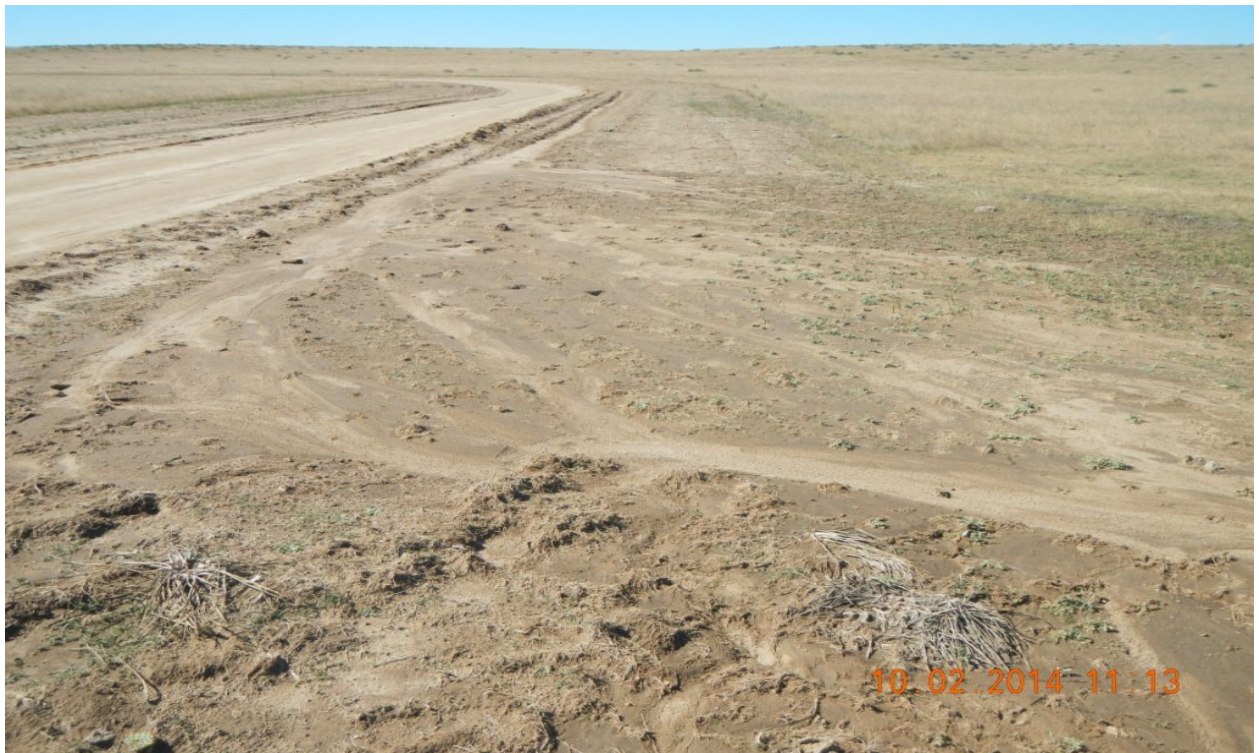
Erosion from access road transporting sediment into adjacent pasture
