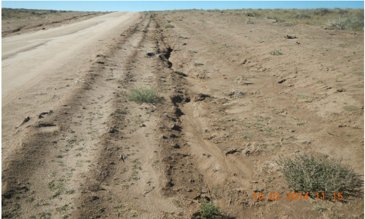
Erosion riling along access road
