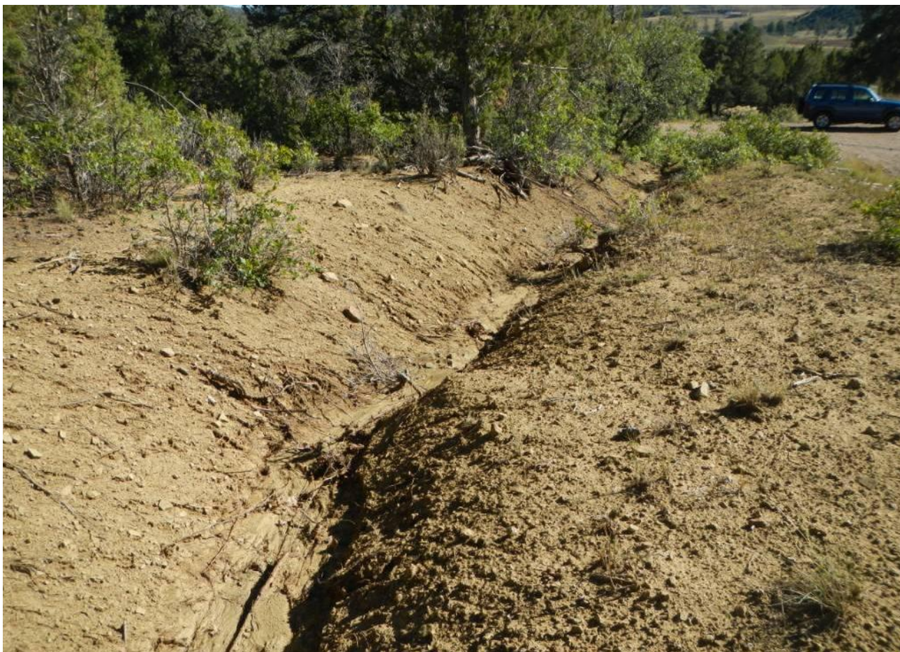
Photo 8. View of water diversion channel on the eastern edge of the project area. Storm water flows appear to move rapidly through this area; down cutting the channel, and carrying sediment off of the location.
