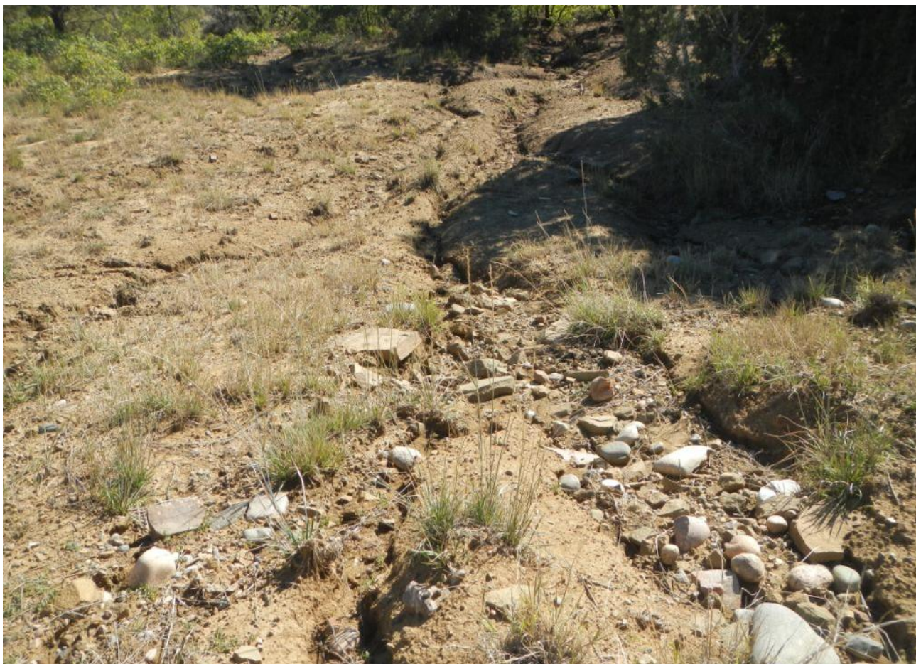
Photo 3. View of continued deep rills and gully forming in the fill slopes within the southern portion of the interim reclamation area.
