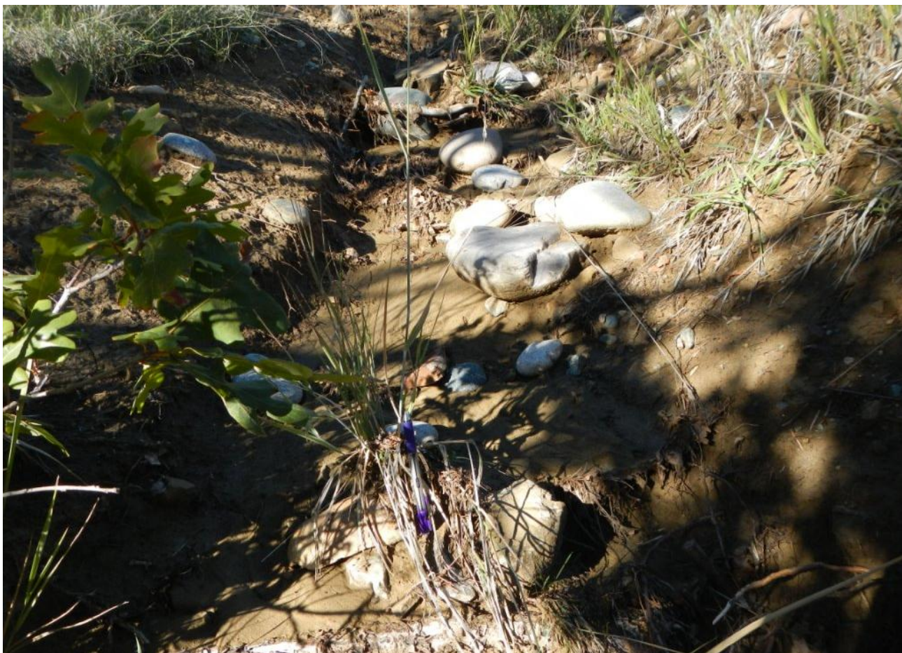
Photo 5. View of water diversion channel on the western edge of the well pad. Approximately six inches of soil has recently been removed as evidenced by the exposed roots on the living grass within the channel bottom.
