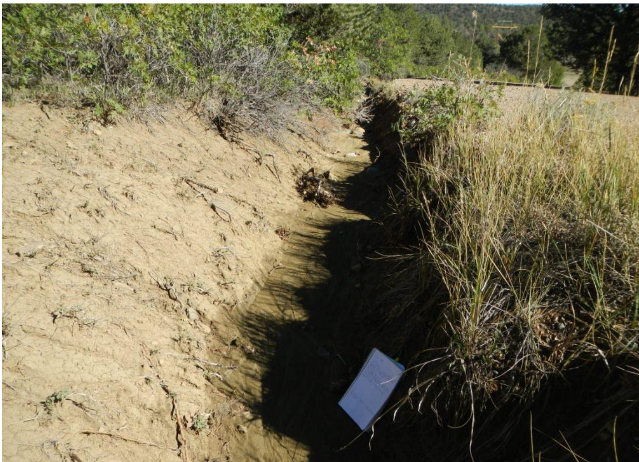
Photo 9. View of roadside ditch/water diversion channel on the eastern side of the access road that is approximately 3 to 4 feet wide and 3 to 4 feet deep.
