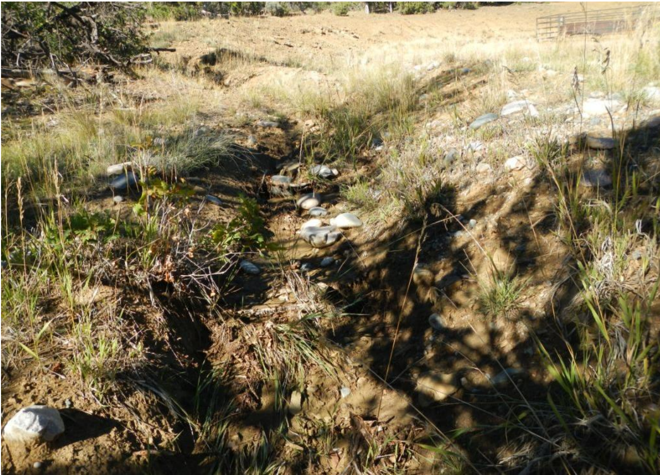
Photo 4. View of water diversion channel on the western edge of the well pad. Storm water flows appear to move rapidly through this area and carrying sediment off of the location.
