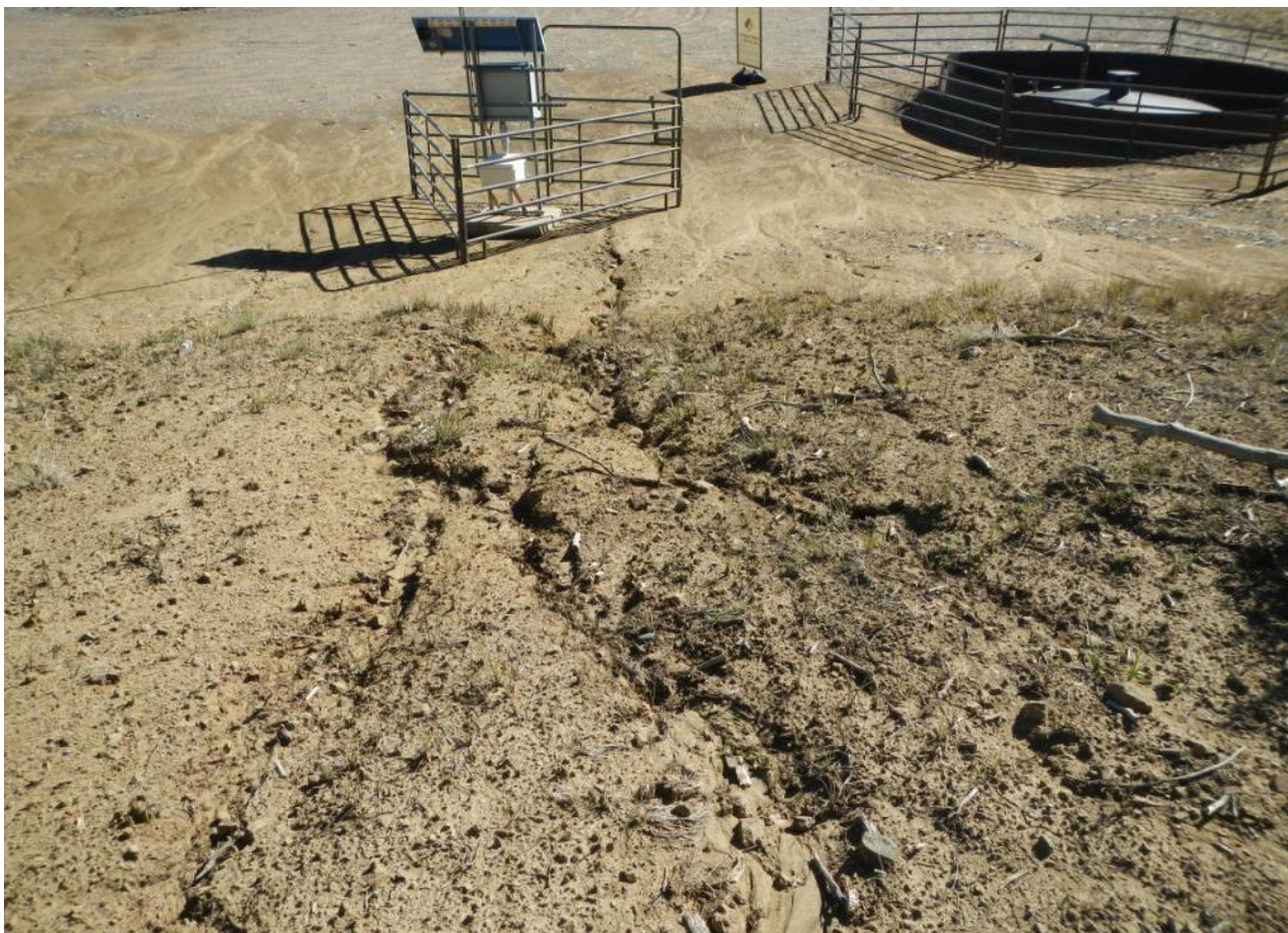
Photo 6. View of rill erosion on the cut-slope in the northern portion of the interim reclamation area and sediment run-on to the well pad from the cut-slope.
