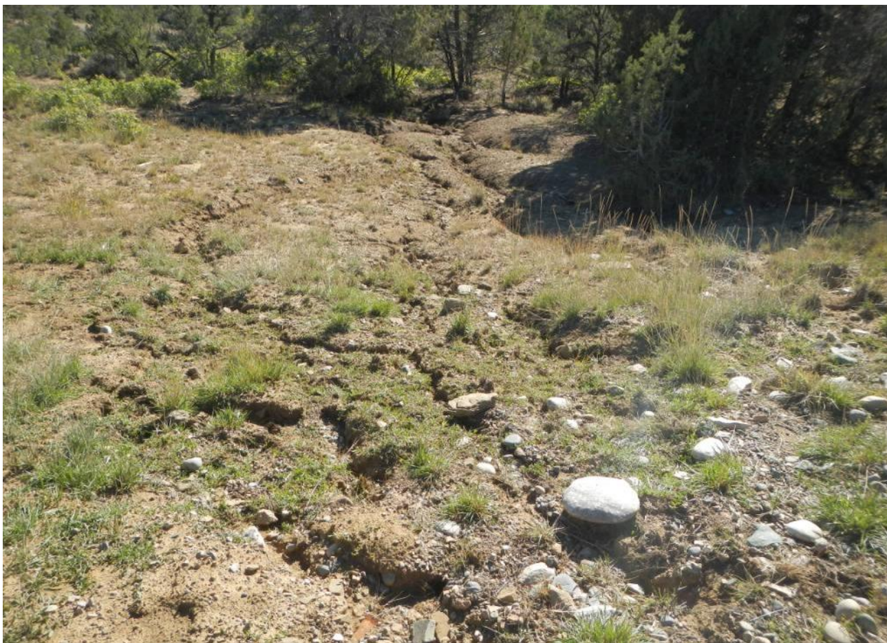
Photo 2. View of deep rills within the southern portion of the interim reclamation area eroding offsite.
