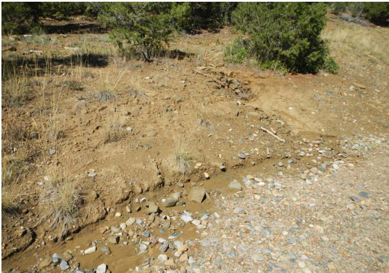
Photo 7. View of head-cut where water from stormwater diversion channel is eroding slope and meets up with access road.
