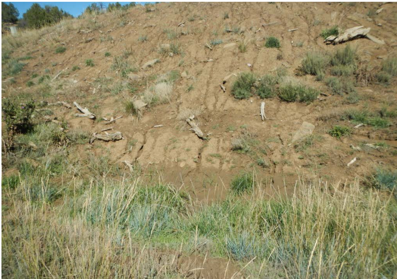
Photo 5. View of rill erosion on the fill slopes within the interim reclamation area.
