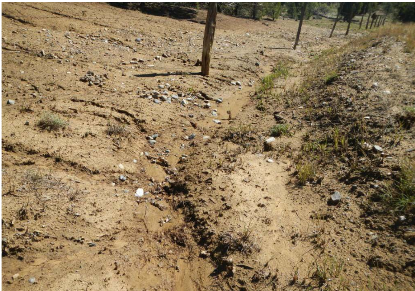
Photo 6. View of water diversion channel directing stormwater flows off of the northern edge of the well pad.
