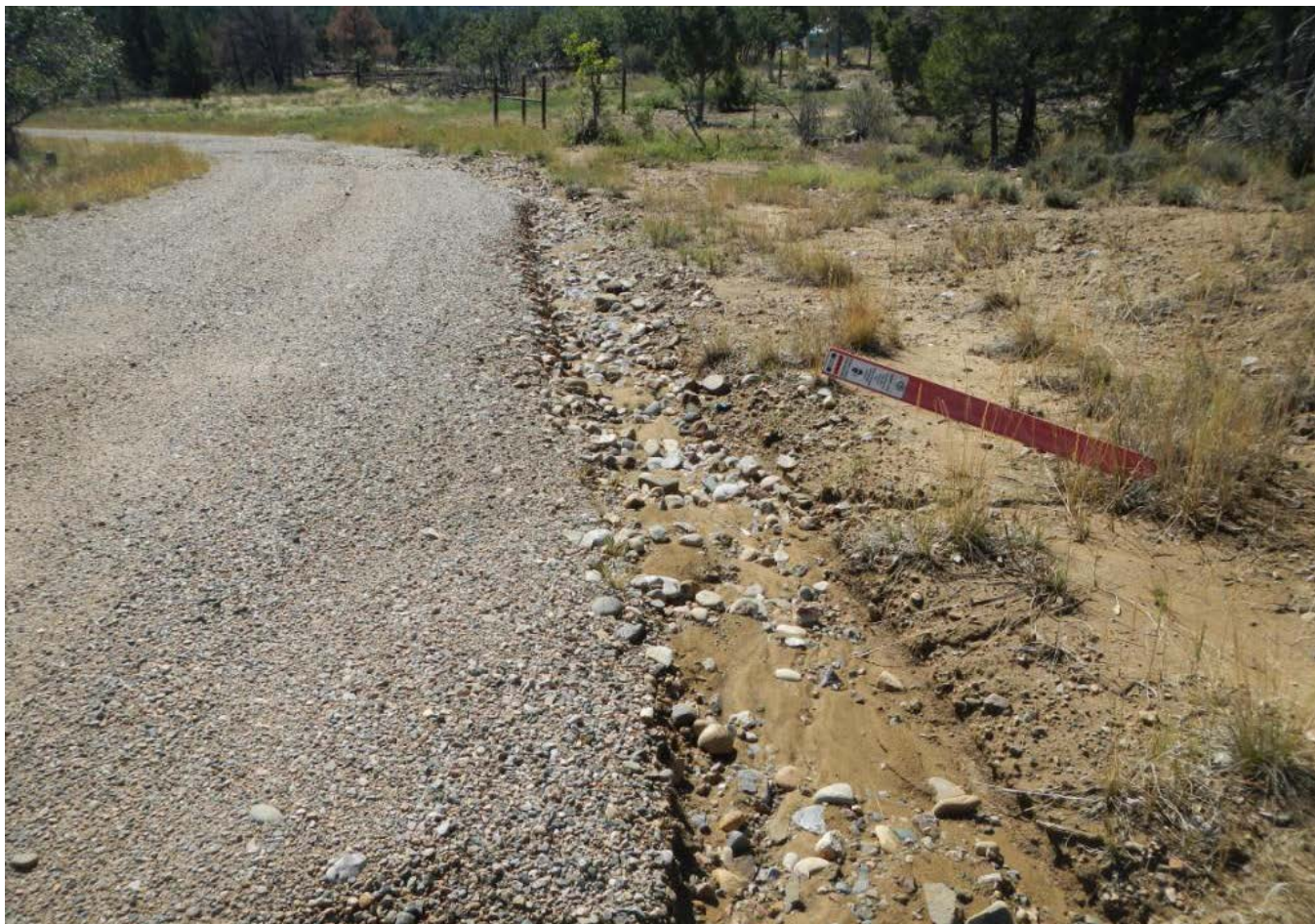
Photo 8. View of erosion along the access road that needs BMPs to de-energize and filter stormwater flows.
