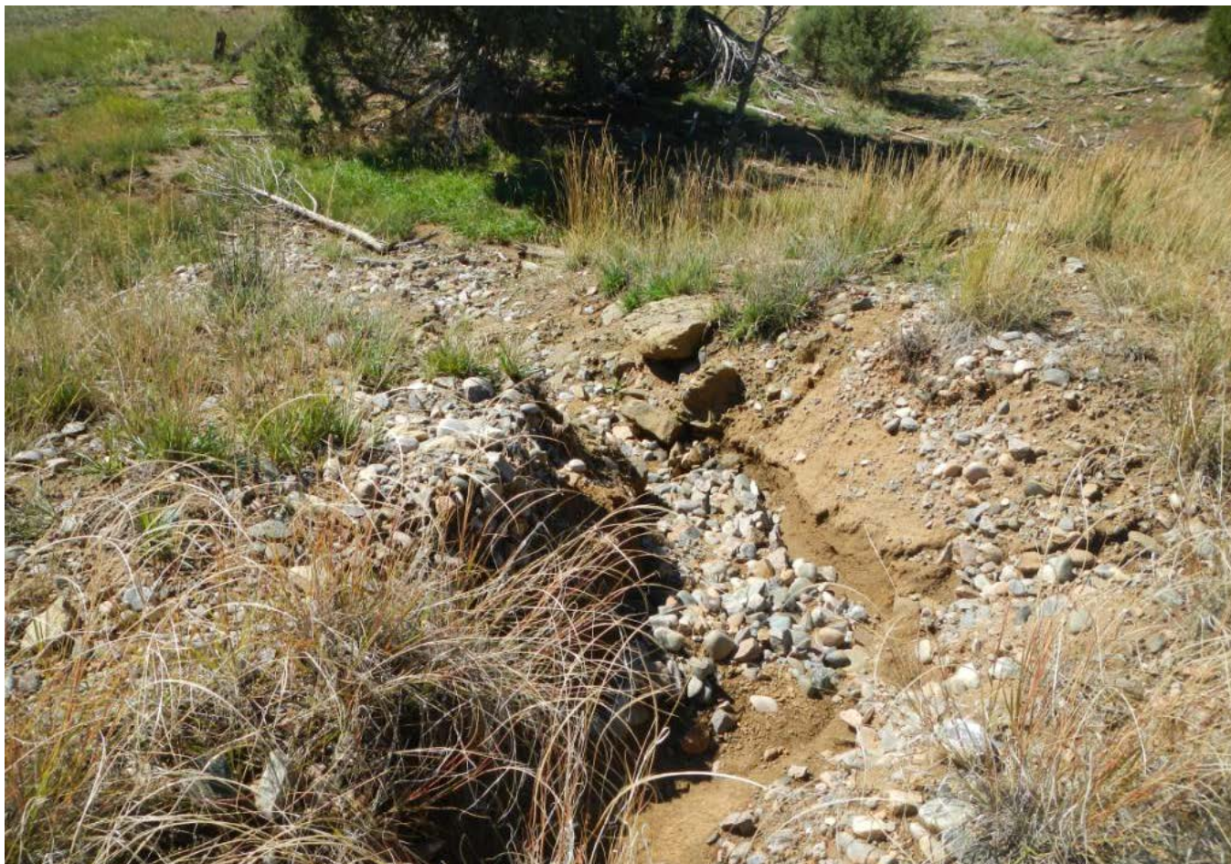
Photo 3. View of gully that is approximately 3 to 4 feet wide by 3 to 4 feet deep within eastern portion of the interim reclamation area.
