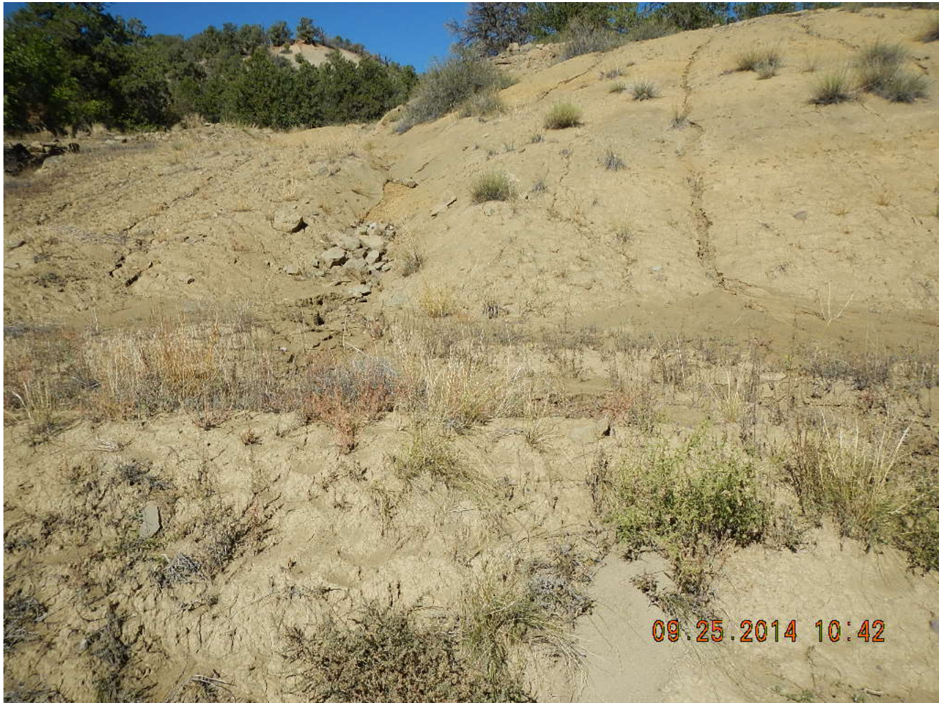
Photo 7. View of gully erosion (approximately 2 to 3 feet wide and 6 to 15 inches deep) occurring on the western edge of the well pad area.
