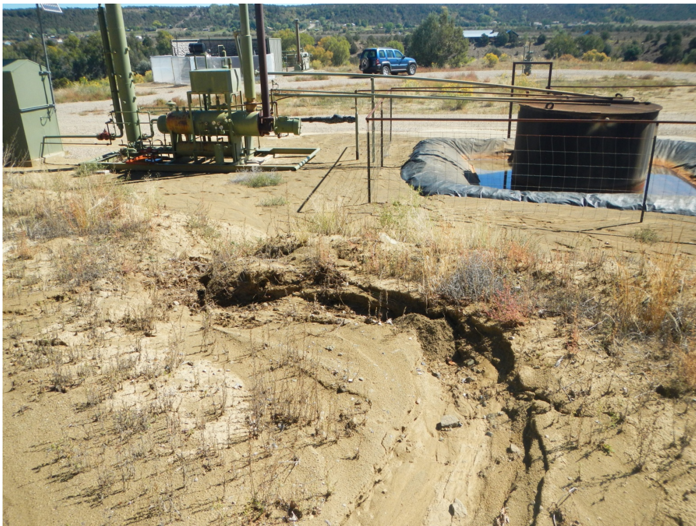
Photo 8. View of failed water diversion berm and sediment deposited on the well pad downstream of the erosional gully shown in Photo 7.
