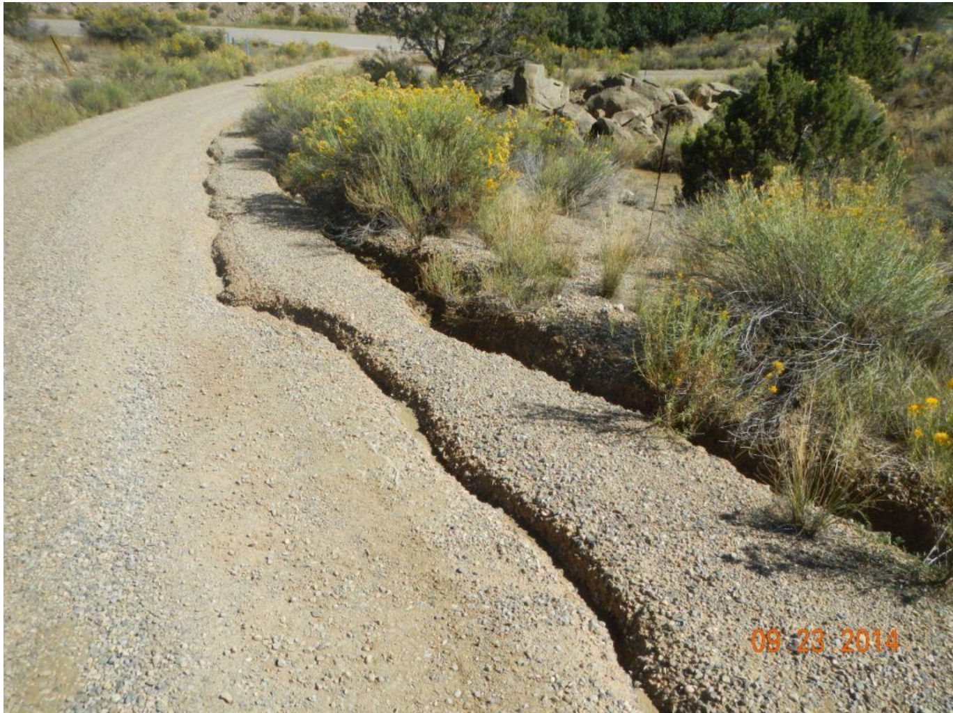
Photo 11. View of erosion on the southern edge of the access road.
