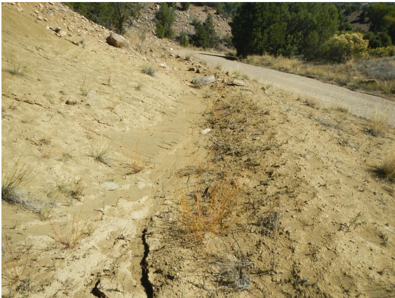
Photo 10. View of water diversion berm on western edge of well pad full of sediment and directing stormwater flows toward the access road.
