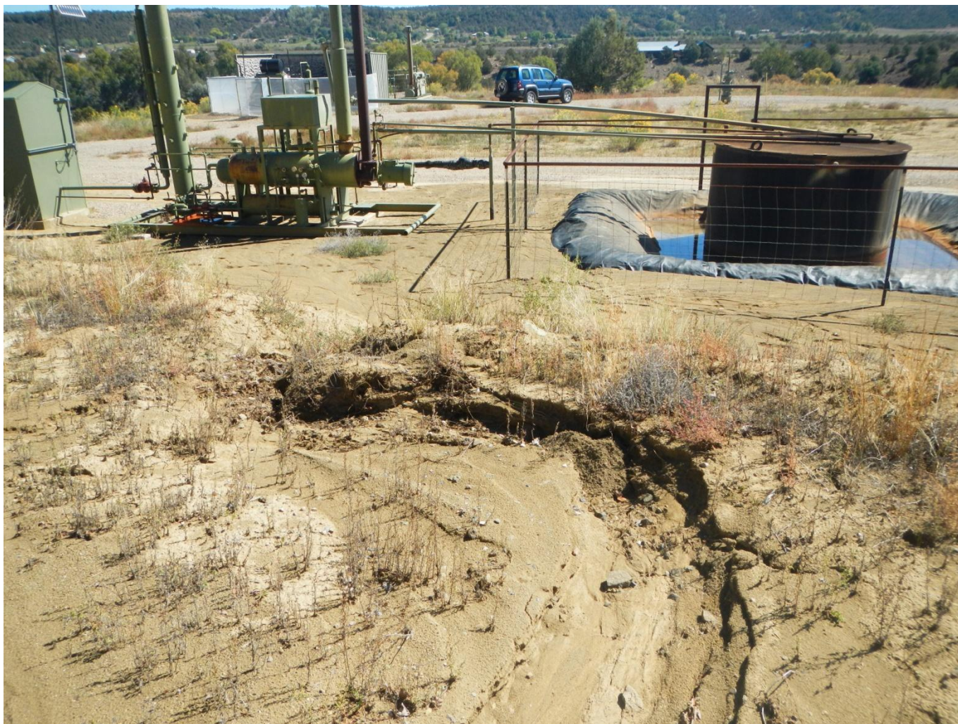
Photo 8. View of failed water diversion berm and sediment deposited on the well pad at the toe of the slope along the western edge of the well pad.
