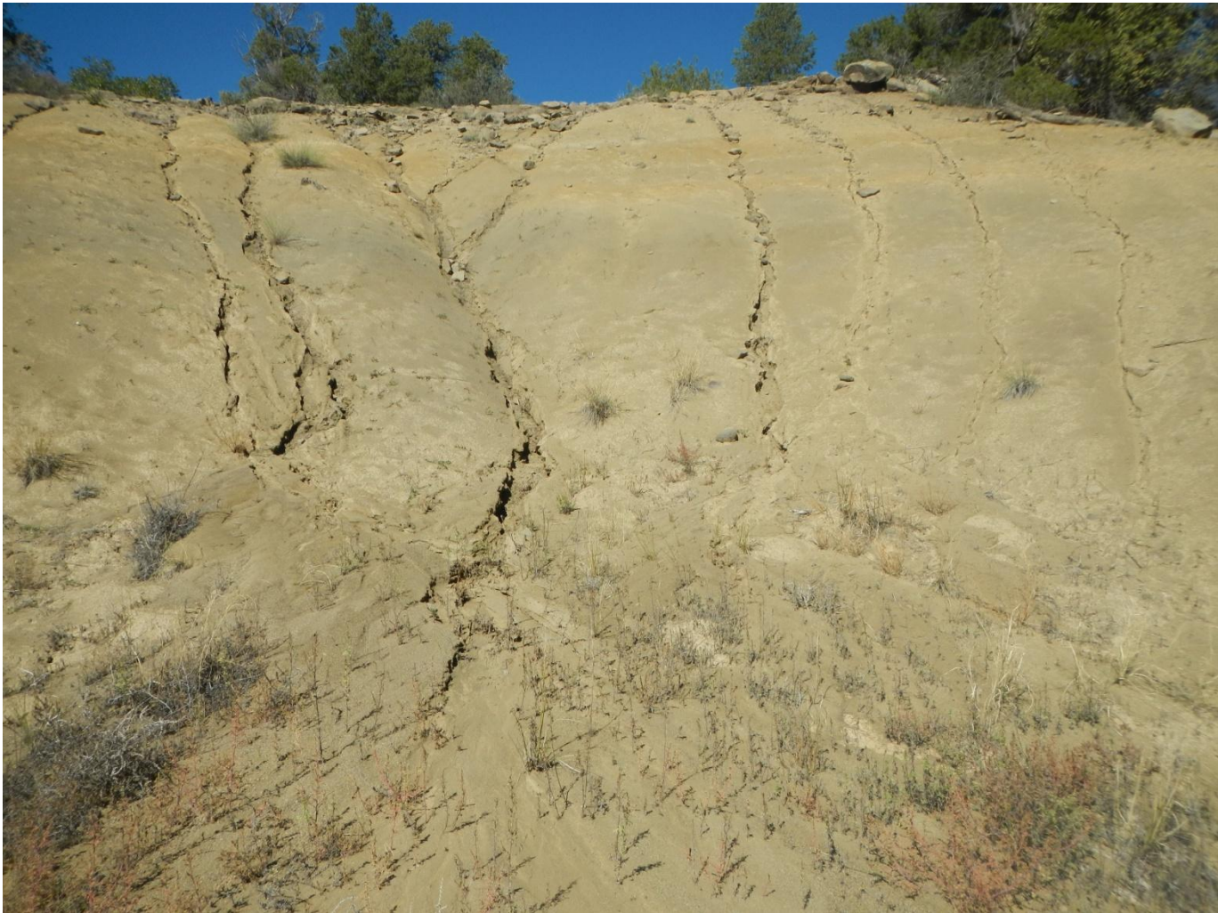
Photo 6. View of the slope above the eastern side of the well pad where rill erosion and sediment deposition is occurring.
