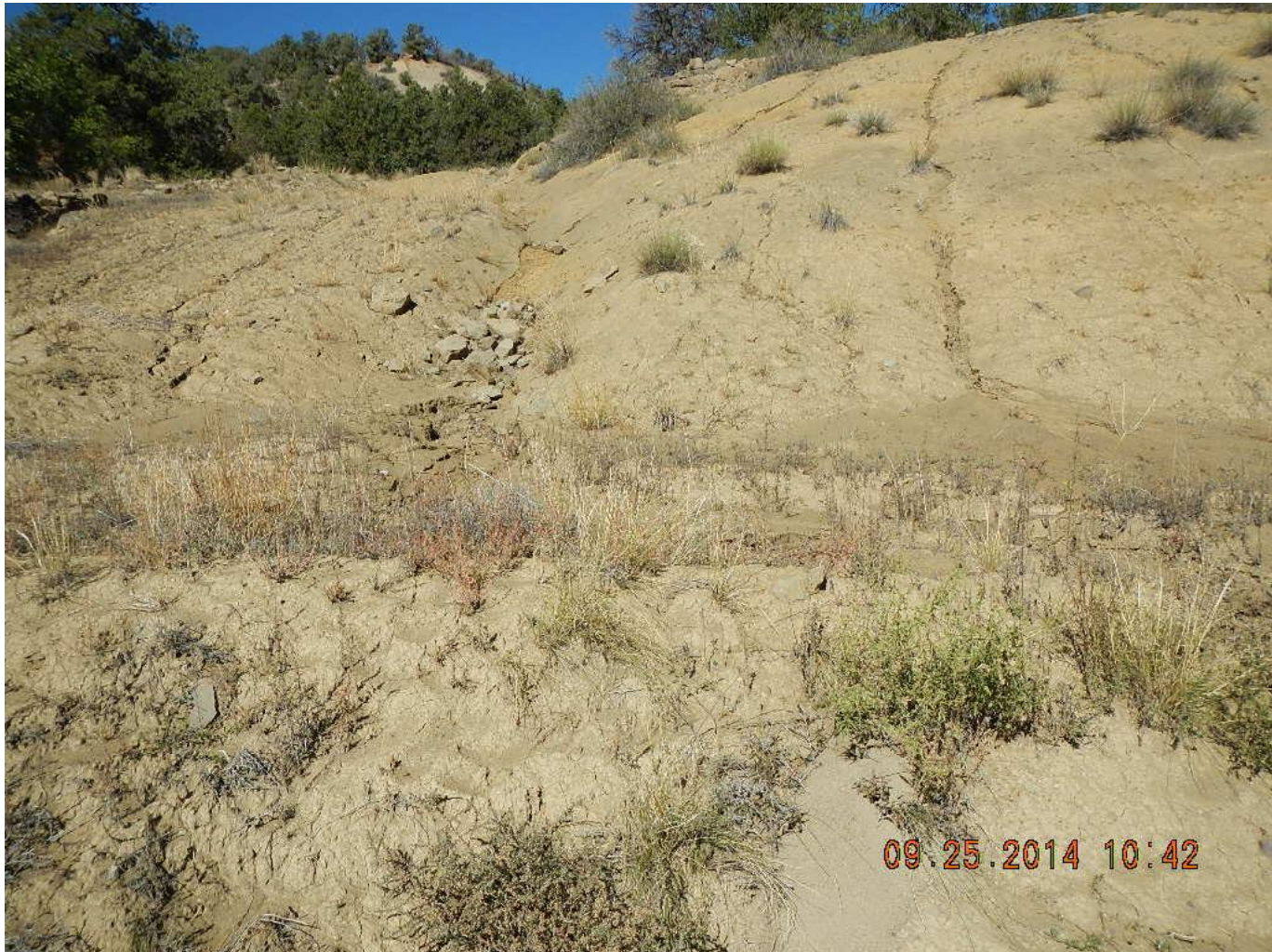
Photo 7. View of gully erosion occurring on the western edge of the well pad area.
