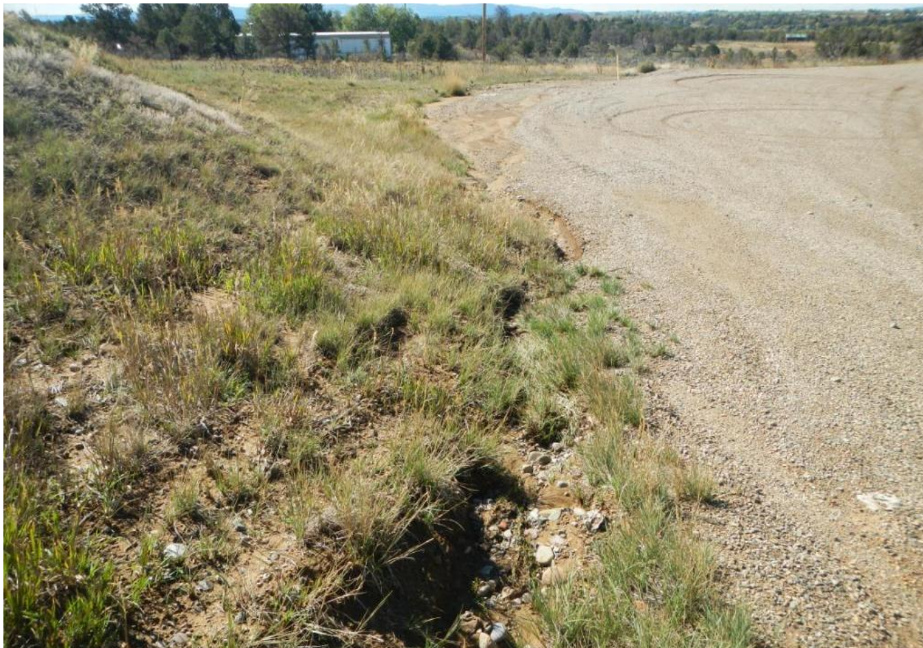
Photo 4. View of erosional channel eroding the eastern edge of the access road and depositing sediment on the well pad.
