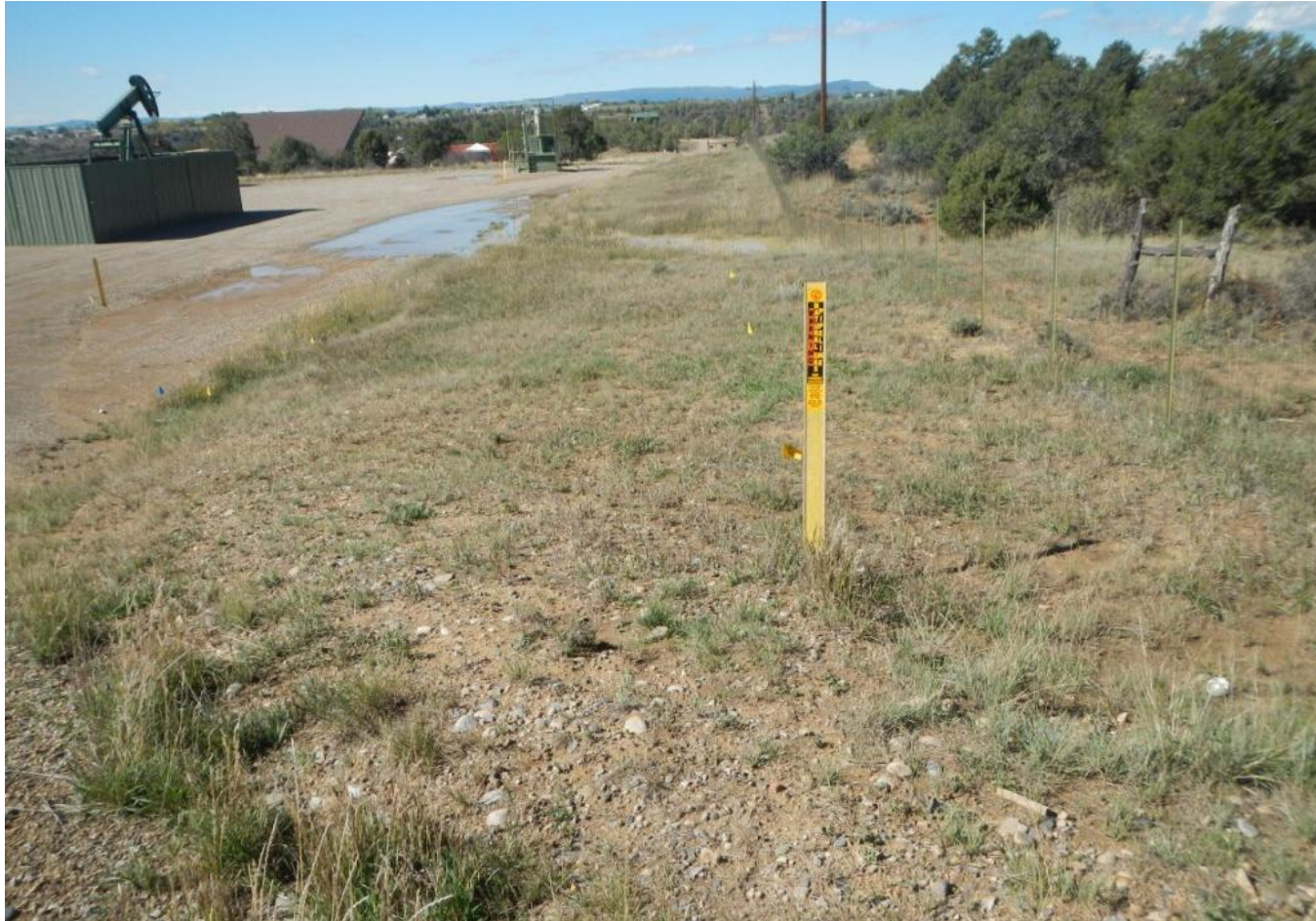
Photo 6. View of western portion of interim reclamation area with silt trap full of water and ponding on the well pad that does not appear to be on the driving surface and does not appear to be overflowing off of the well pad.
