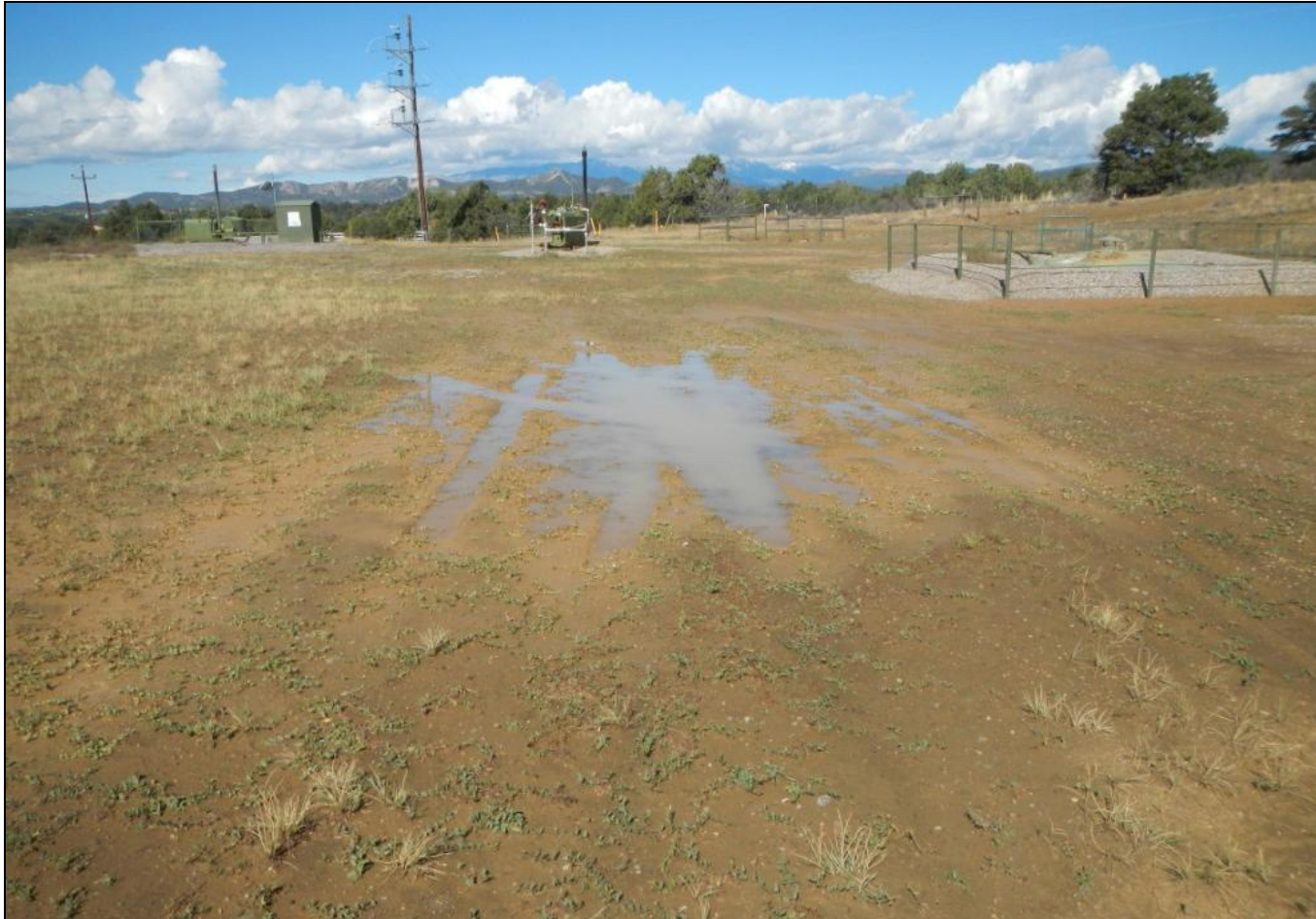
Photo 8. View of water ponding on the driving surface of the well pad.
