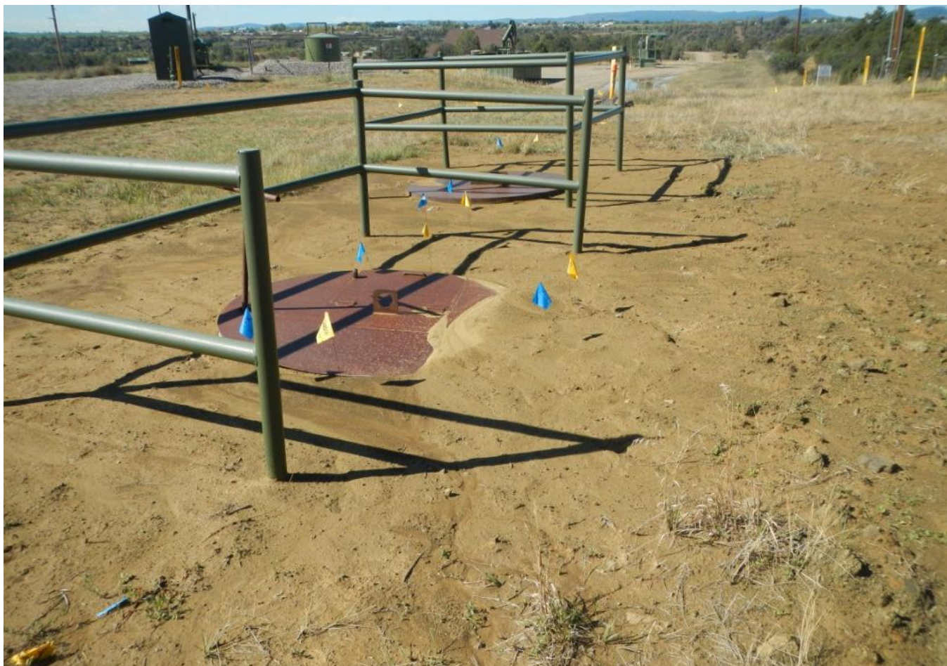
Photo 5. View of sediment deposition on well pad and facilities from unstabilized cut-slope on northern edge of the well pad.
