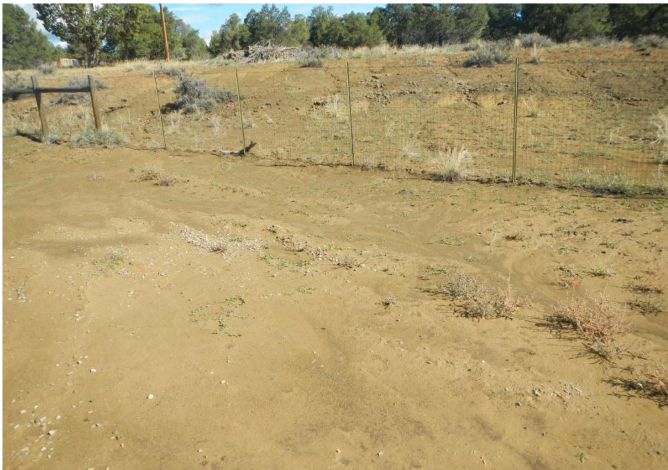
Photo 7. View of sediment deposition on the well pad downstream of the cut-slope on the northern edge of the well pad.
