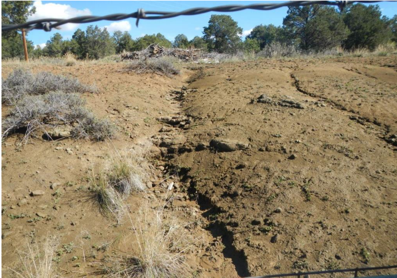
Photo 6. View of erosional channels on the cut-slope on the northern edge of the project area.
