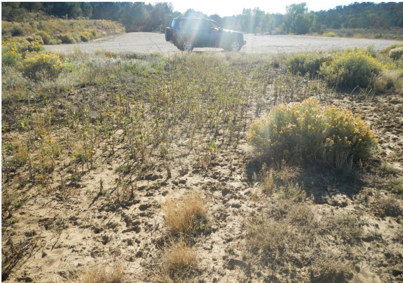
Photo 1. View of silt trap largely full of sediment within the northern portion of the interim reclamation area.
