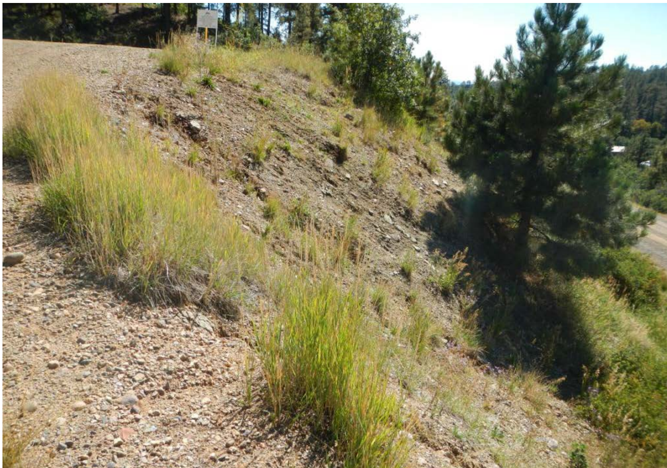
Photo 1. View of fill slope with some rill erosion occurring on the western edge of the well pad from the access road facing southward.
