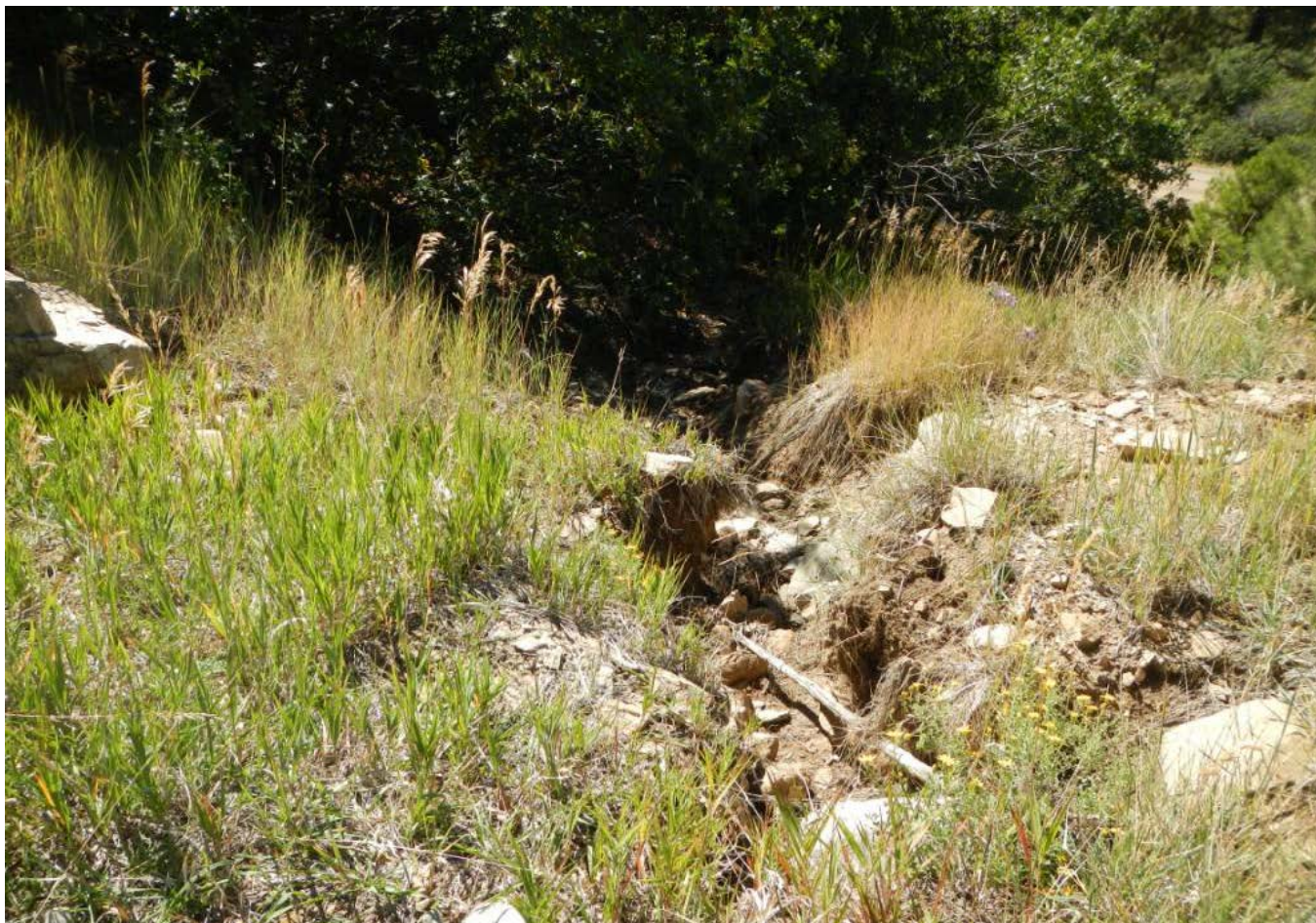
Photo 2. Gully that is approximately 2 to 3 feet wide and 1 to 1.5 feet deep eroding the fill slope in southwestern corner of the well pad.
