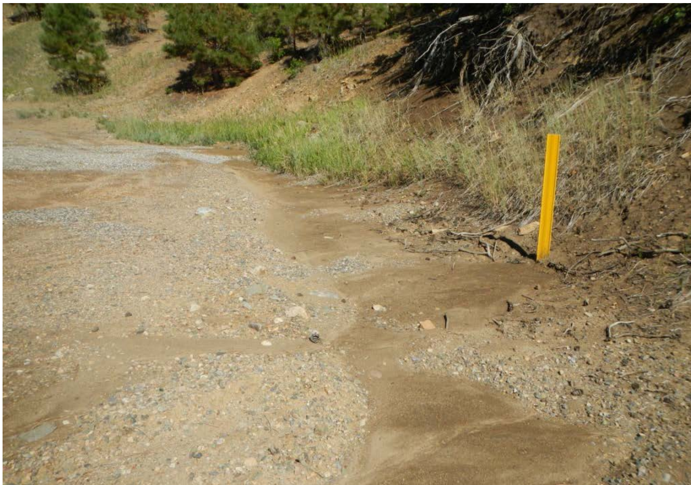
Photo 4. View of sediment deposition on the well pad from the cut slopes along the eastern edge of the well pad.
