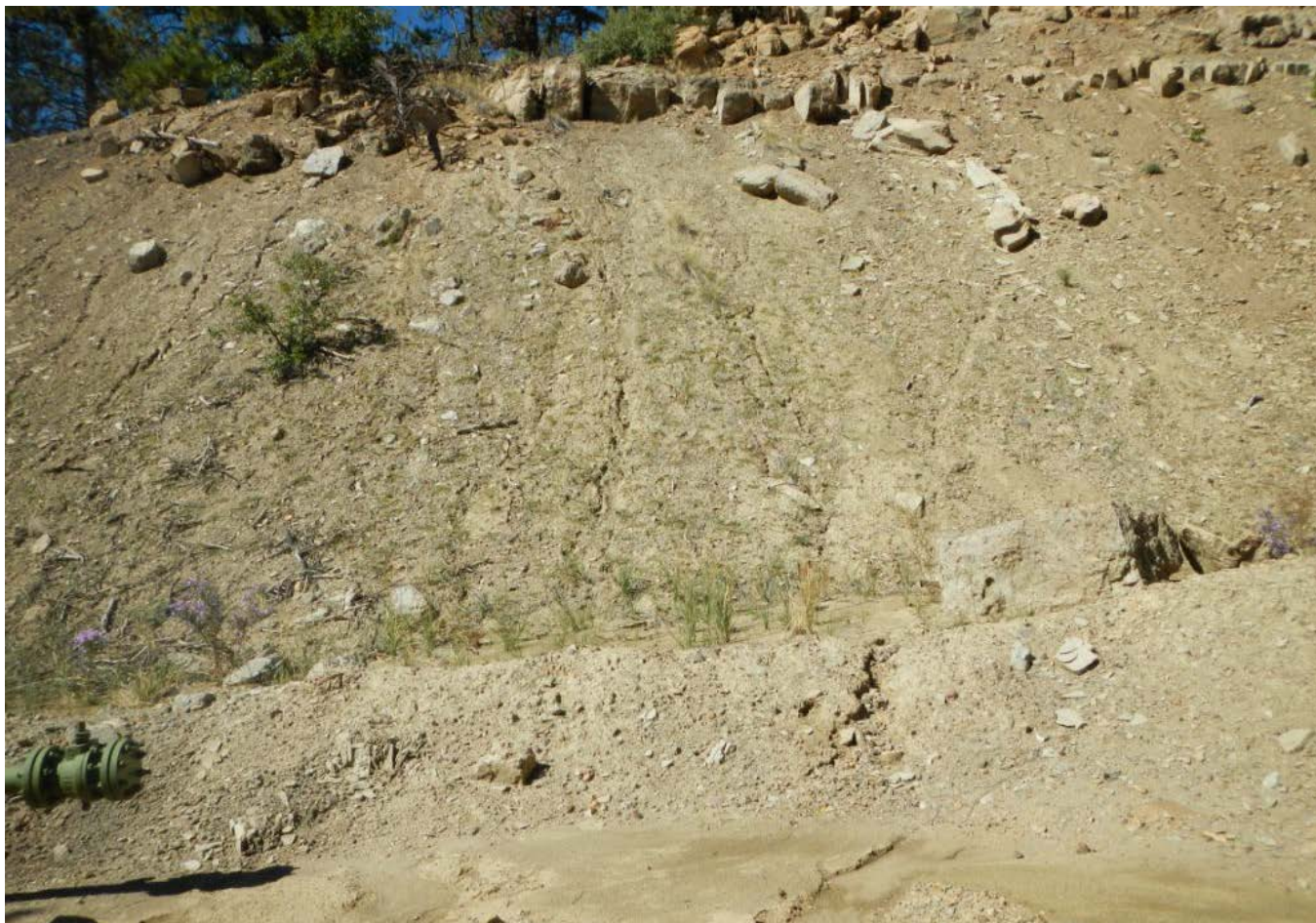
Photo 6. View of rill erosion in the cut slope on the northern edge of the well pad.
