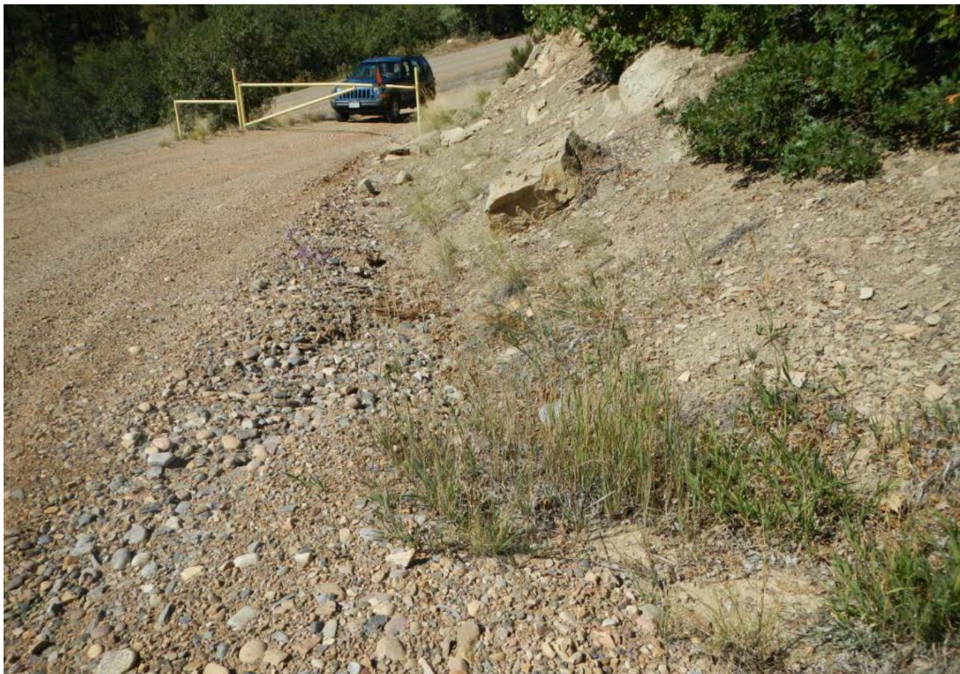
Photo 7. View of erosion along the access road from the well pad facing downhill and westward.
