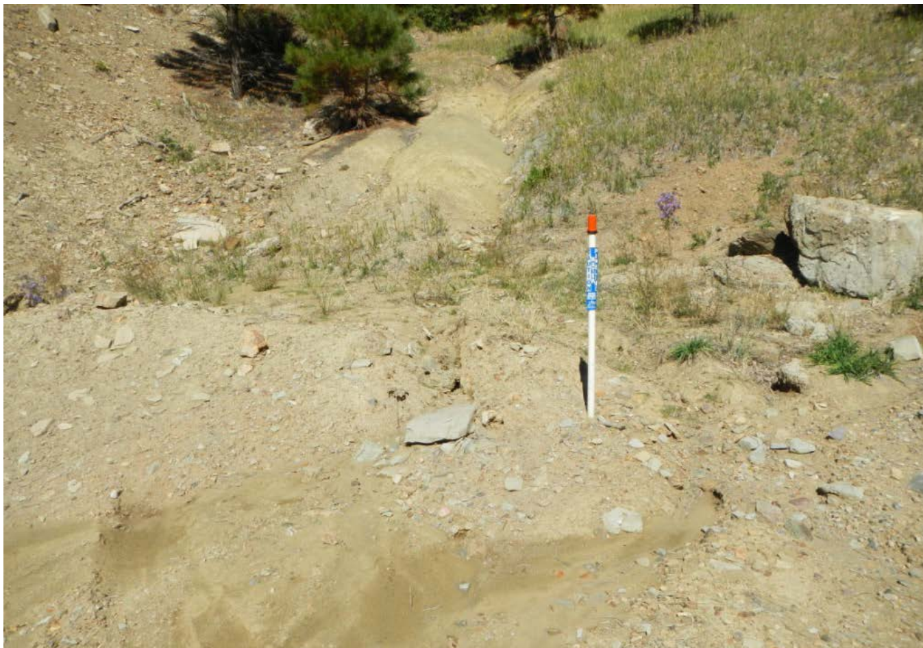
Photo 5. View of gully in northeastern corner of well pad that has eroded through a diversion berm and is eroding sediment onto the well pad.
