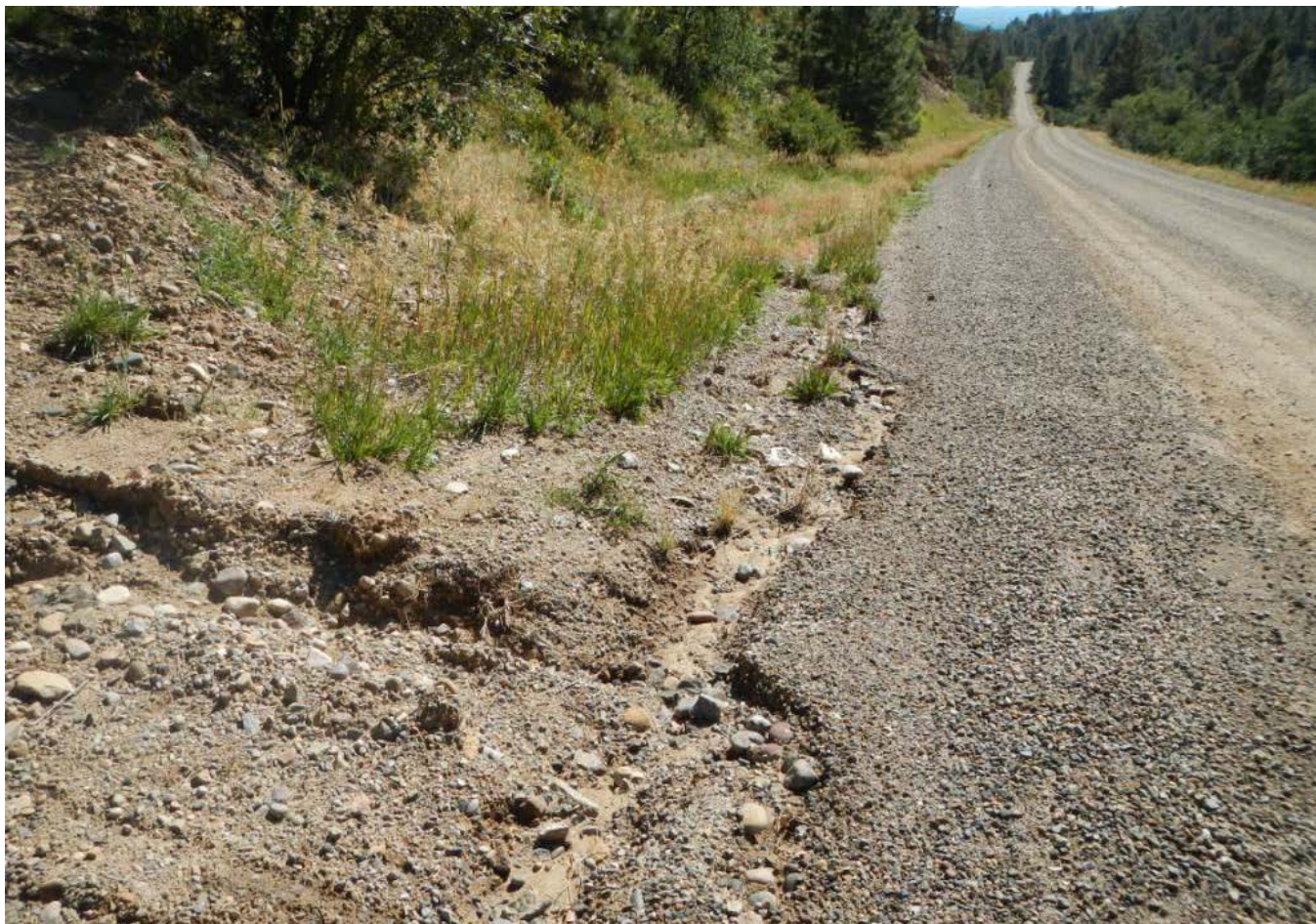
Photo 8. View of erosion along Road 502 and downstream from the entrance to the access road that appears to be caused from stormwater exiting the well pad.
